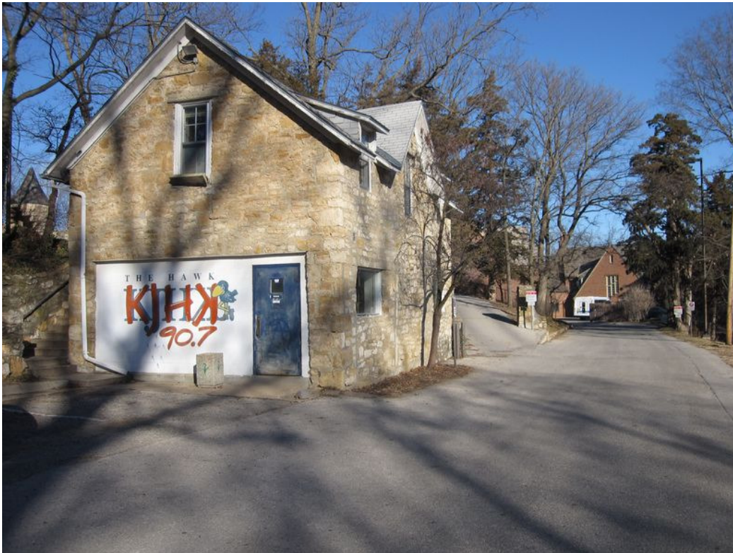
Figure 8 (below): Lane-Duncan Stable / 1132 W 11 th Street, Lawrence, Douglas County Front, east-facing elevation, photo taken 1-8-2011. Note: Central 2 nd -story window opening has been shortened
