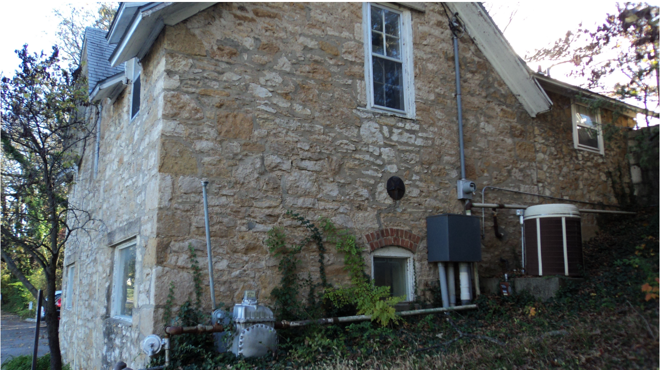
Figure 10: Lane-Duncan Stable / 1132 W 11 th Street, Lawrence, Douglas County Side, north-facing elevation, photo taken October 27, 2010
