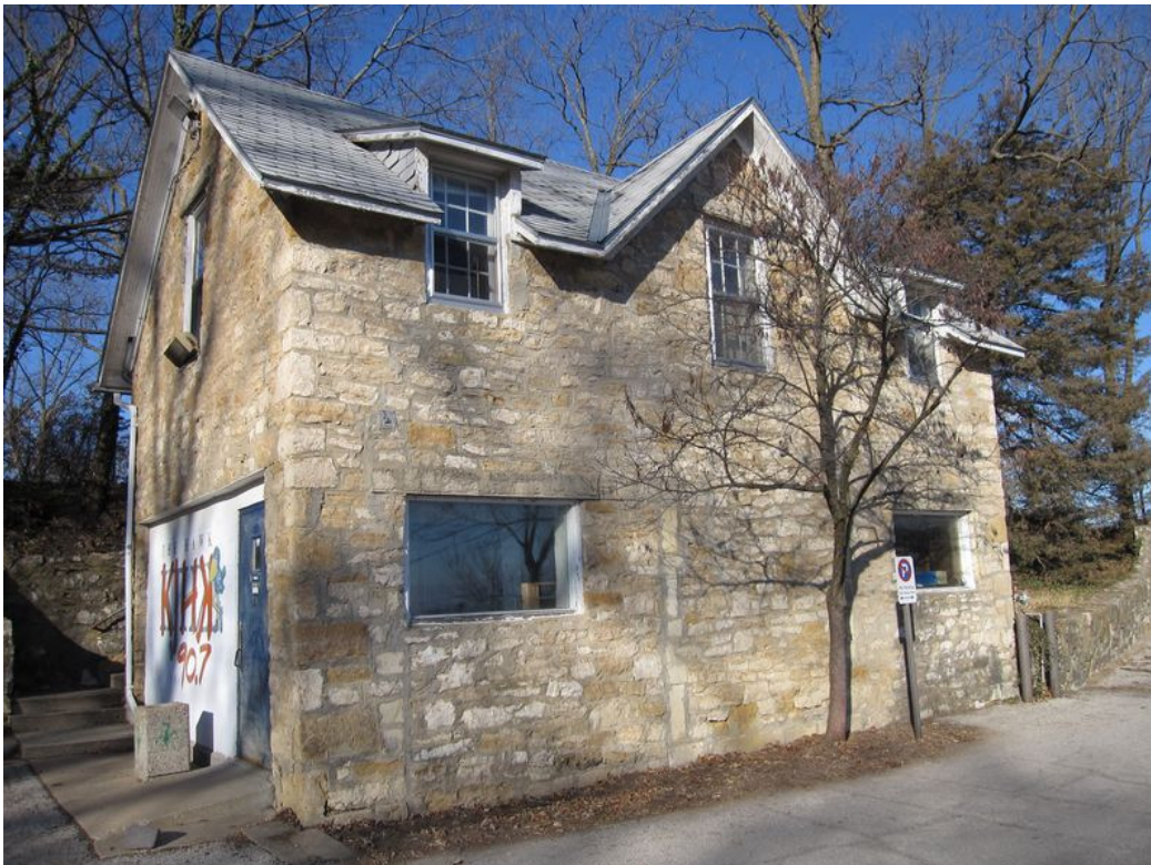
Figure 8 (below): Lane-Duncan Stable / 1132 W 11 th Street, Lawrence, Douglas County Front, east-facing elevation, photo taken 1-8-2011. Note: Central 2 nd -story window opening has been shortened
