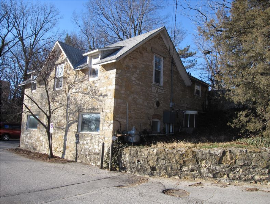
Figure 9 (below): Lane-Duncan Stable / 1132 W 11 th Street, Lawrence, Douglas County East (front) and north (side) elevations, photo taken 1-8-2011.
