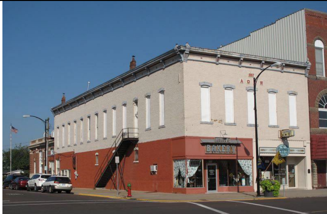
A.O.W.U. Building (1887) with opera house in the second floor. Loughlin, 2017, KHRI.
