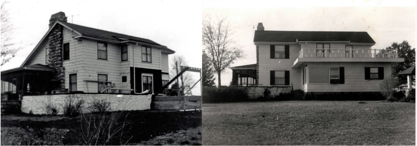
Figure 7. Early 1960s construction photos of northwest addition. (Karen Cloud Seaberg)
