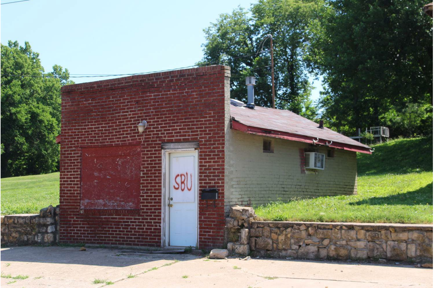
Photo 5 West (main) and south elevations of the Garage
