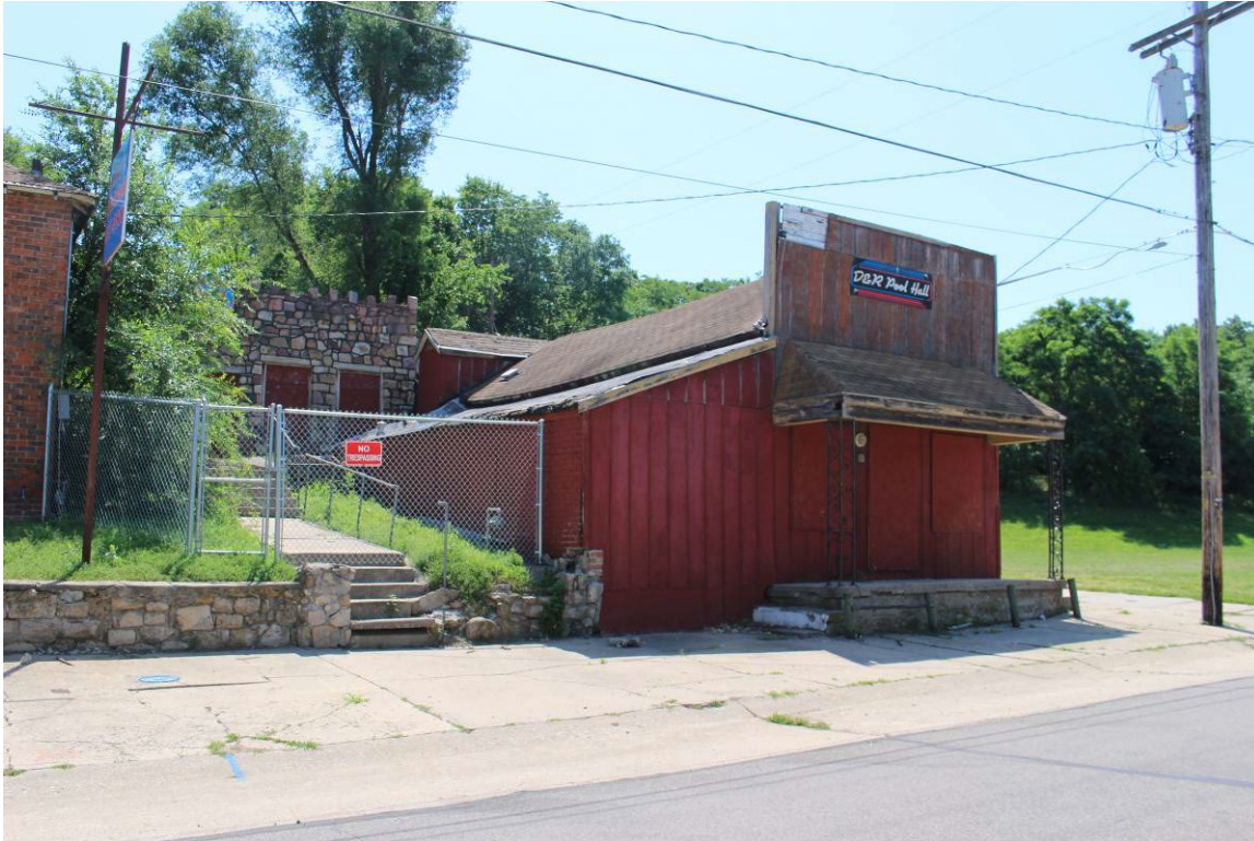
Figure 1: North and West (main) elevations of the Grocery building.
