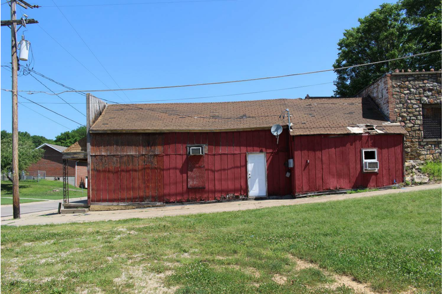
Photo 2 South elevation of the Grocery Building
