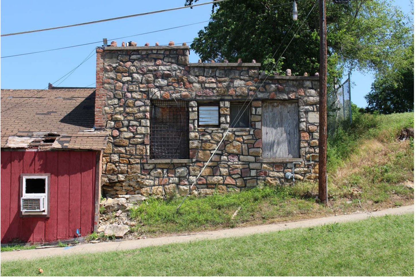
Photo 4 South elevation of the Rock-Inn
