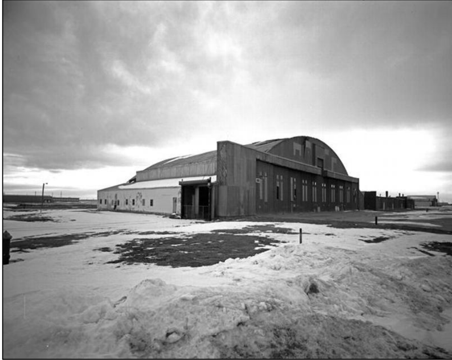
Figure 7. SW view of NW elevation (Historic American Engineering Record Inventory KS-09 photograph by Matthew Holtkamp.)
