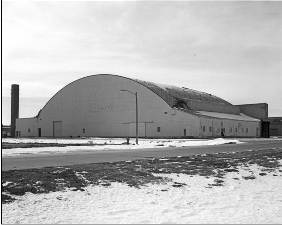
Figure 9. SW view of NE elevation (HAER KS-09 photograph by Matthew Holtkamp.)
