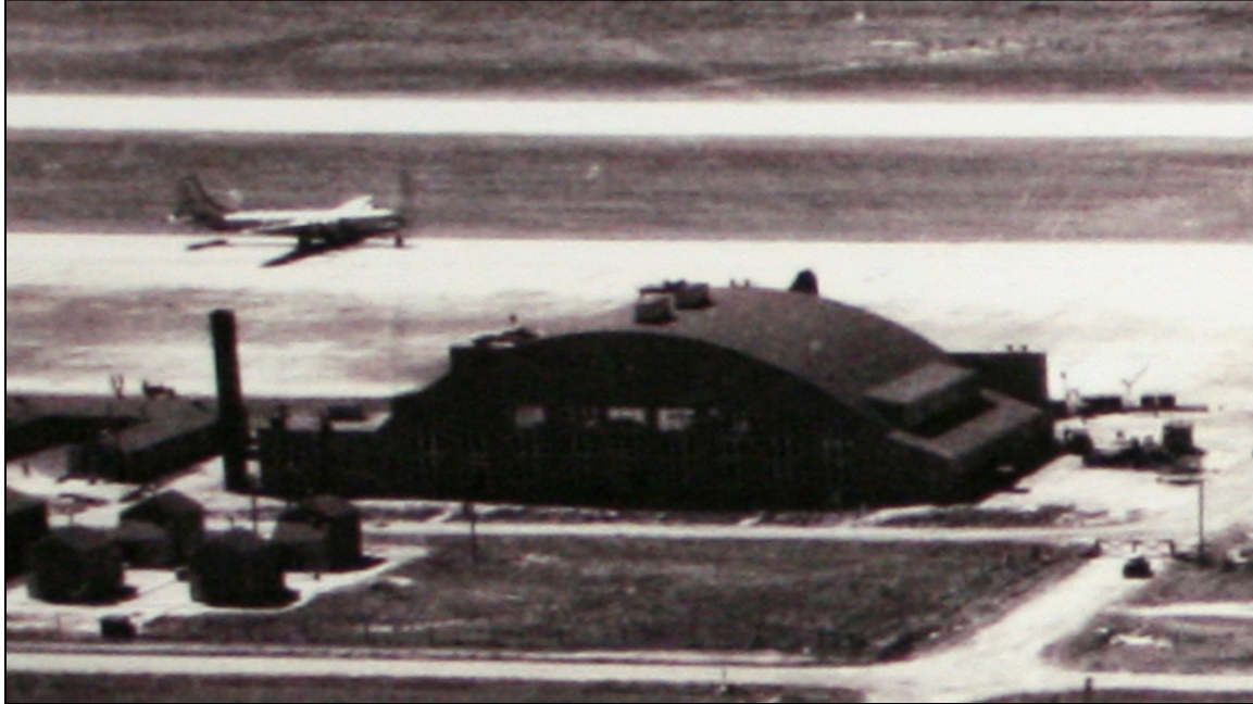
Figure 5. Undated photograph of the B-29 hangar during World War II. (Barton County Historical Society records.)
