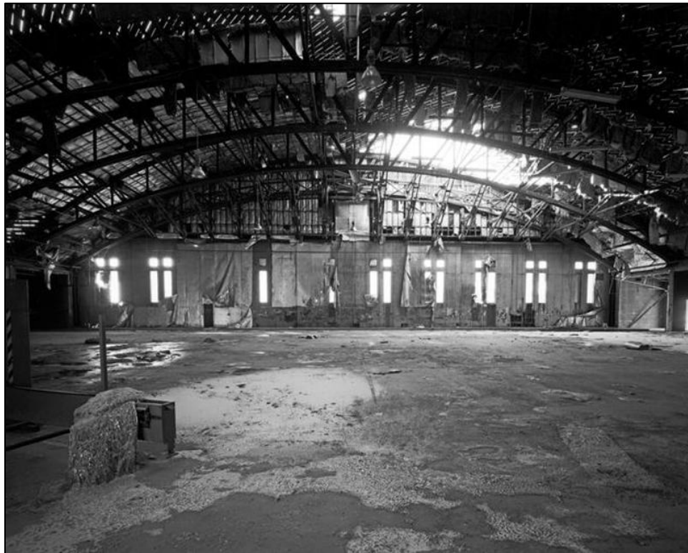
Figure 14. West view of interior (HAER KS-09 photograph by Matthew Holtkamp.)
