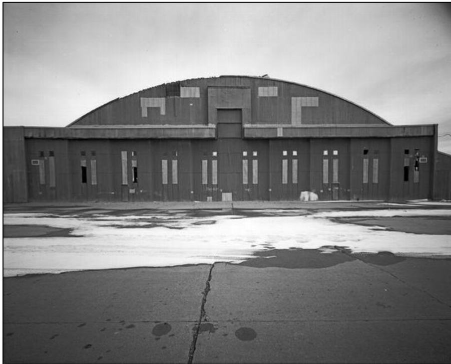
Figure 8. West elevation (HAER KS-09 photograph by Matthew Holtkamp.)
