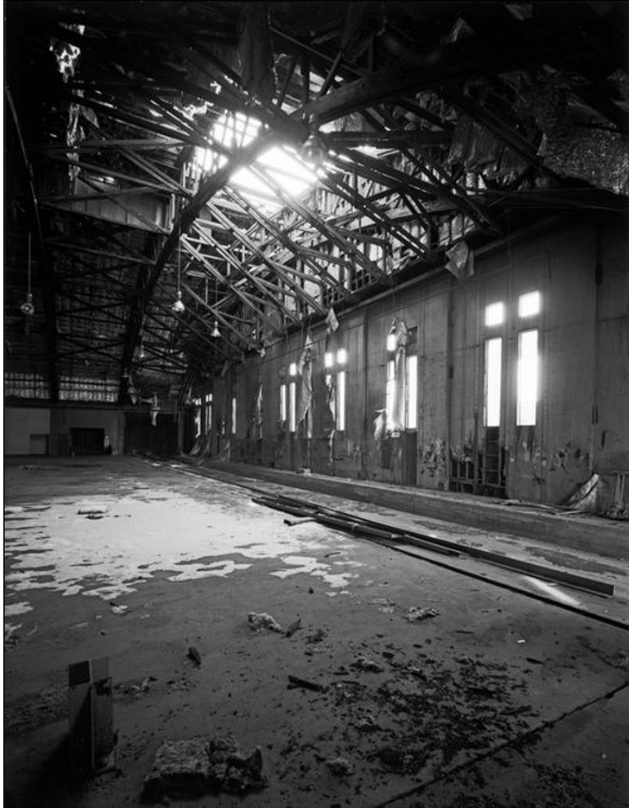
Figure 15. SW view of interior (HAER KS-09 photograph by Matthew Holtkamp.)
