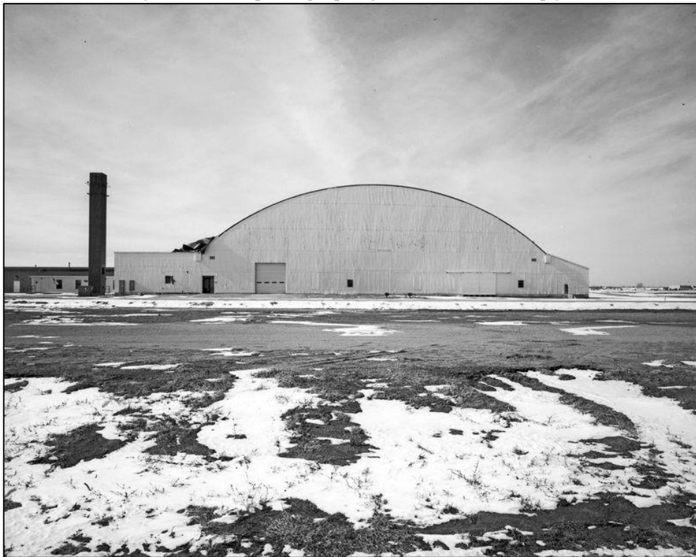
Figure 10. East elevation (HAER KS-09 photograph by Matthew Holtkamp.)
