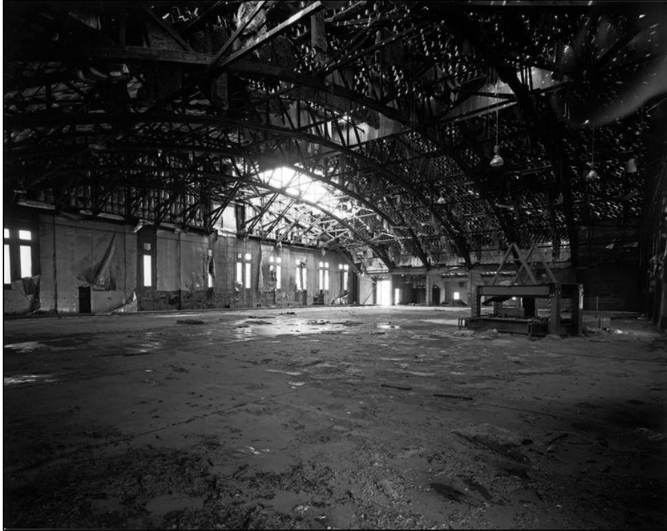
Figure 11. NW view of interior (HAER KS-09 photograph by Matthew Holtkamp.)
