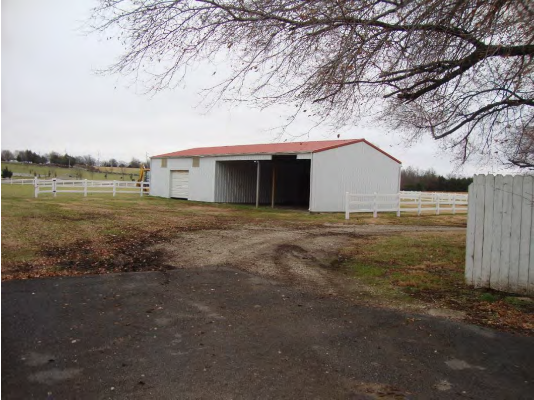
Photograph 6: 2000 utility pole barn, northeastern corner
