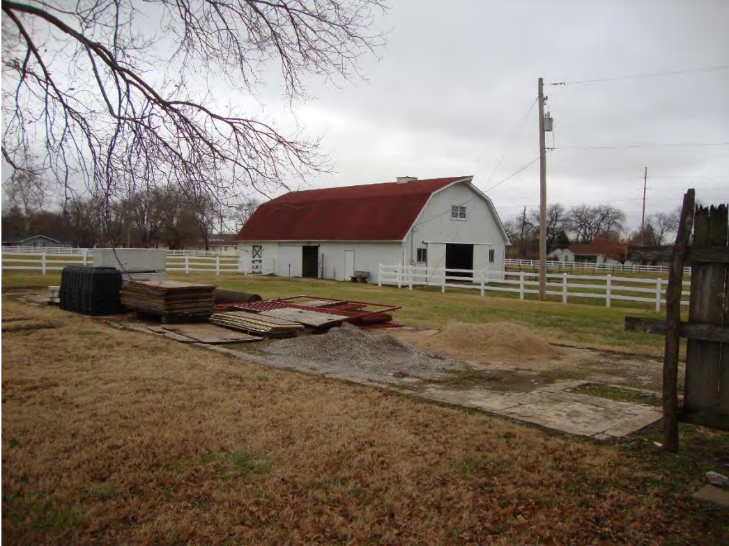
Photograph 5: 1990 horse barn (northeastern corner) with concrete slab in the foreground
