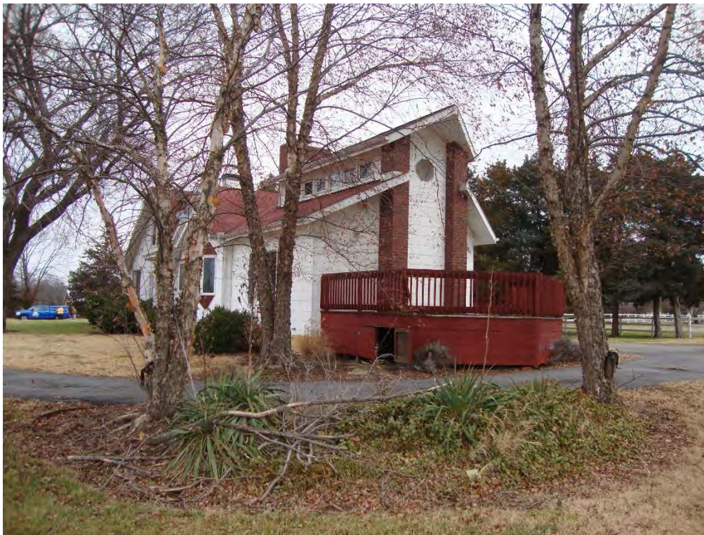
Photograph 2: 1935 farmhouse, 1996 rear addition with deck, southwestern corner
