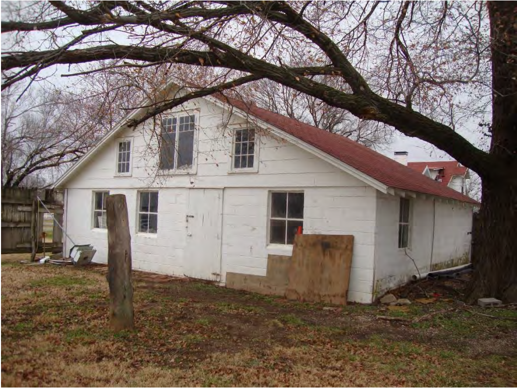
Photograph 4: 1950 garage, southeastern corner
