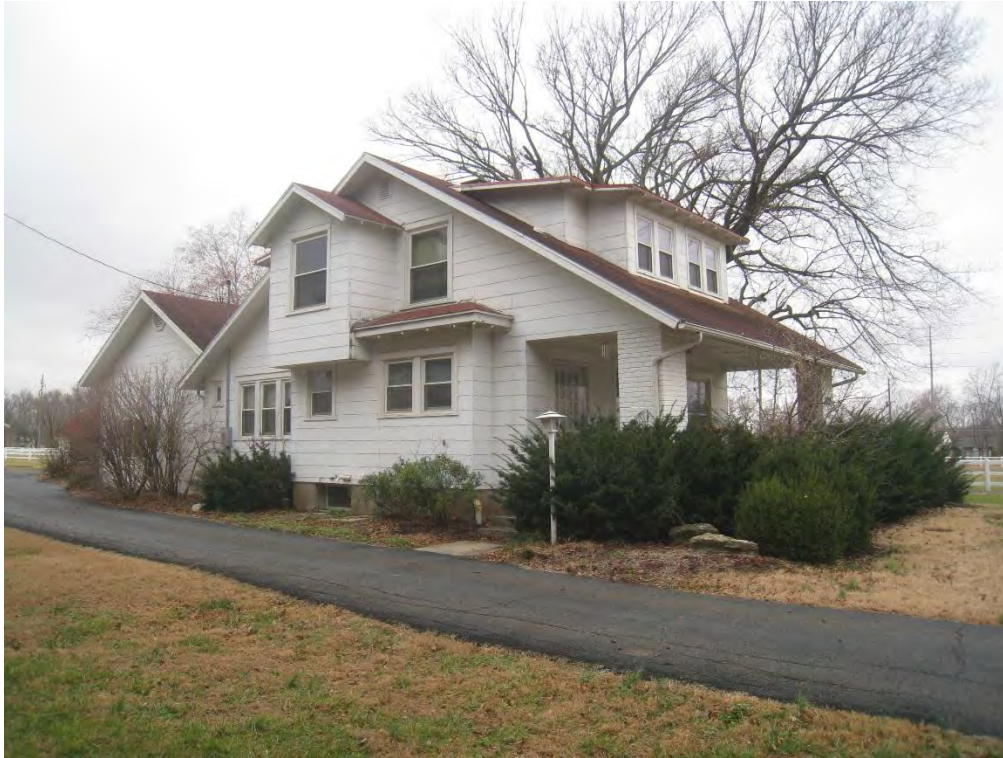
Photograph 1: 1935 bungalow-style farmhouse (rear addition visible on far left), northeastern corner
