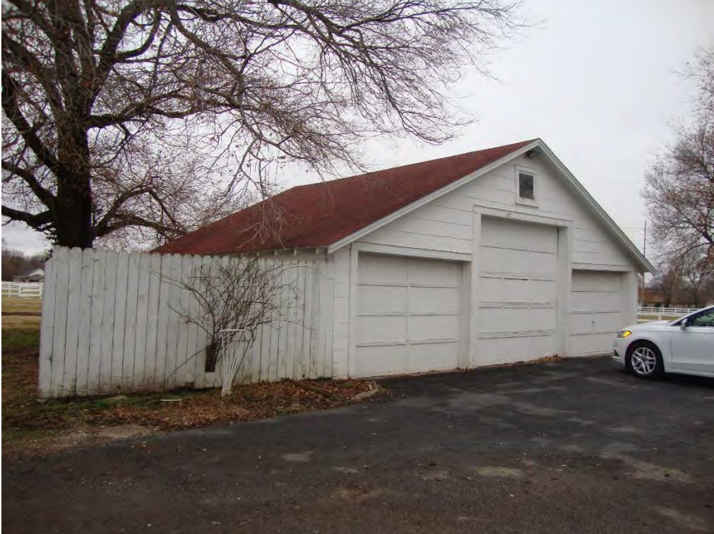
Photograph 3: 1950 garage, northeastern corner
