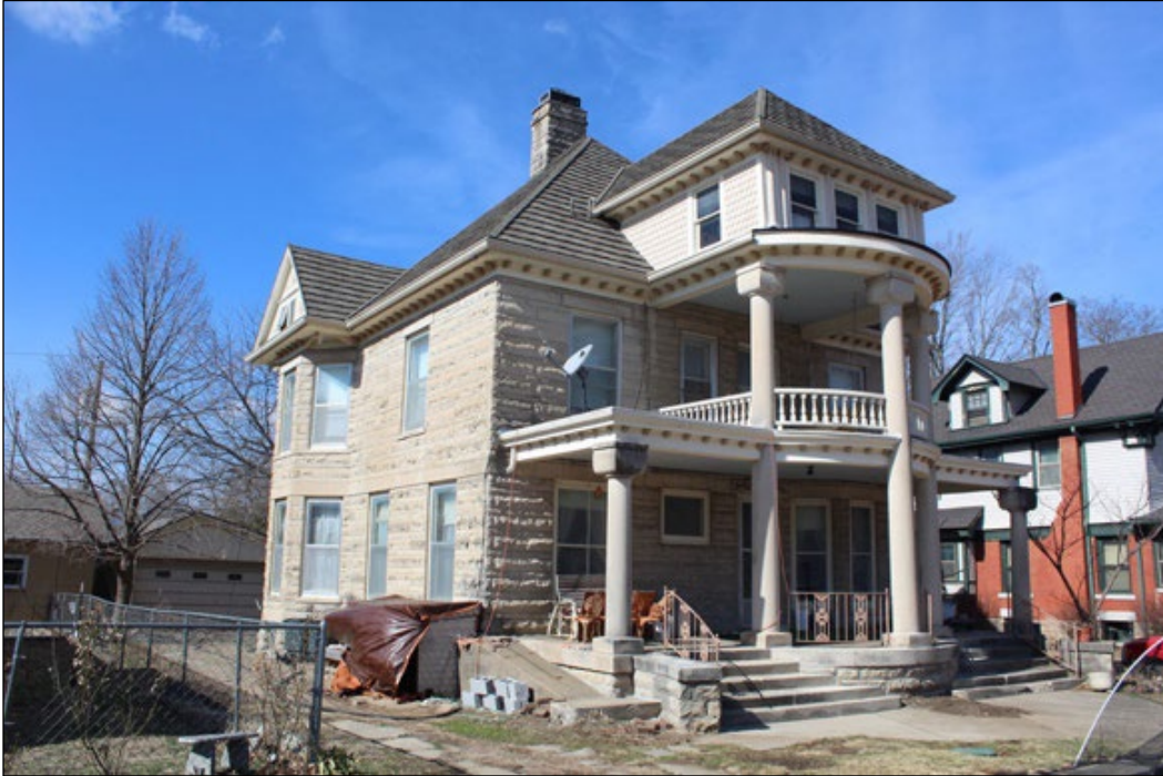
Photo 1 Southeast elevation. Camera pointing northwest.
