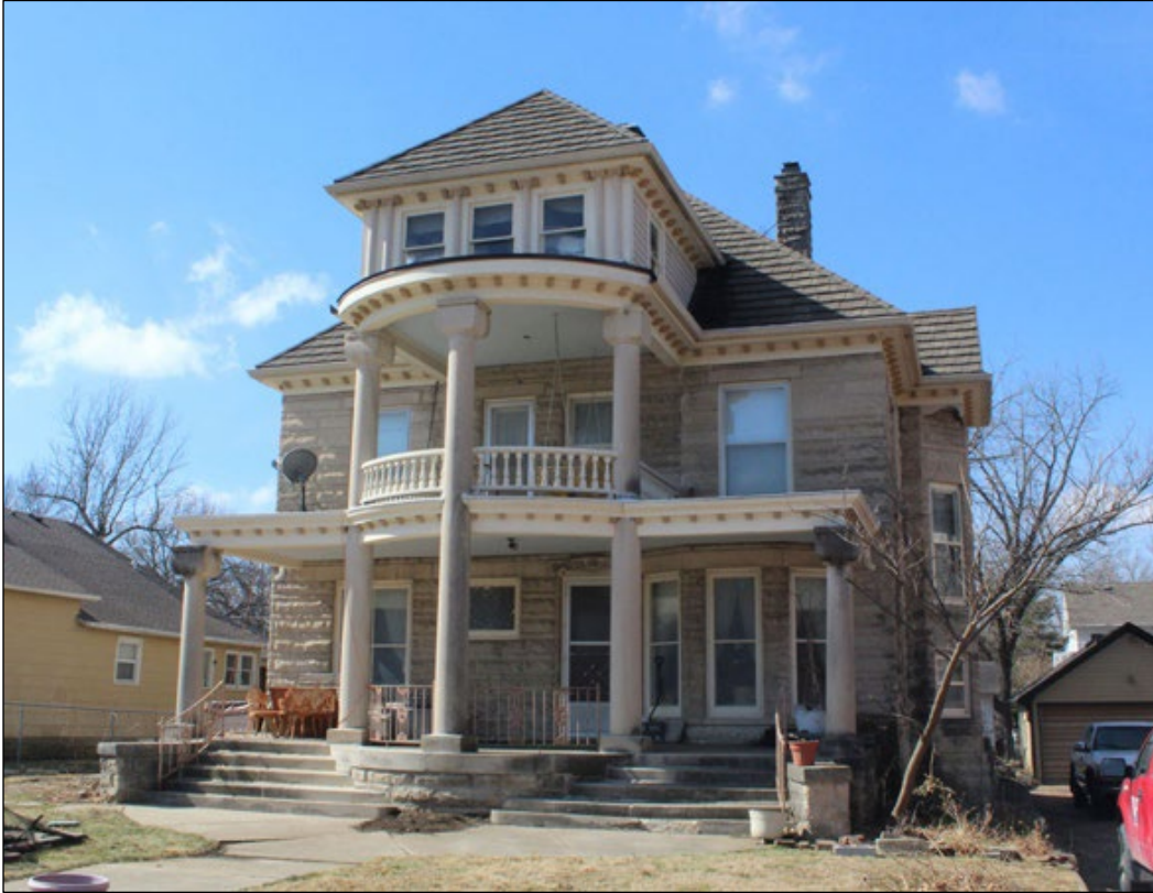
Photo 3. Northeast elevation. Camera pointing southwest.
