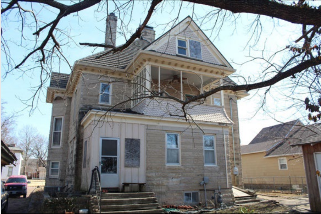
Photo 5. West elevation. Camera pointing southeast.
