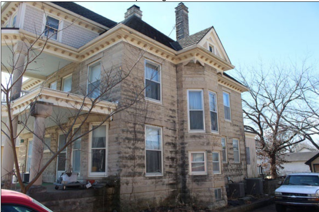
Photo 4. North elevation. Camera pointing southwest.
