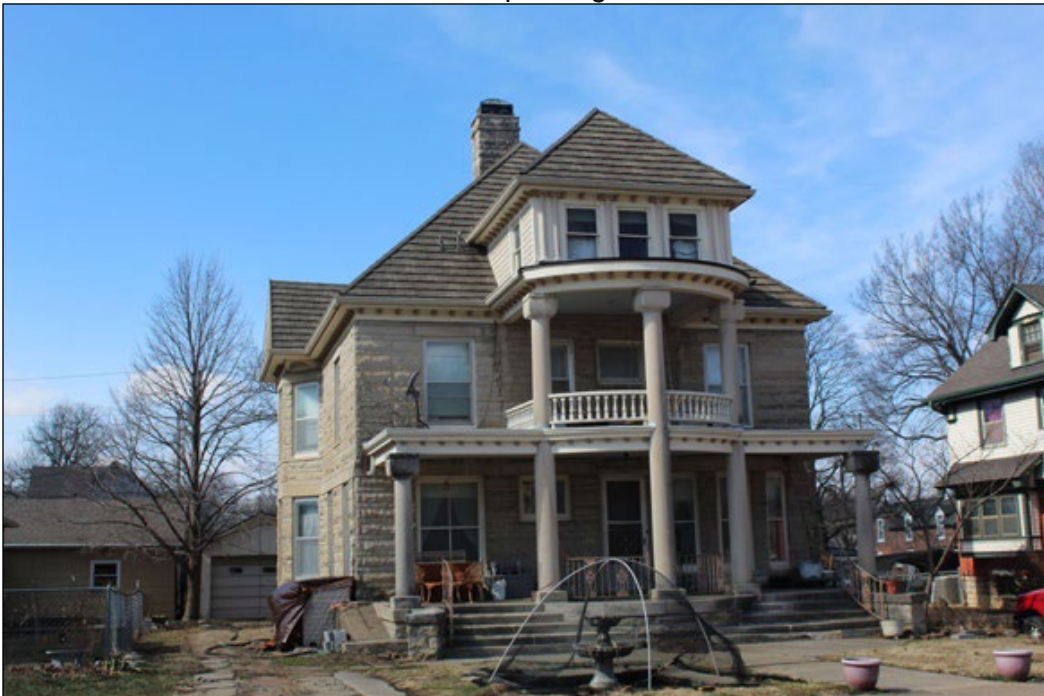
Photo 2. Southeast elevation. Camera pointing northwest.
