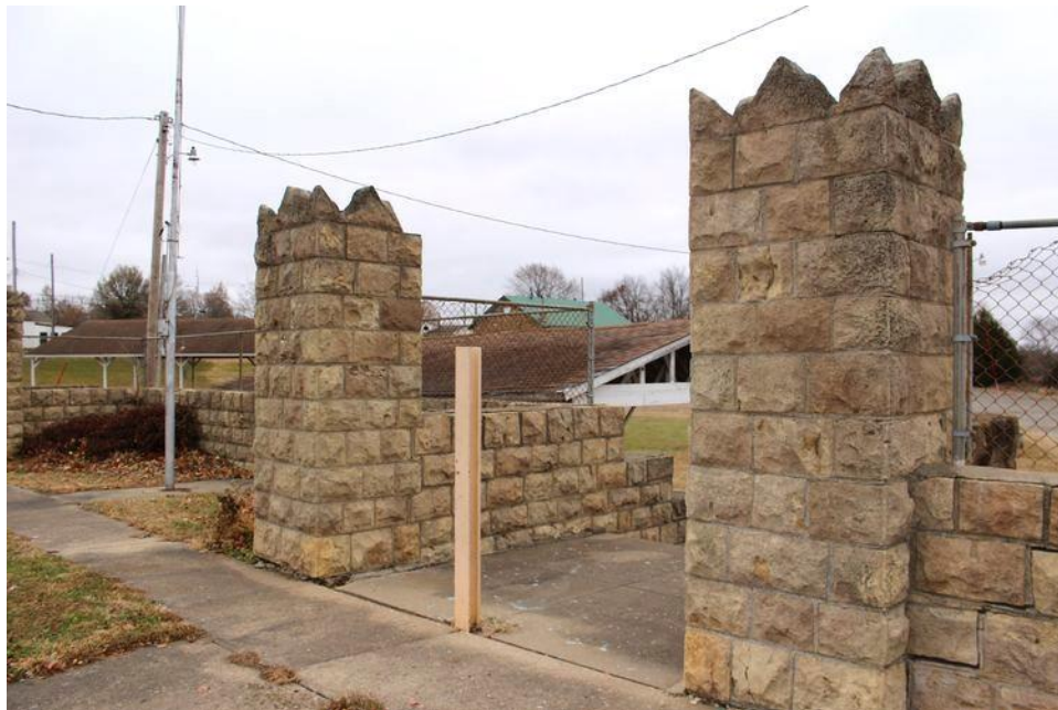
Figure 7: Landscape walls and gate posts constructed of local limestone ca. 1937-1939. Chain link fence date is unknown. Viewed looking southeast 11/21/2019. KSHS.
