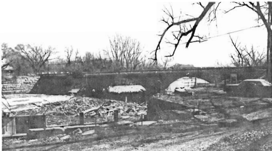
Cottonwood River Bridge west side looking east.
