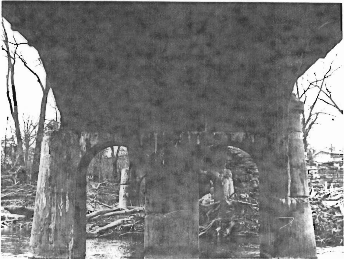
Cottonwood River Bridge substructure looking south.
