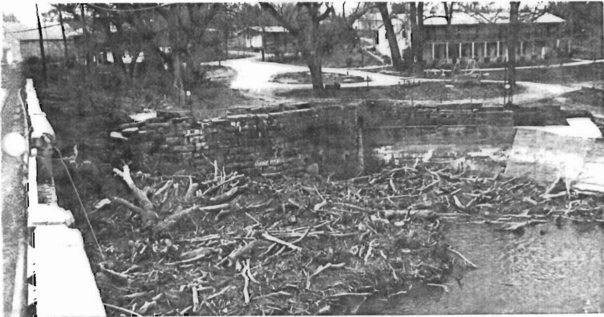
Cottonwood River Bridge looking southeast at remains of old mill.
