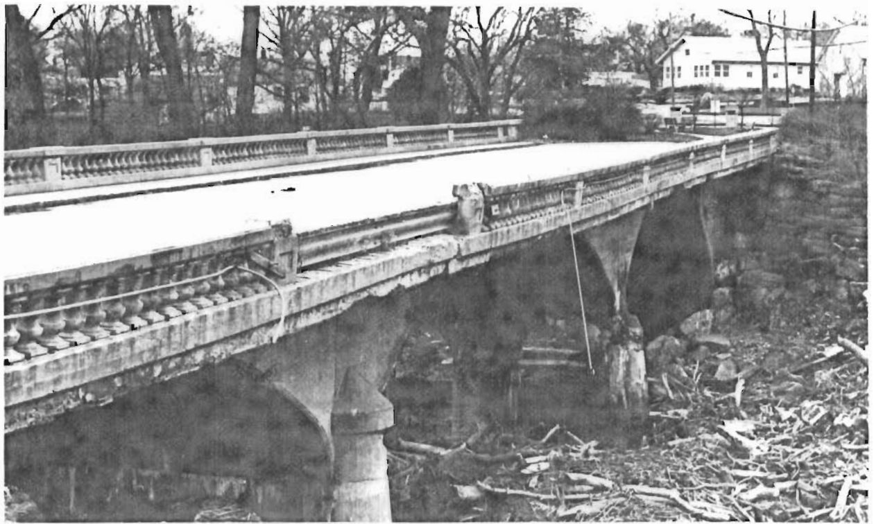
Cottonwood River Bridge west side looking south.
