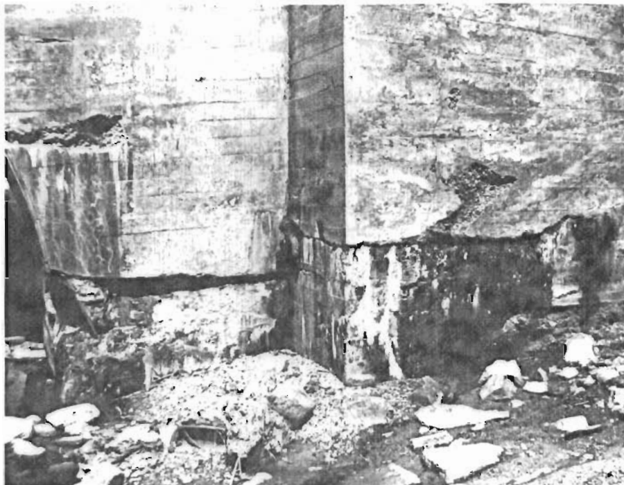
Cottonwood River Bridge east side of north abutment.
