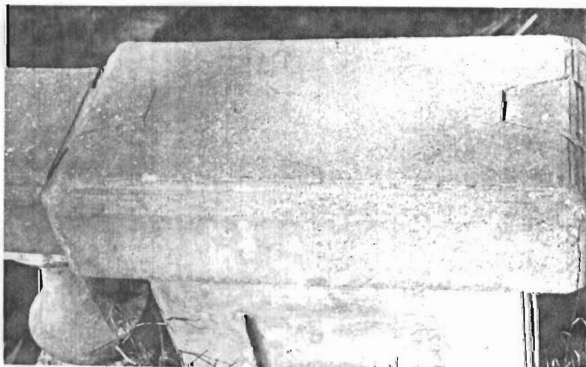
Cottonwood River Bridge tongue and groove railing connection.
