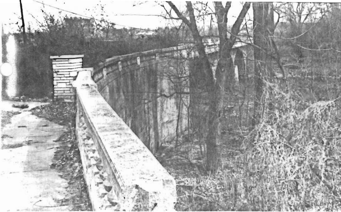
Cottonwood River Bridge east side looking north.
