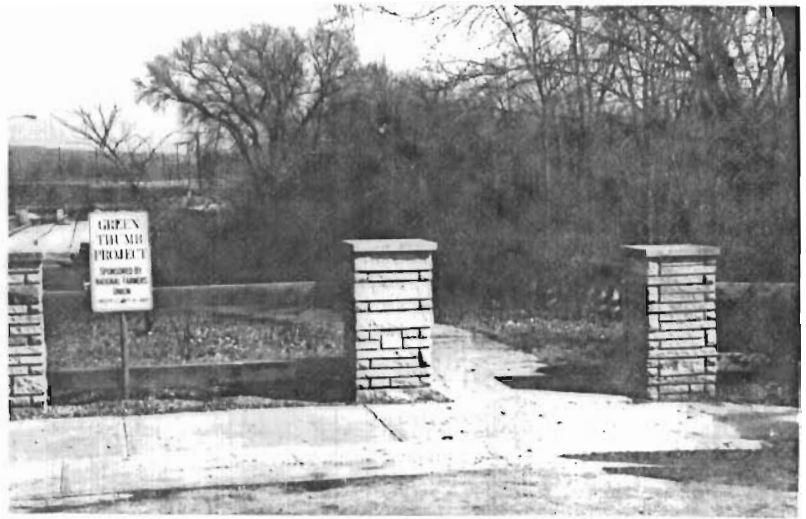
Cottonwood River Bridge entrance to south approach looking northeast.
