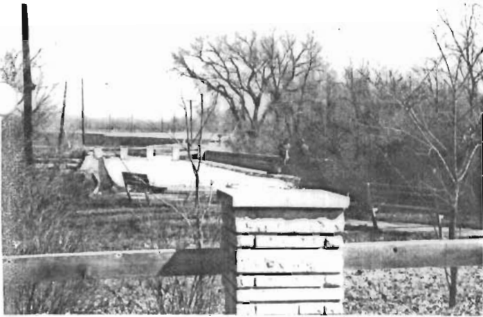
Cottonwood River Bridge park on south approach looking north.
