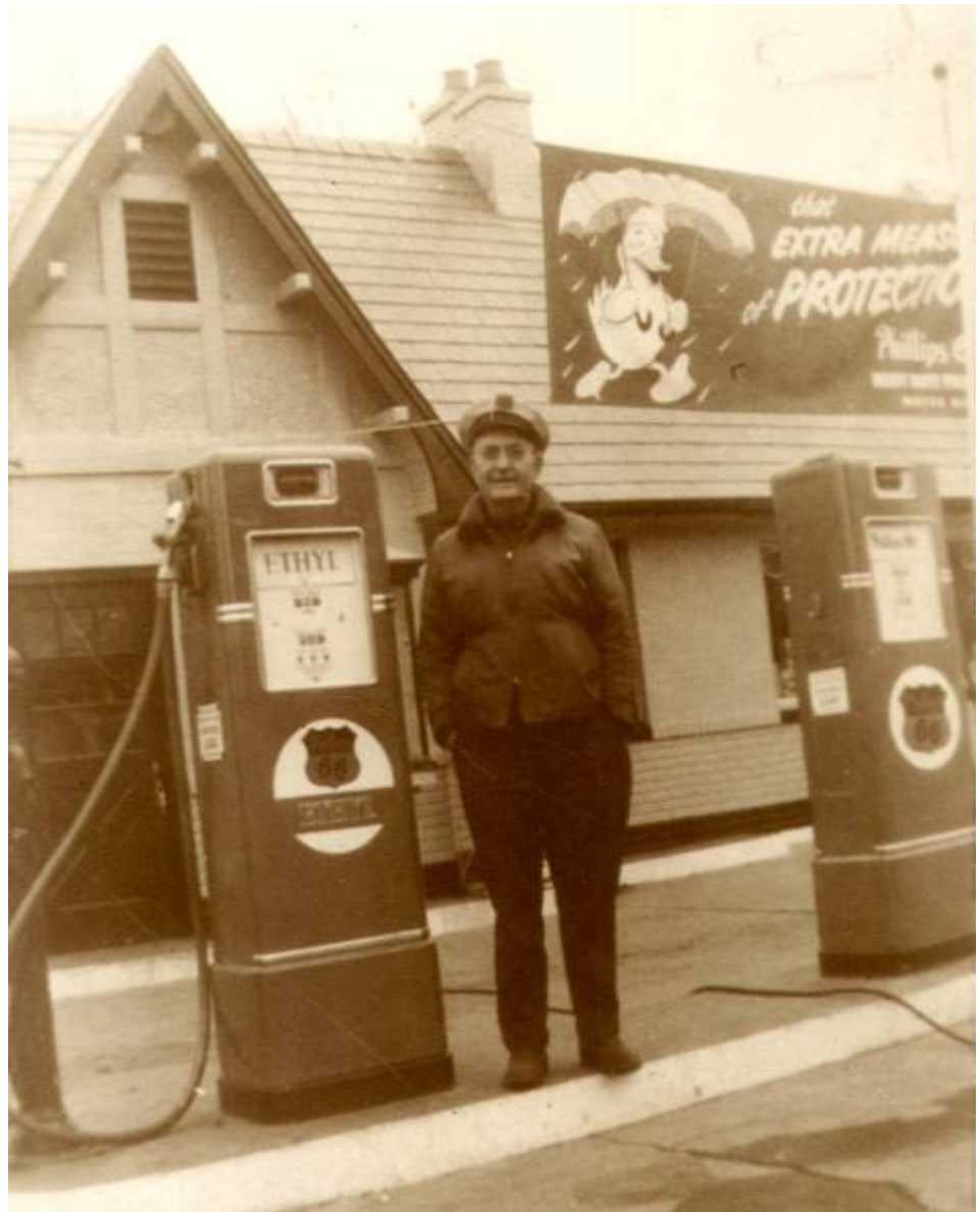
Ray Parsons, Parsons Oil, Tenth and Military, Baxter Springs, Kansas Undated photograph, c.1950's (Baxter Springs Historical Society) In this photo, the building appears to be sporting the tan and maroon color scheme used by Phillips from 1947 to 1959. The gas pumps are Bowser model 575 manufactured by S. F. Bowser & Co. of Ft. Wayne, Indiana, from 1941 to 1948.
