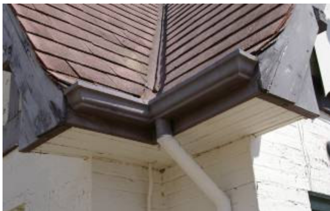
Gutter and downspout at southwest corner
