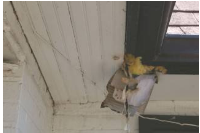
Soffit at inside corner of addition
