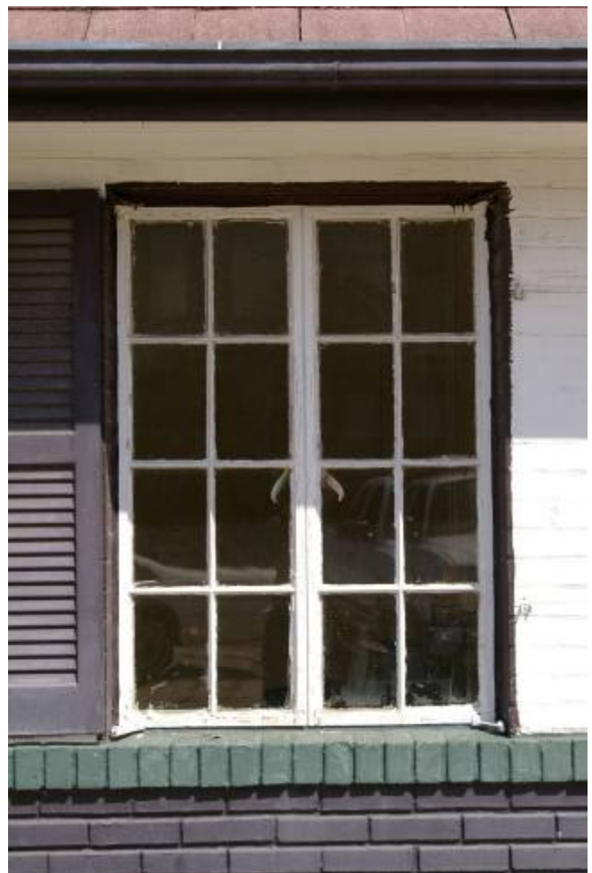
South casement window, original building
