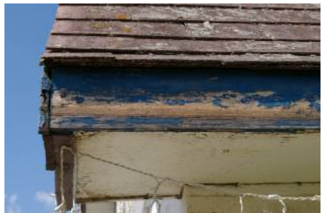
Soffit and trim at southeast corner of garage
