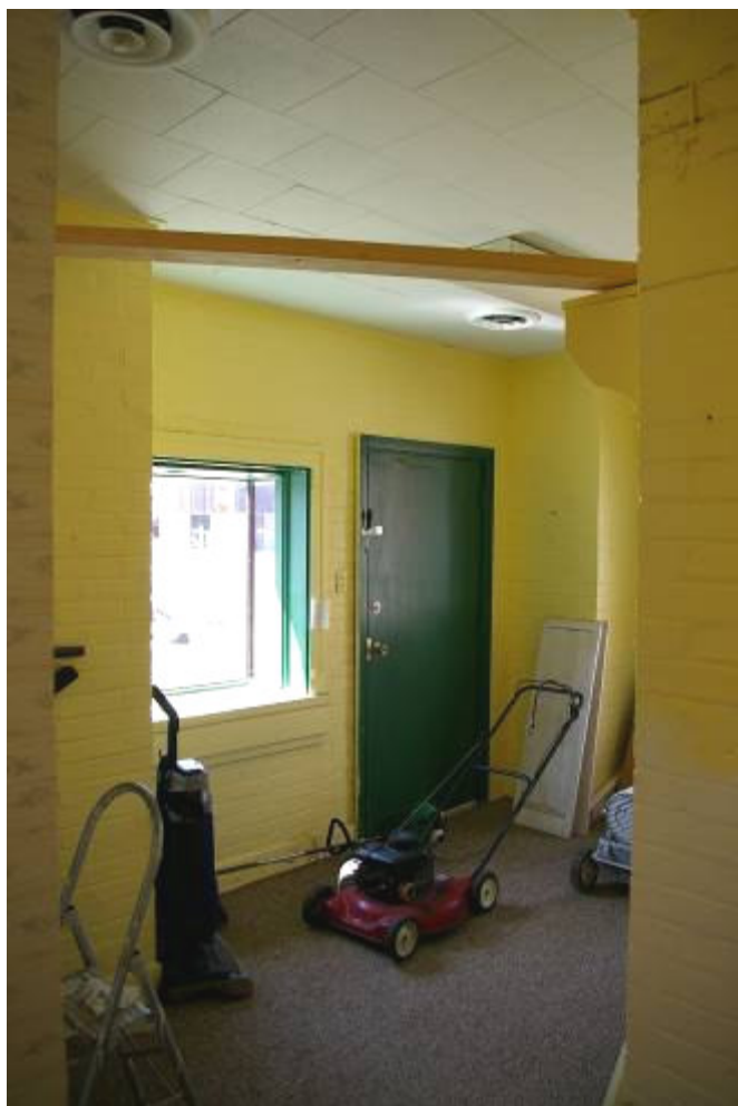
Office looking southwest toward front door
