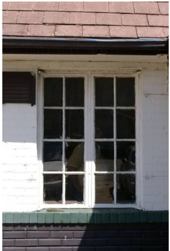
South window, addition
