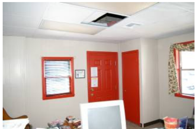
Garage SE area, looking southwest
