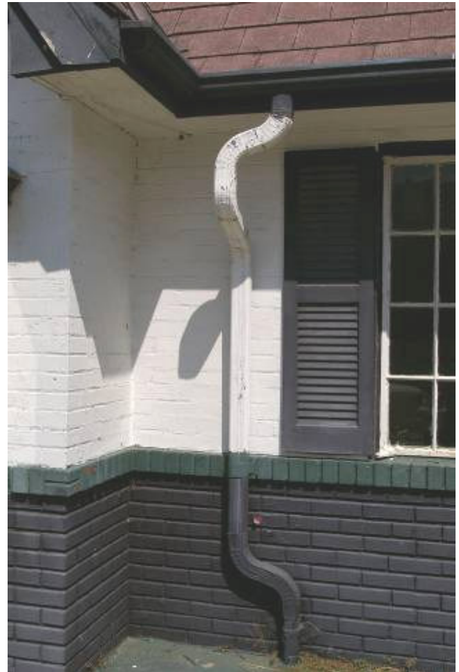
Downspout on south side of original building
