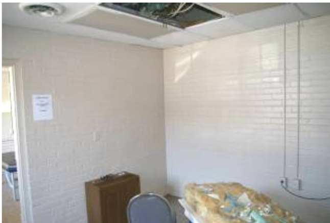
Garage NW area, looking northwest
