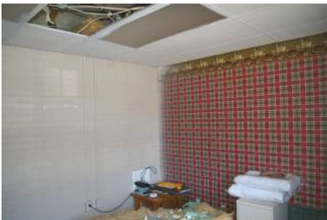
Garage NW area, looking northeast
