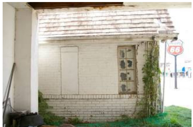
Men's room window on left, ladies' room on right
