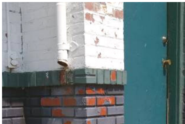
Surface-mounted outlet (left) at southwest corner
