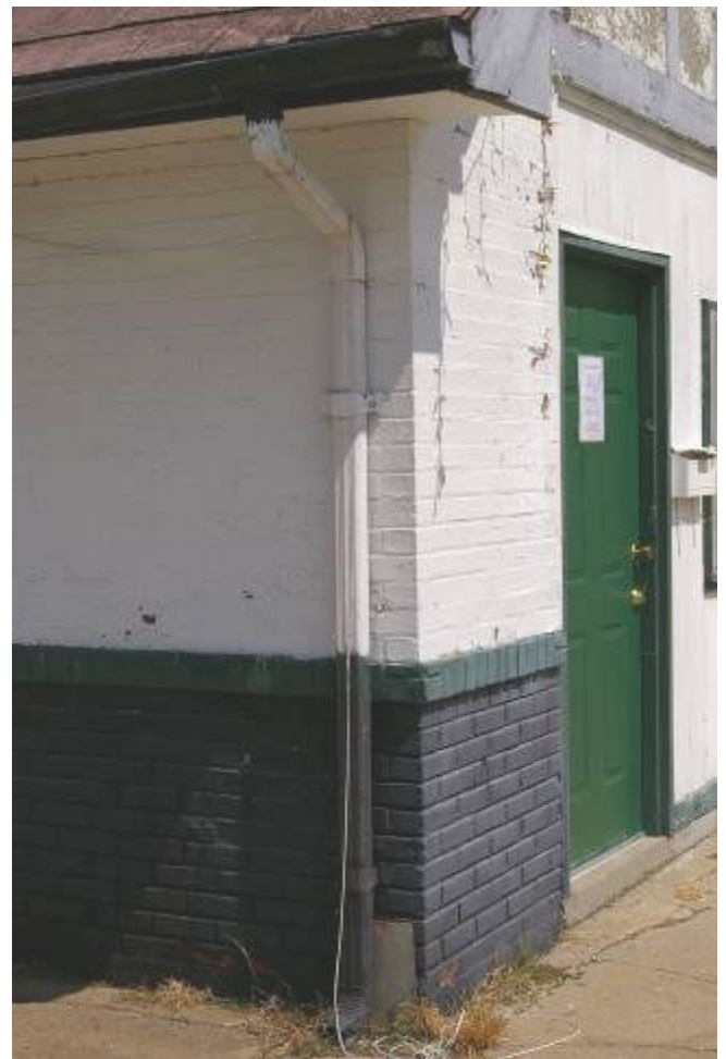
Gutter and downspout, southwest corner of garage
