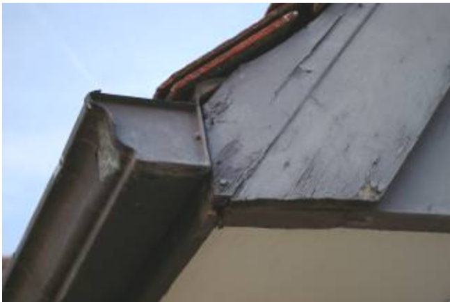
End of gutter on garage addition
