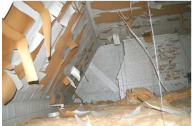
Original sheetrock ceiling
