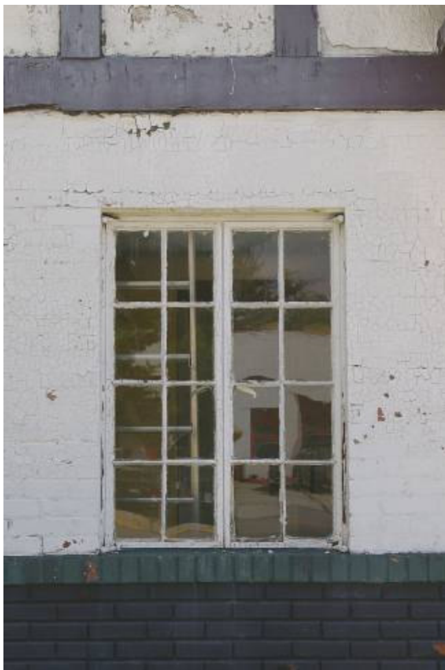
East casement window
