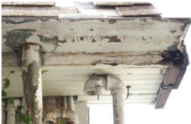
Gutter and downspout at northwest corner
