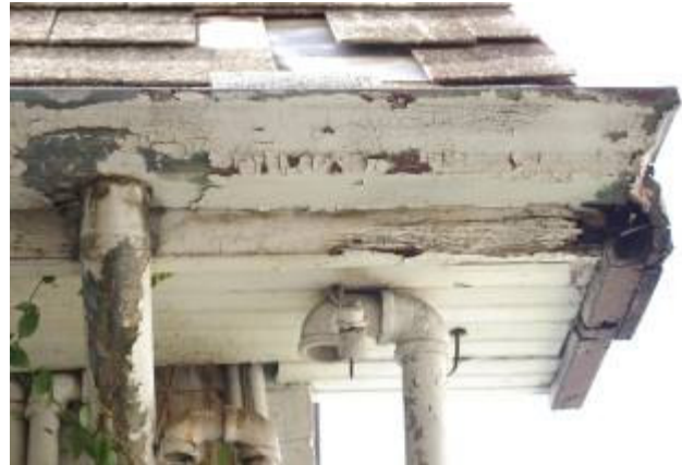
Soffit and trim at northwest corner of building
