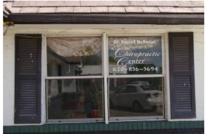
West garage window
