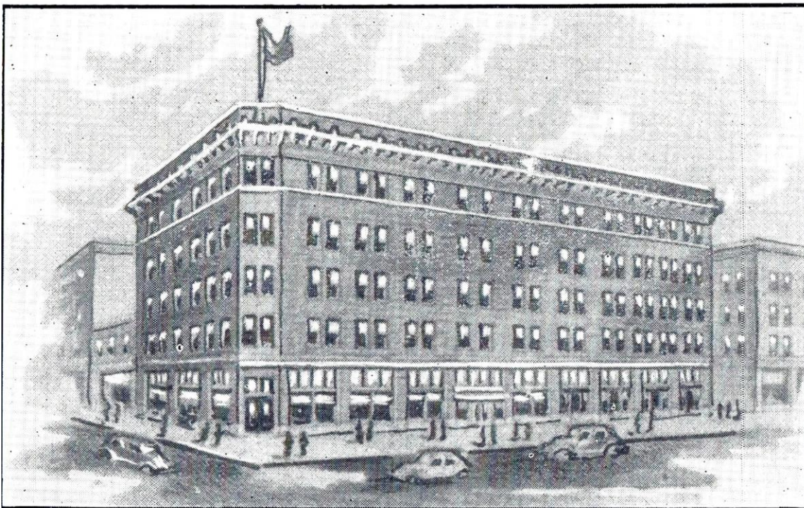
HOTEL McCLELLAN, FIREPROOF — 100 ROOMS ALL WITH BATH
