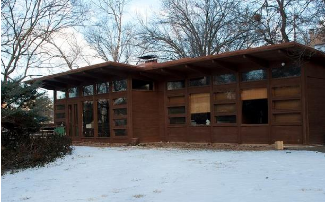
Figure 9. South elevation in 2014 (top) and 1951 (bottom). Top image by John Charlton; bottom image from Lawrence Modern ( http://lawrencemodern.com/bakers-dozen/university-place/post-construction-photos/ ).
