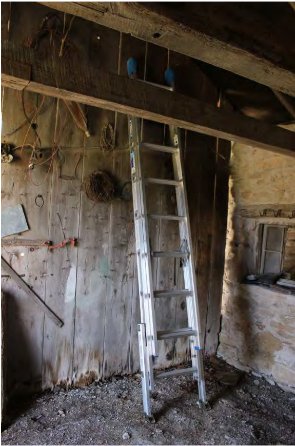
Photo 13: Interior – middle room
