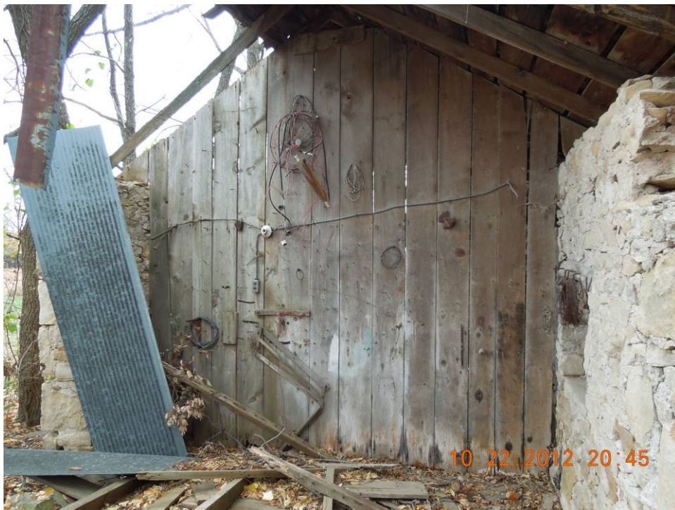
Figure 12: Stone building inside wall south end, chicken coup on other side.
