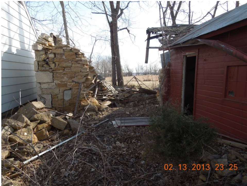
Figure 13: Stone building NW side and north side of shed
