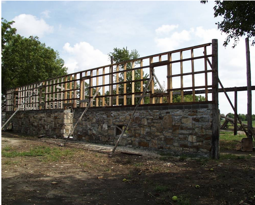
Figure 7: Stable NW outside, wall rebuilt and wood wall added 2001
