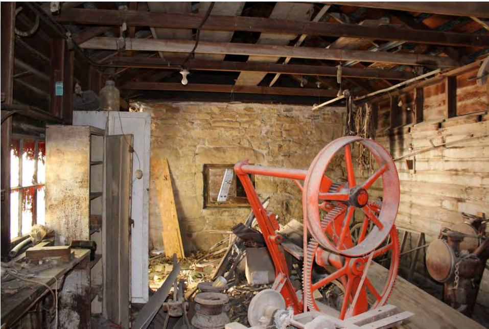
Photo 23: Interior – wood-framed addition looking toward stone building
