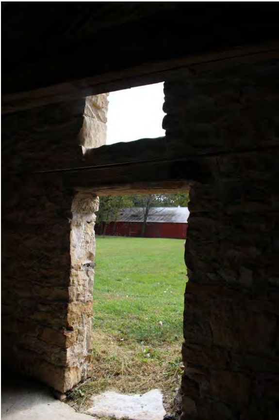
Photo 21: Interior – south room door and window
