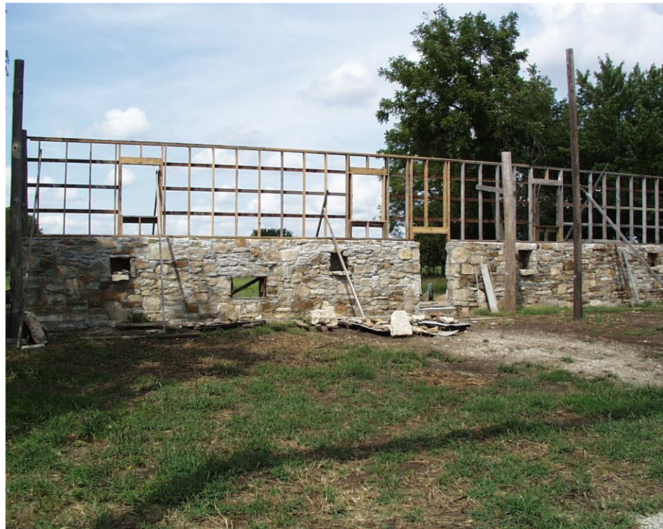
Figure 8: Stable, inside NW end west 2/3 rd rebuilt and wood wall added 2001
