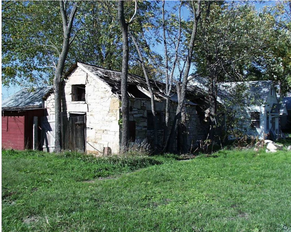
Figure 9: Stone building se view taken 2001
