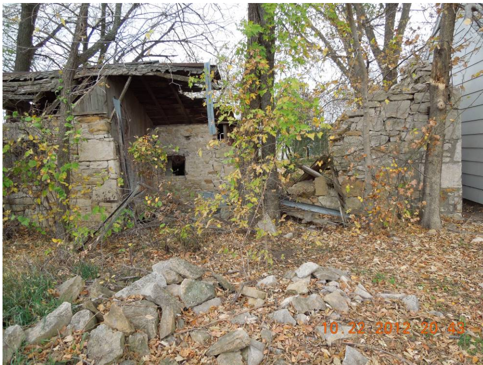
Figure 14: Stone building east wall
