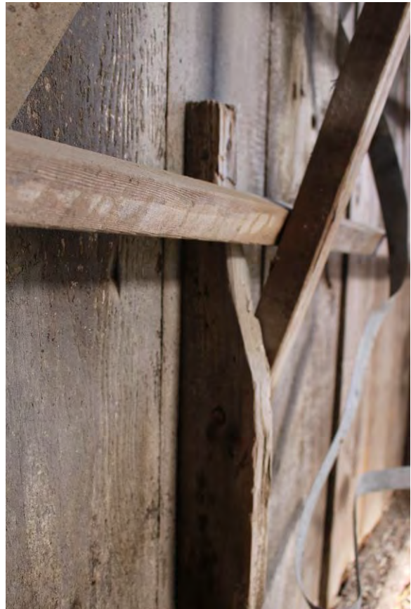
Photo 18: Interior – south room close up
