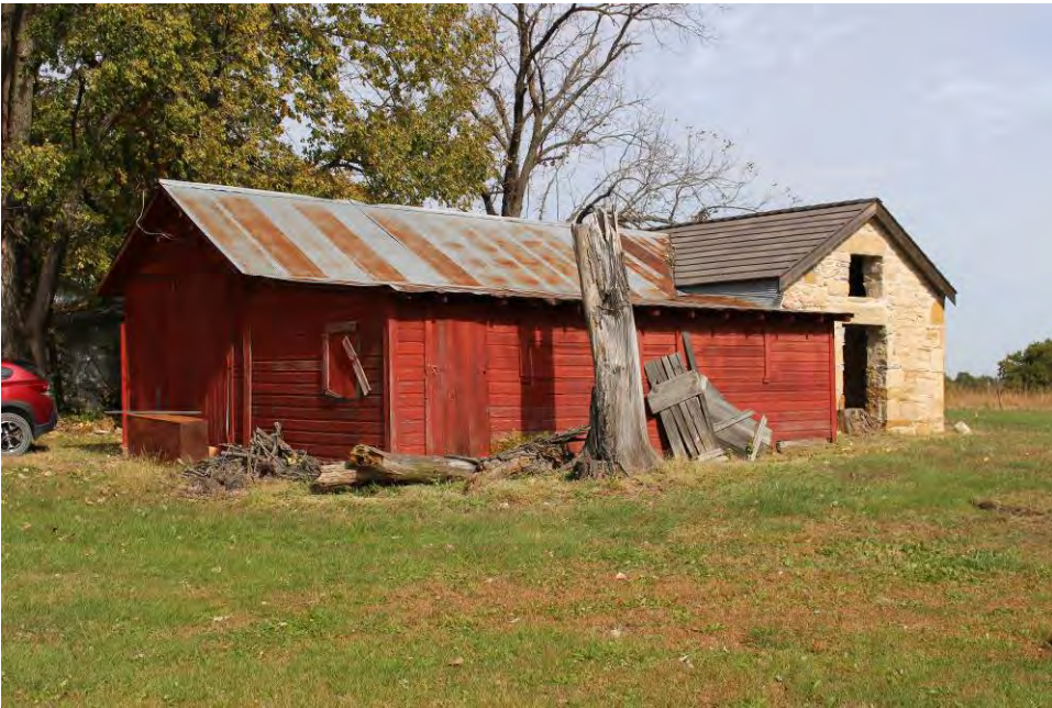
Photo 2: West and south elevations
