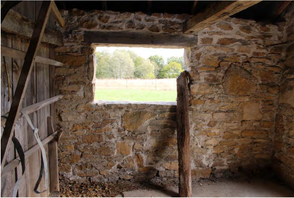
Photo 20: Interior – south room window
