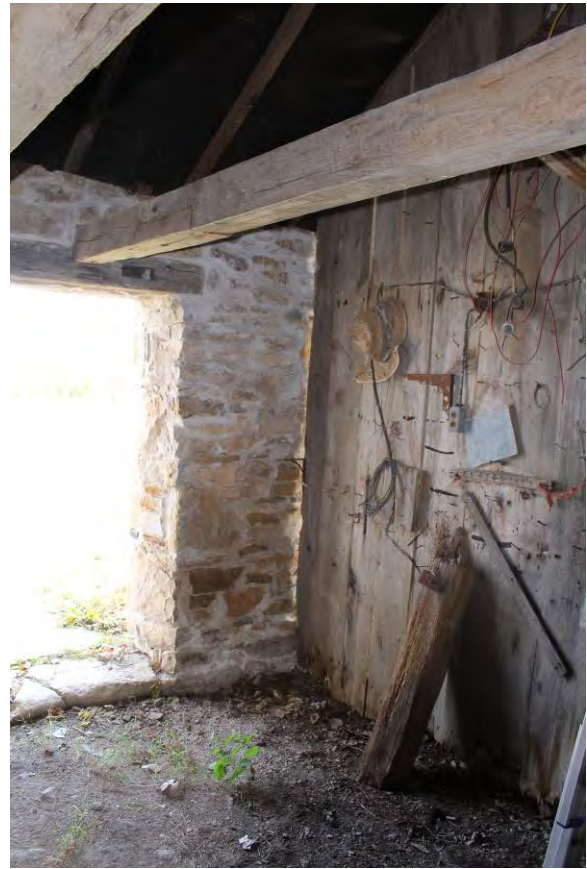
Photo 14: Interior – middle room
