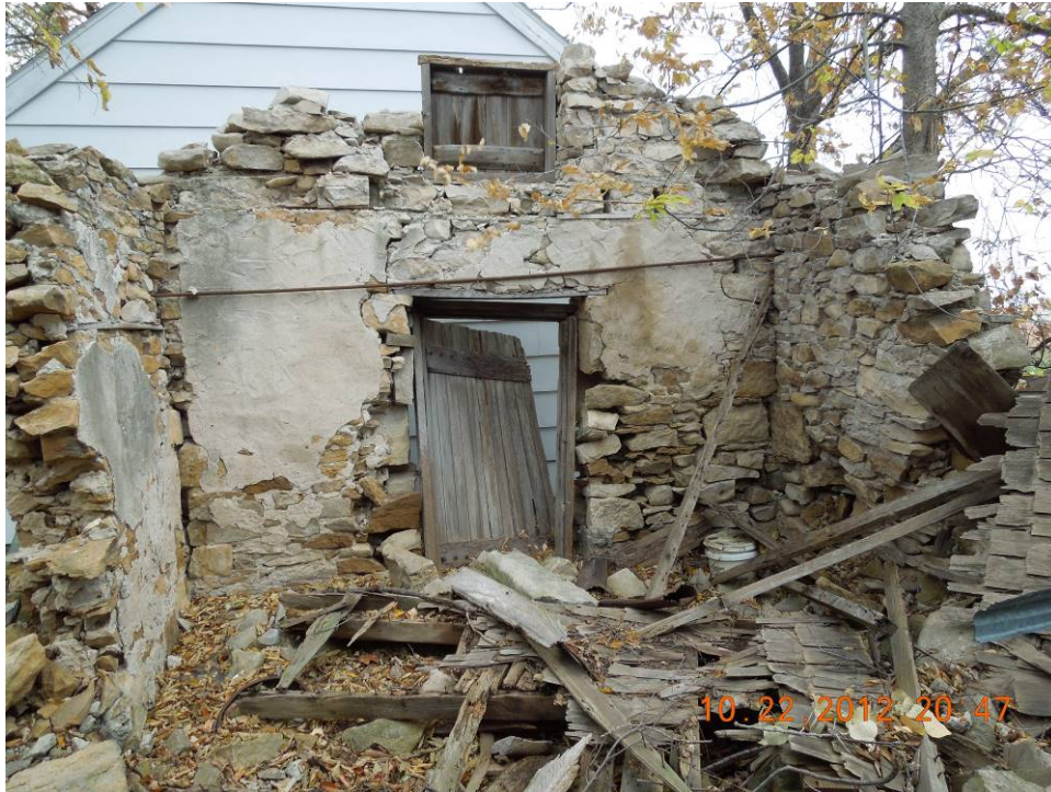
Figure 15: Stone building inside north wall
