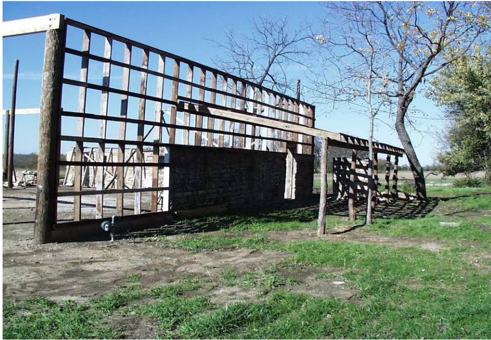
Figure 5: Original outside of east wall of stable. Wood structure added in 2001
