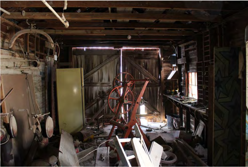
Photo 24: Interior – wood-framed addition looking toward west
