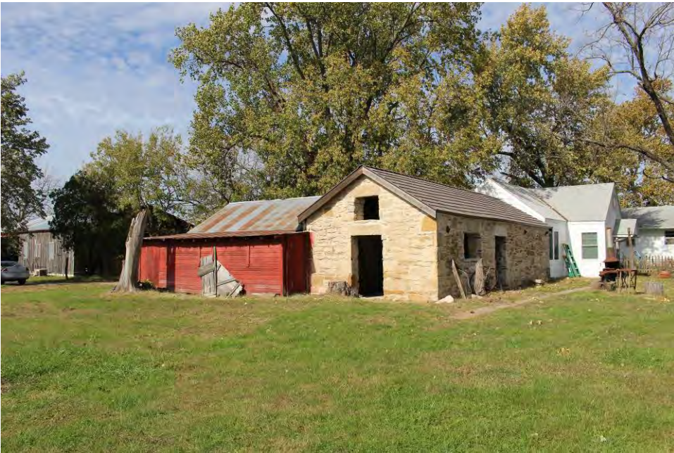
Photo 4: South and east elevations
