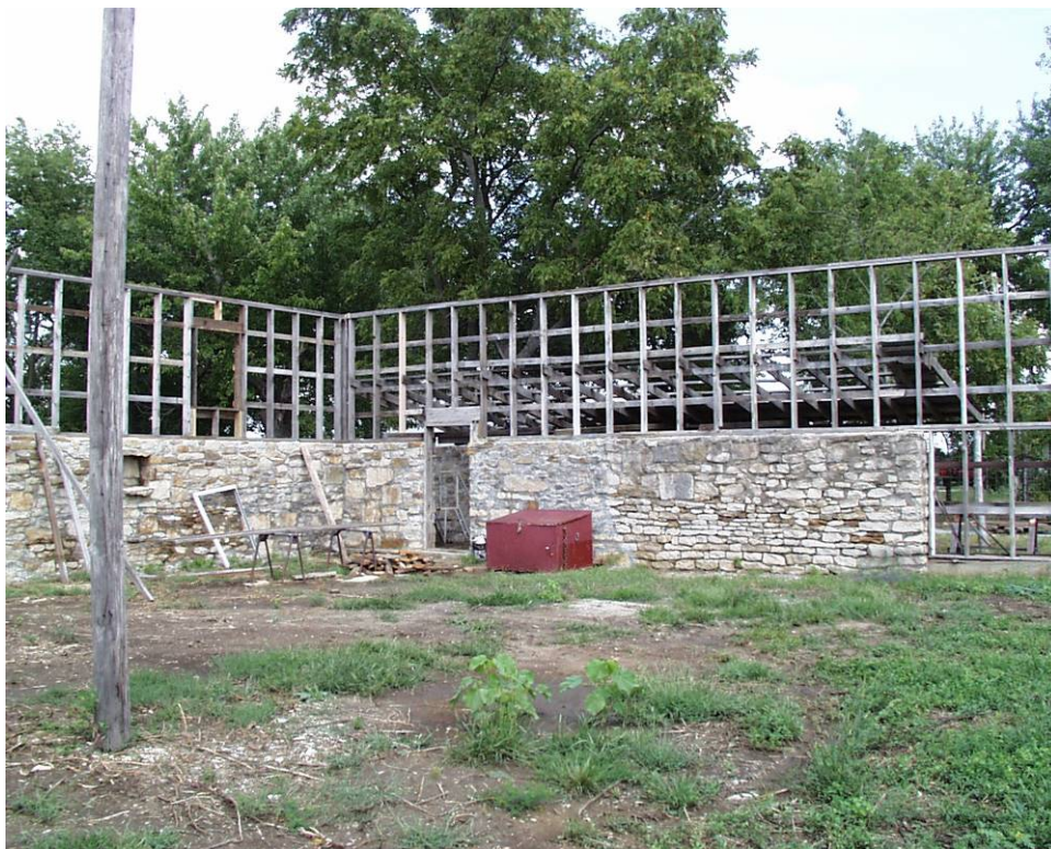
Figure 6: Inside east original wall, wood frame and wall rebuilt to left 2001
