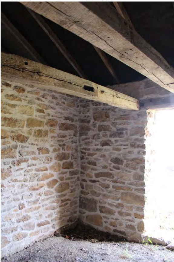
Photo 15: Interior – middle room
