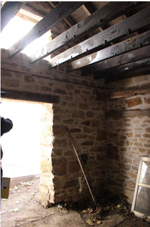
Photo 11: Interior – of north room
