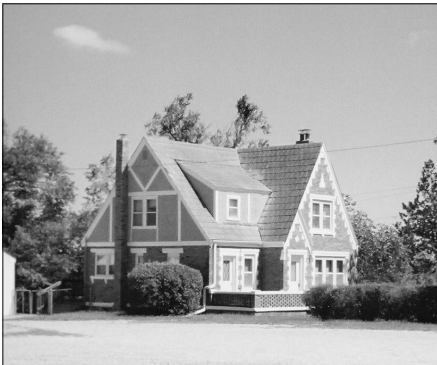
The Methodist Parsonage, still in good condition, stands east of the Church.
