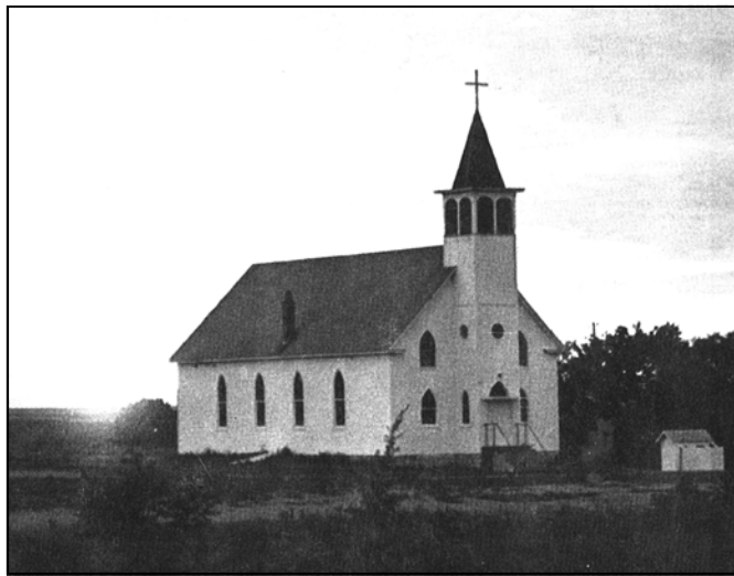
In 1984, St. Peter's Parish Church moved many valued items such as stained glass windows, statues and its cornerstone to the Territorial Capital Museum before it was taken down rather than left standing to face inevitable vandals.
