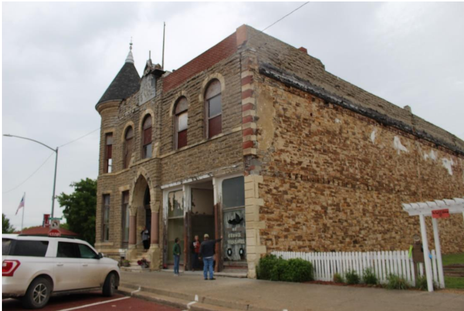
Photo 4: Looking NE – oblique of the south building elevations
