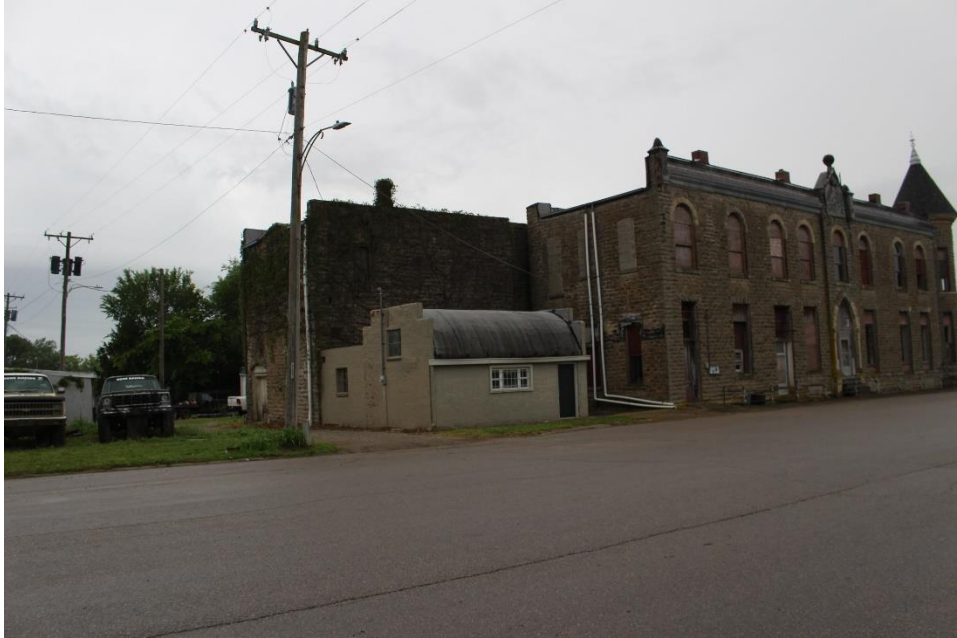
Photo 5: Looking SW – the back of the two buildings and the small building in the “el”
