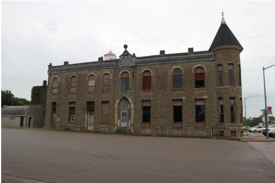
Photo 3: Looking S – the north façade of the Bank
