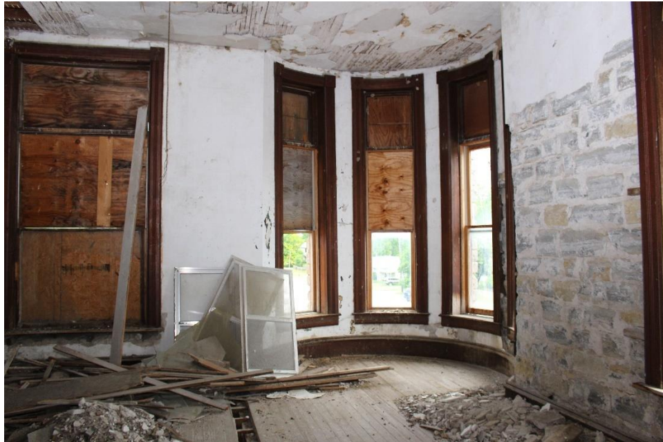
Photo 15: Looking W – 2 nd floor interior – turret room
