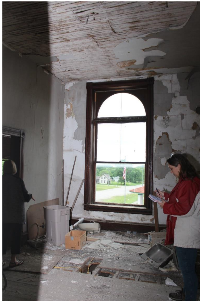
Photo 16: Looking N – 2 nd floor interior – turret room
