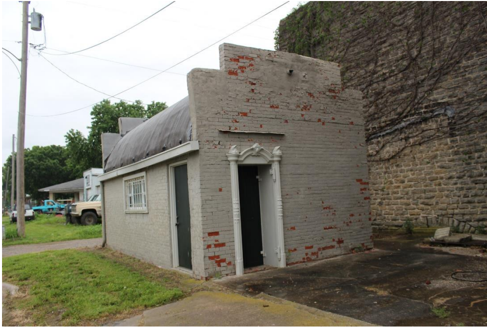
Photo 32: Adjacent property within the "ell"
