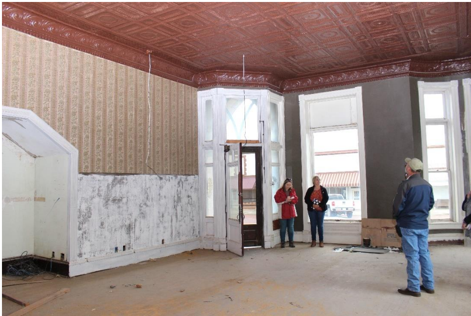
Photo 8: Looking SW – interior of the main Bank lobby
