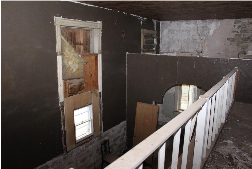
Photo 14: Looking E – interior view of the back third of the Bank
