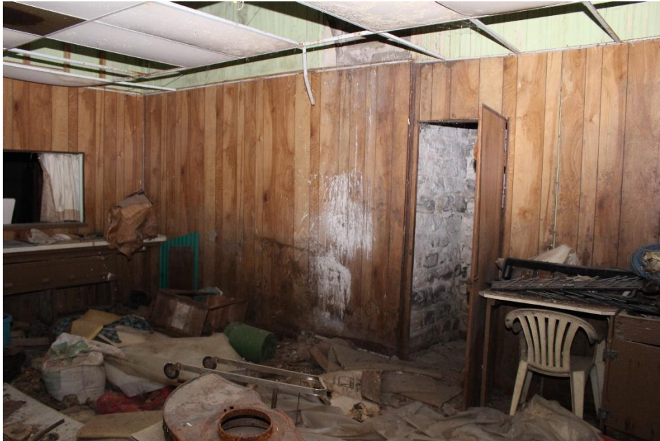
Photo 26: Looking SE – first floor of 149 Wabash
