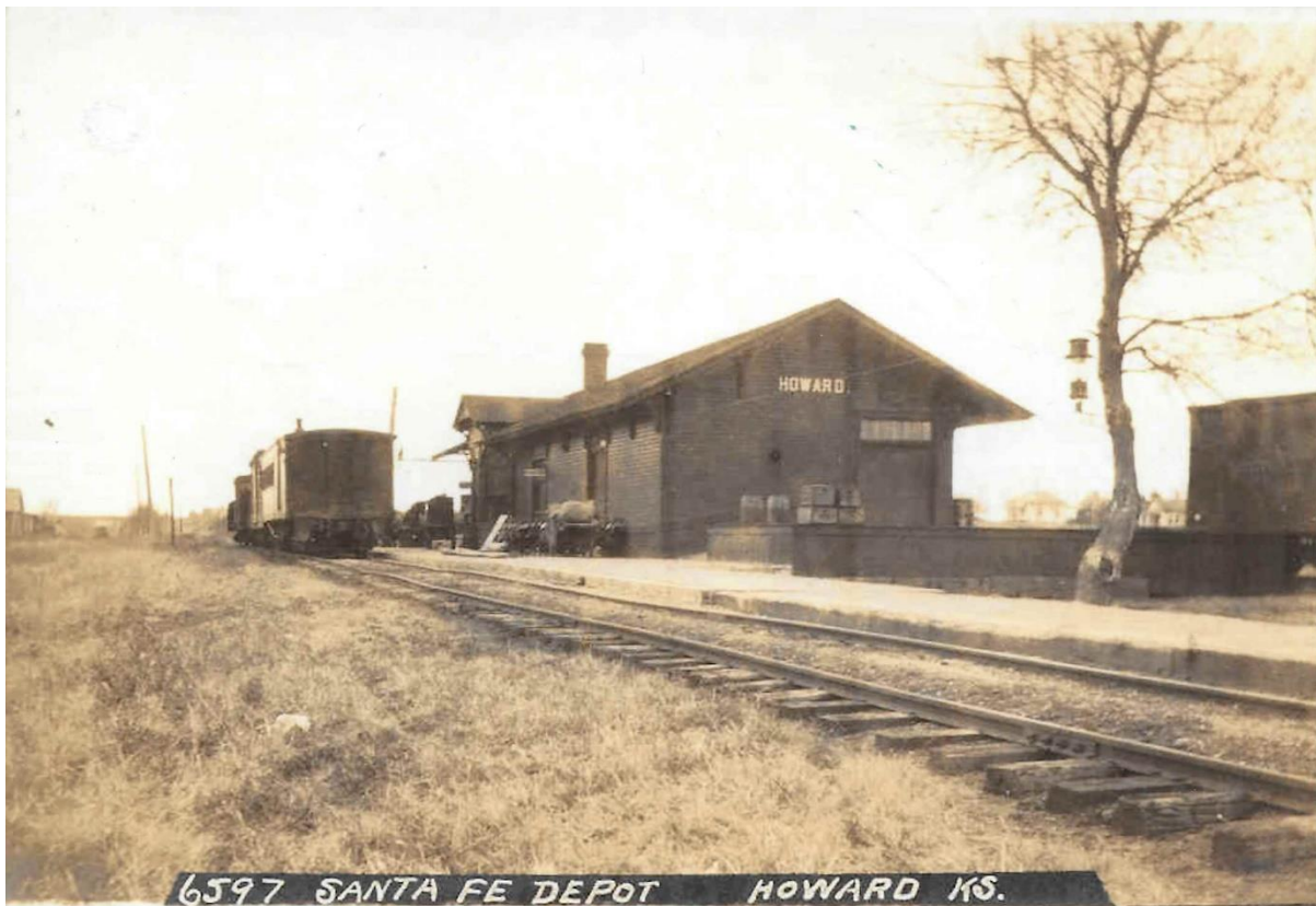
Figure 4: Santa Fe Depot west side of Howard, Kansas. Built in 1879, closed in May 1975.
