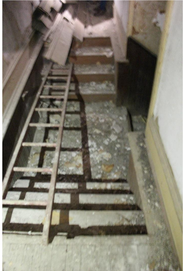
Photo 18: 2 nd floor – looking at the stair to the elevator
