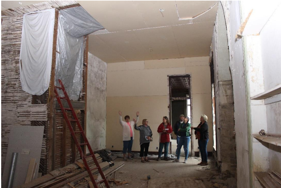
Photo 11: Looking W – interior of the middle portion of the Bank building
