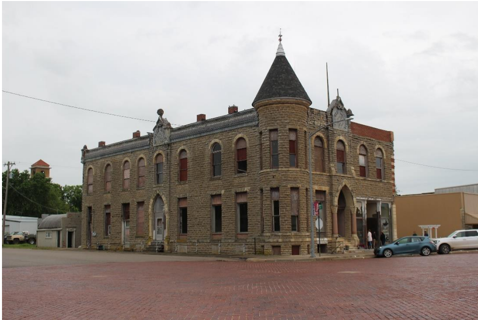
Photo 1: Looking SW – oblique of the two buildings facing the main and north facades
