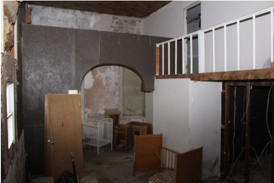
Photo 13: Looking E – interior view of the back third of the Bank
