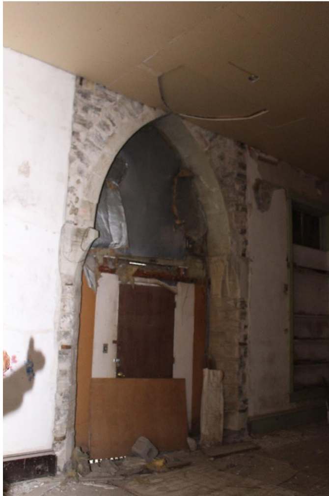
Photo 12: Looking NE – interior view of the Washington entrance to the Bank
