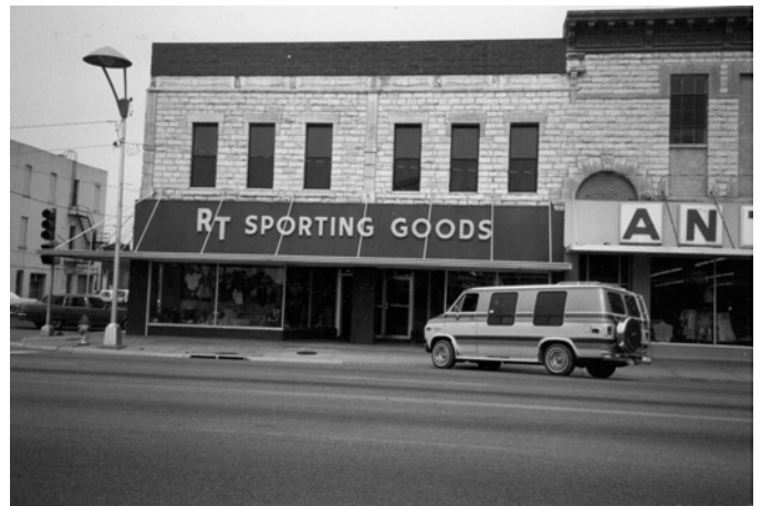
1991 view after removal of third floor and installation of block parapet
