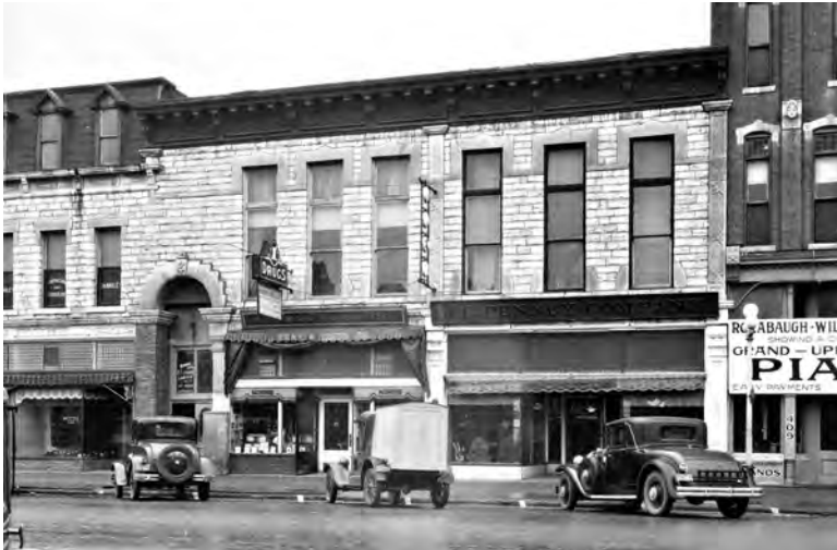
ca. 1930 view of Stevens Building/Masonic Hall with Norris Drug (405) and J.C. Penney (407) Note brick sheathing over south cast-iron column at arched entry to second floor.
