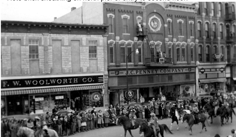
1946 parade photo illustrating F.W. Woolworth at 407 with new downsized steel windows on upper floor; former Stevens Opera House on right with ground floor occupied by J.C. Penney Figure 9 – Historic Views of J.A. Stevens Building/Masonic Hall at 407 N. Main All historic photos courtesy of Finney County Historical Museum in Garden City.
