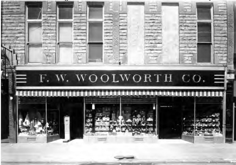
ca. early 1940s view of Stevens Building/Masonic Hall after 1931 remodeling and 1941 expansion of Woolworth to occupy entire first floor – Note brick sheathing on north pier of entry to second floor.
