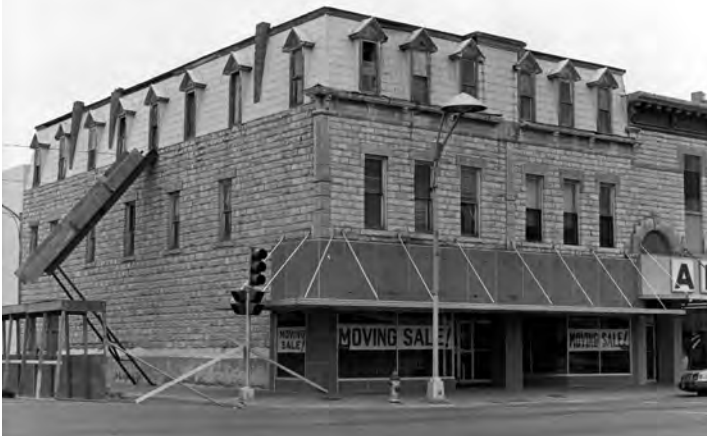
1985 view prior to removal of third floor
