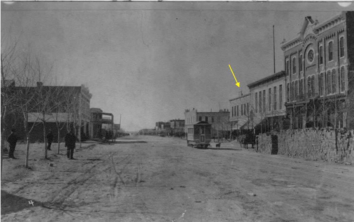
1887 view looking south in 400 block of N. Main Street. Bricks stacked along the west side (R) reflect construction of the Windsor Hotel underway just out of the photo to the north. NOTE – The building at 401 N. Main is extant as a two-story building.
