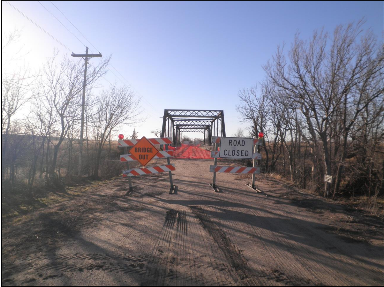
Figure 5. Mulberry Creek Truss Bridge looking west. Photograph taken on January 21, 2014.
