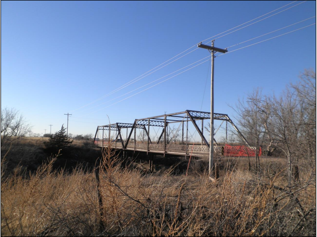
Figure 4. Mulberry Creek Truss Bridge looking northwest. Photograph taken on January 21, 2014.
