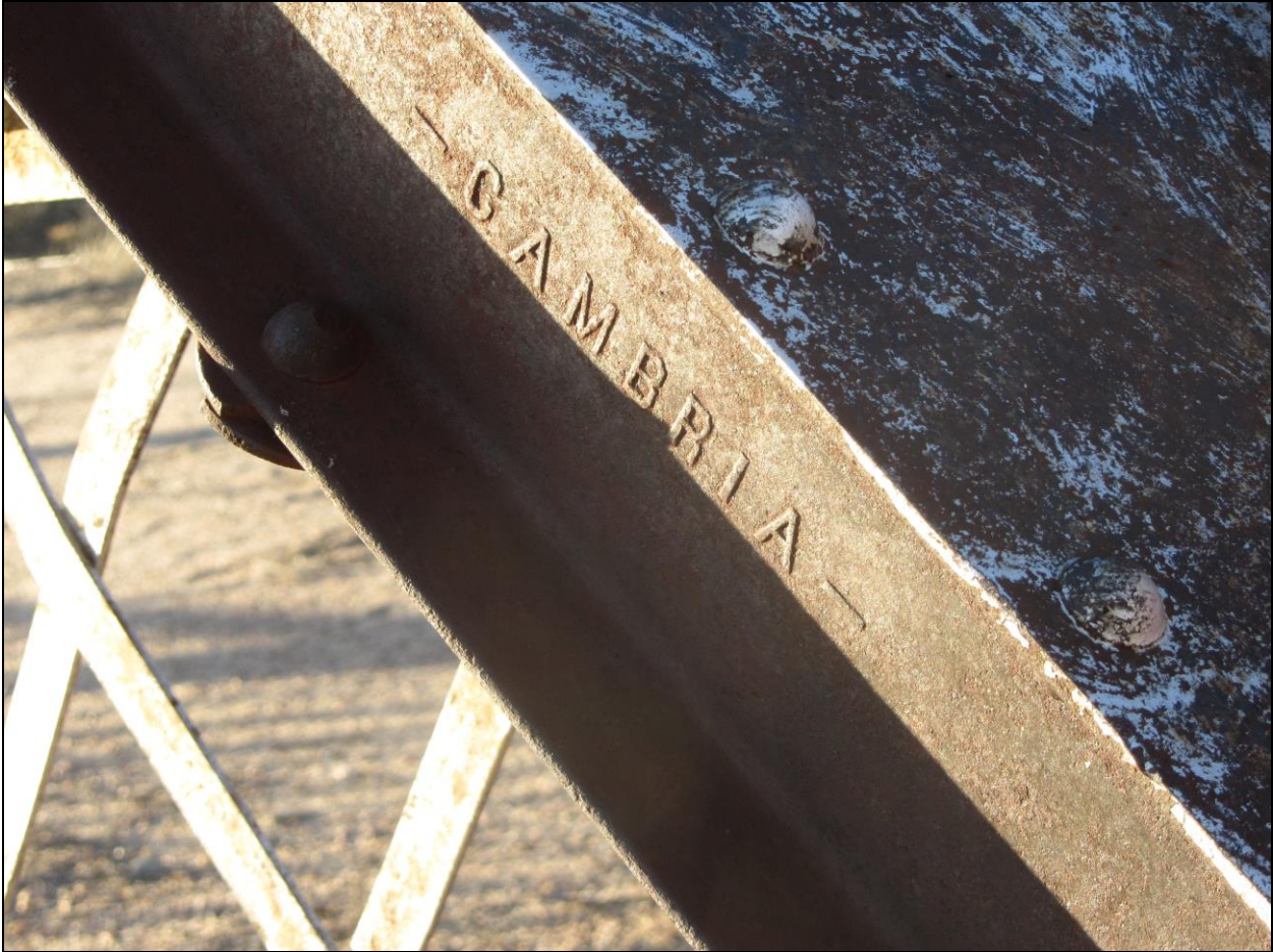
Figure 6. Mulberry Creek Truss Bridge – makers mark. Photograph taken on February 19, 2014.
