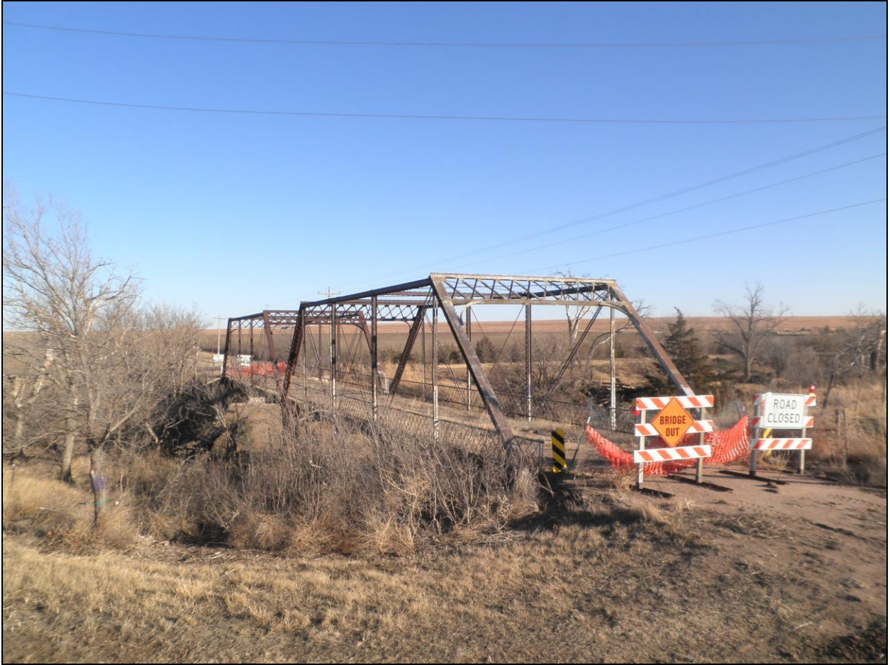
Figure 2. Mulberry Creek Truss Bridge looking southeast. Photograph taken on January 21, 2014.
