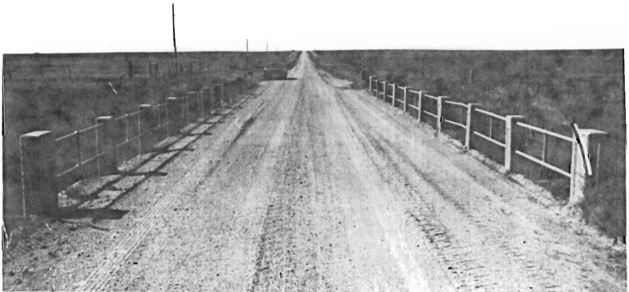
Hackberry Creek Bridge, north approach looking south.
