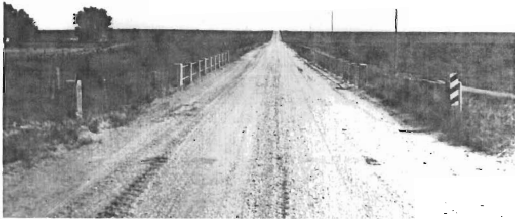
Hackberry Creek Bridge, south approach looking north.
