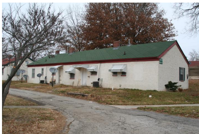
Figure 13 – Current views of residential buildings with exteriors dating to early 1970s remodeling by Hansen including: stucco finish on concrete block walls, porch added at front entry and shutters installed at windows. Some homes retain the metal slat awnings also installed in the early 1970s. (Spencer December 2013 and March 2014)
