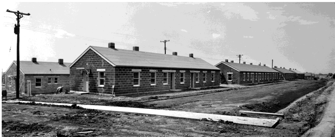
Figure 7 – Four-plex and Six- plex residential buildings (L to R) seen shortly after construction - prior to block being painted - June 24, 1943 FPHA photo by Harkins Commercial Photo (Courtesy of Johnson County Museum)
