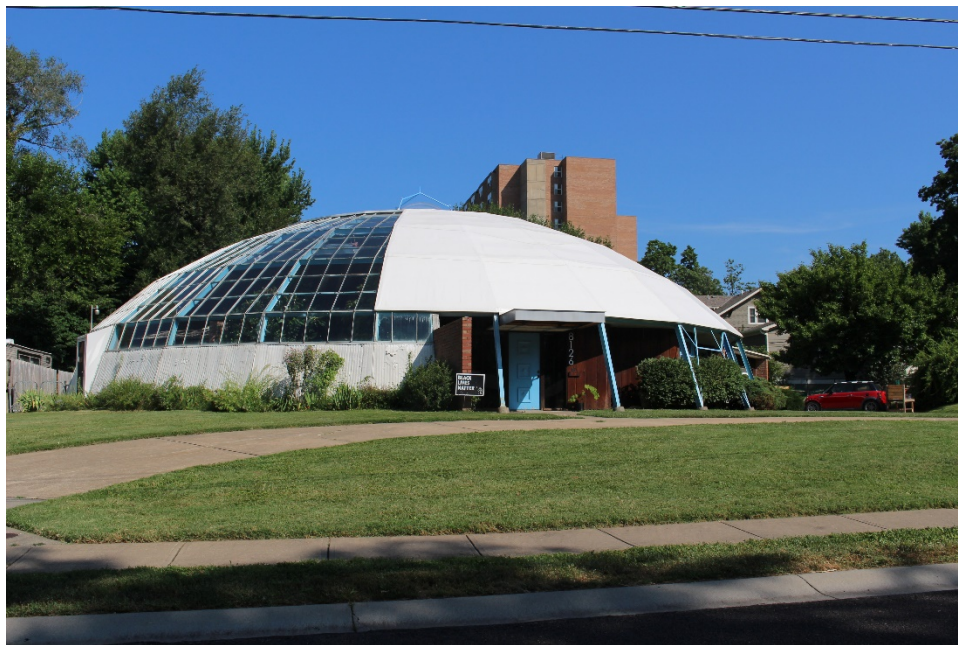
View of the courtyard windows (south) and entrance (southeast)
