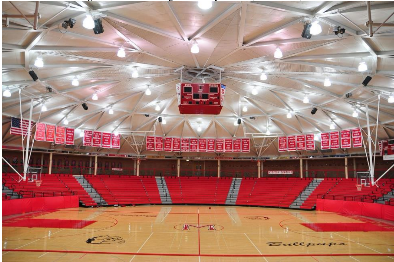
Figure 8 McPherson High School Gymnasium, McPherson, KS
