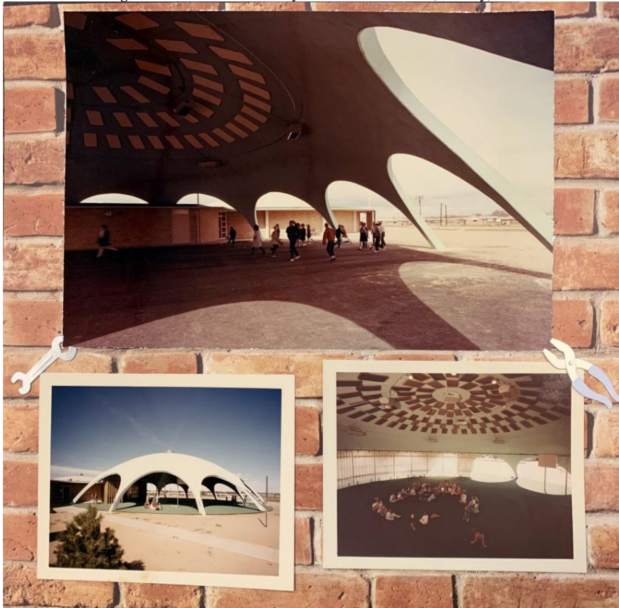
Figure 10 Sherwood Elementary School Dome Pavilion, Greeley, CO
