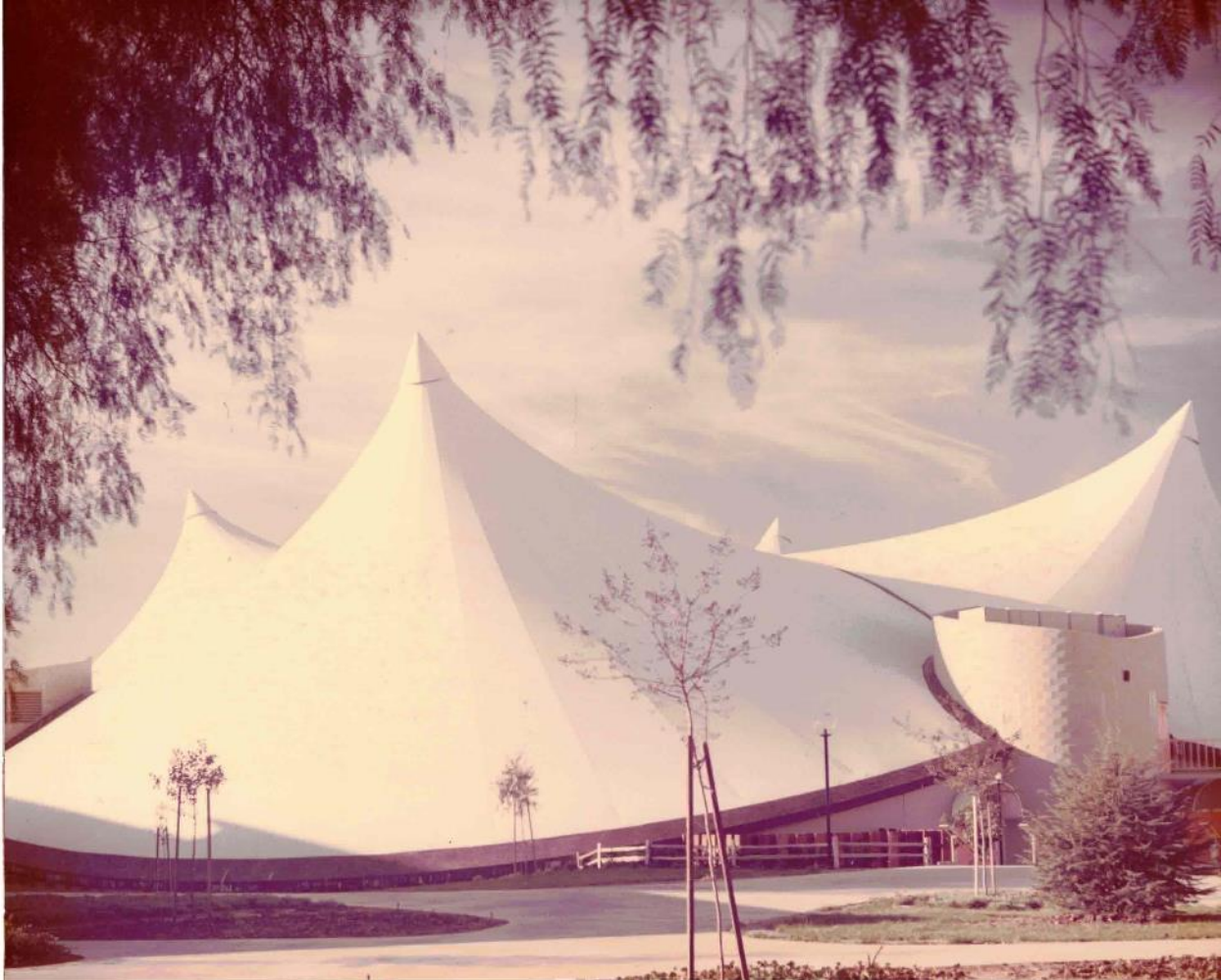
Figure 6 La Verne University – Tension Fabric Roof Design
