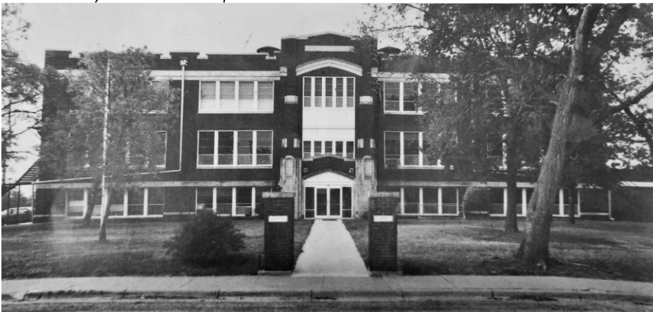
Figure 10 – ca. 1990 view of school (replacement windows and doors in place at most openings) 1991 Lincoln High School Centennial Booklet, Lincoln Carnegie Library
