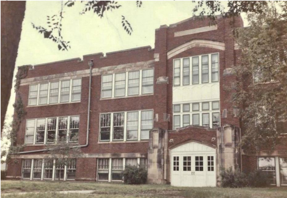
Figure 9 - ca.1970s of front of school (new storm windows in place at some windows-dark frames) Lincoln County Economic Development Foundation
