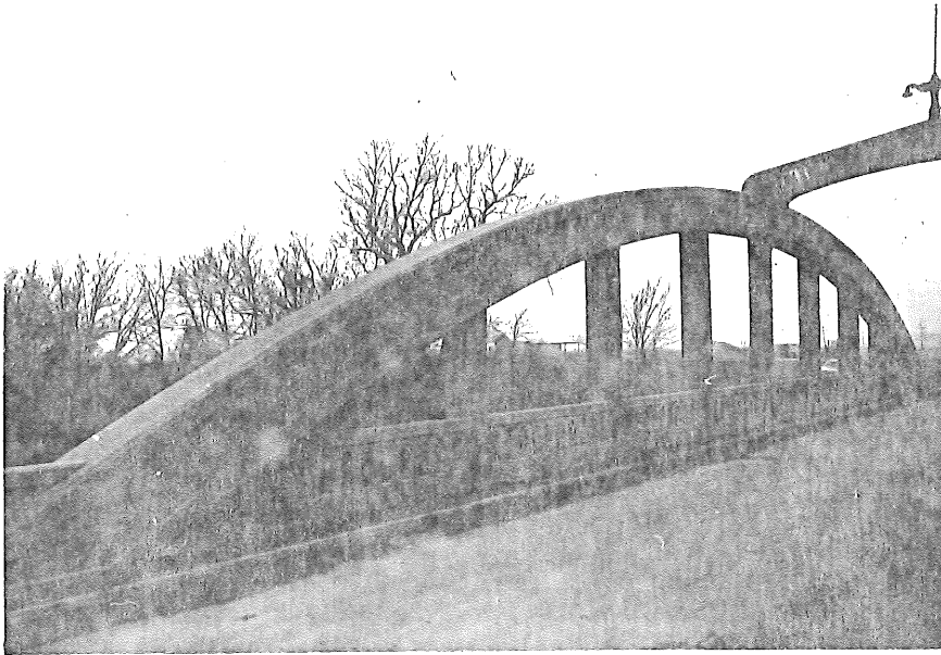
Cottonwood River Bridge South arch looking southwest.
