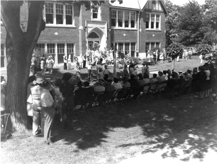
View of school from southwest.
