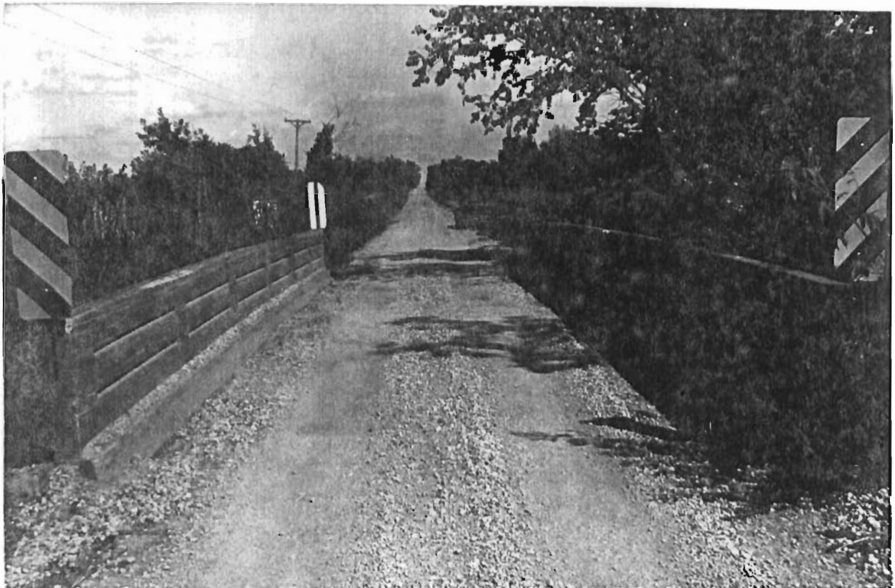
Jake's Branch Bridge. West approach looking east.
