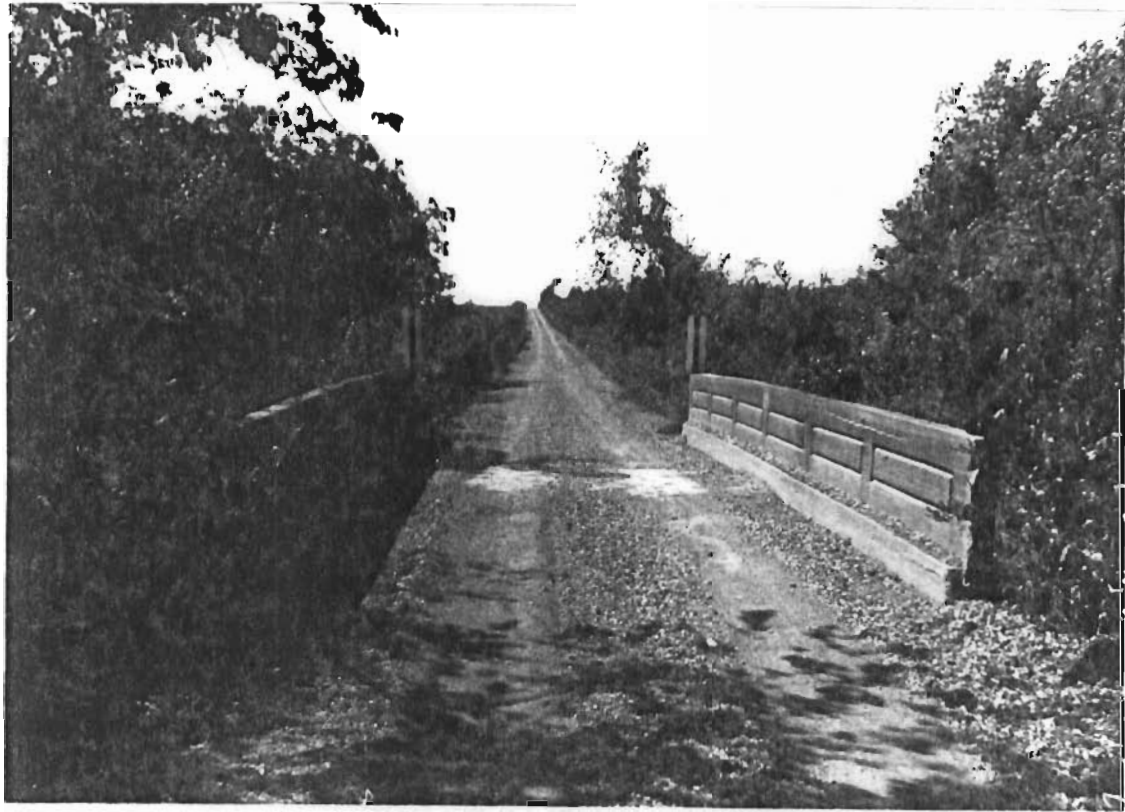
Jake's Branch Bridge. East approach looking west.
