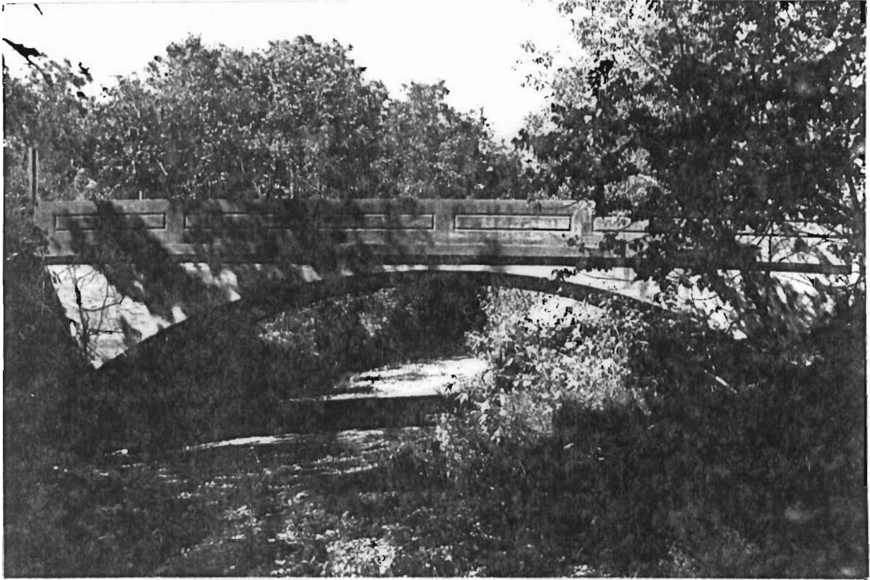
Jake's Branch Bridge. South side looking north.
