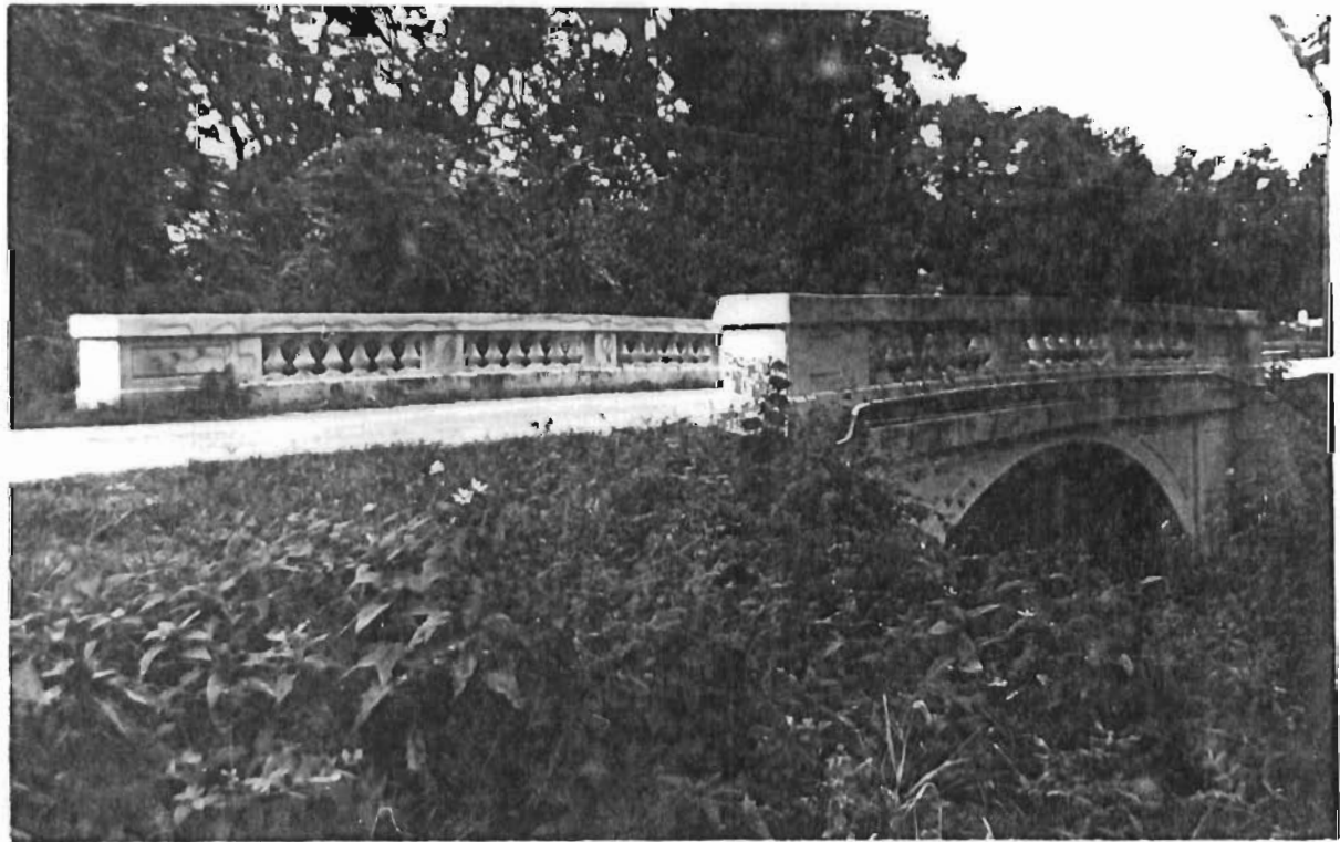
State Street Bridge. North Side Looking Southwest.
