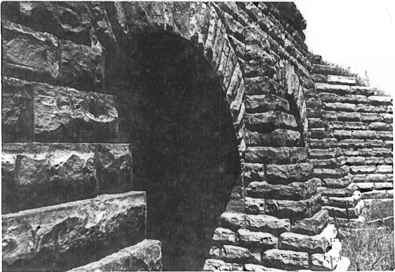
Pawnee River Tributary Bridge. Detail of East Side.
