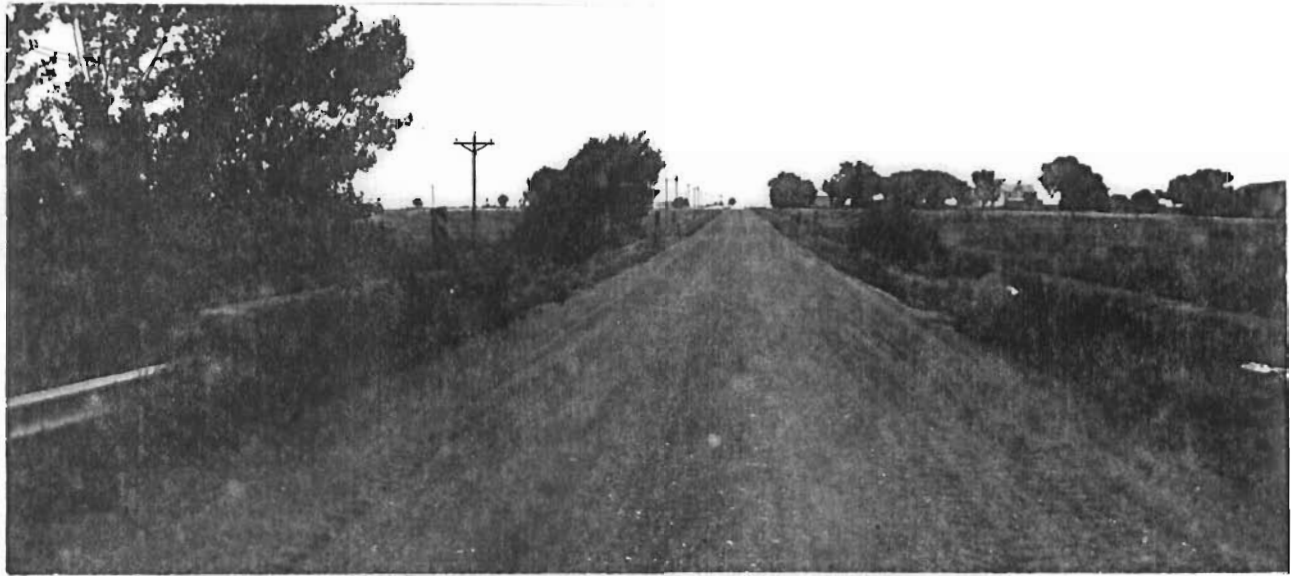
Pawnee River Tributary Bridge. South Approach Looking North
