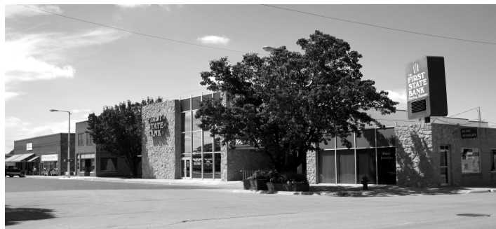
Preservation Solutions LLC
