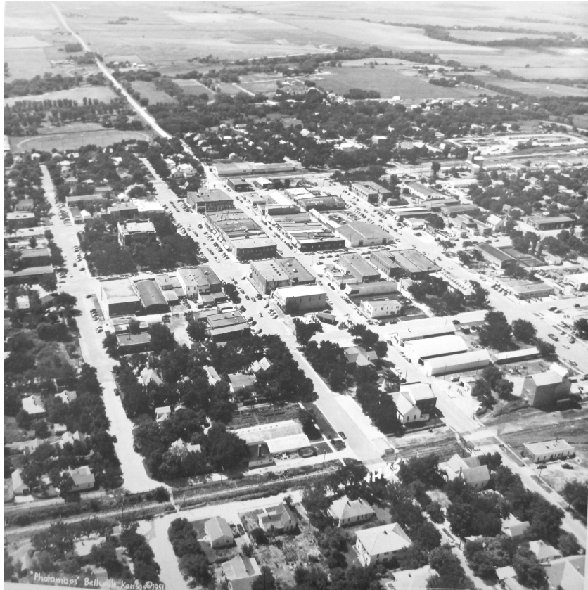
FIGURE 11: 1951 aerial view southwest of downtown Norton
