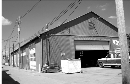
Preservation Solutions LLC
