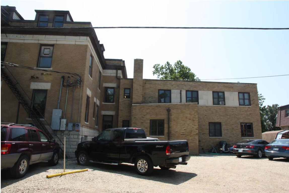
North elevation, west (1958) addition at right.
