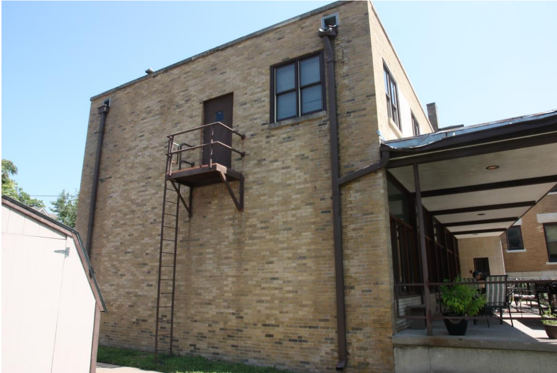
West elevation of 1958 addition.
