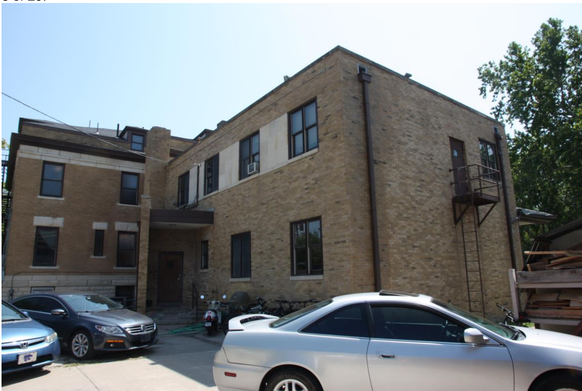
West elevation, from the northwest.
