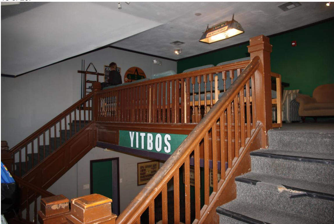
Interior - Third floor landing, looking up and northeast. Original building.
