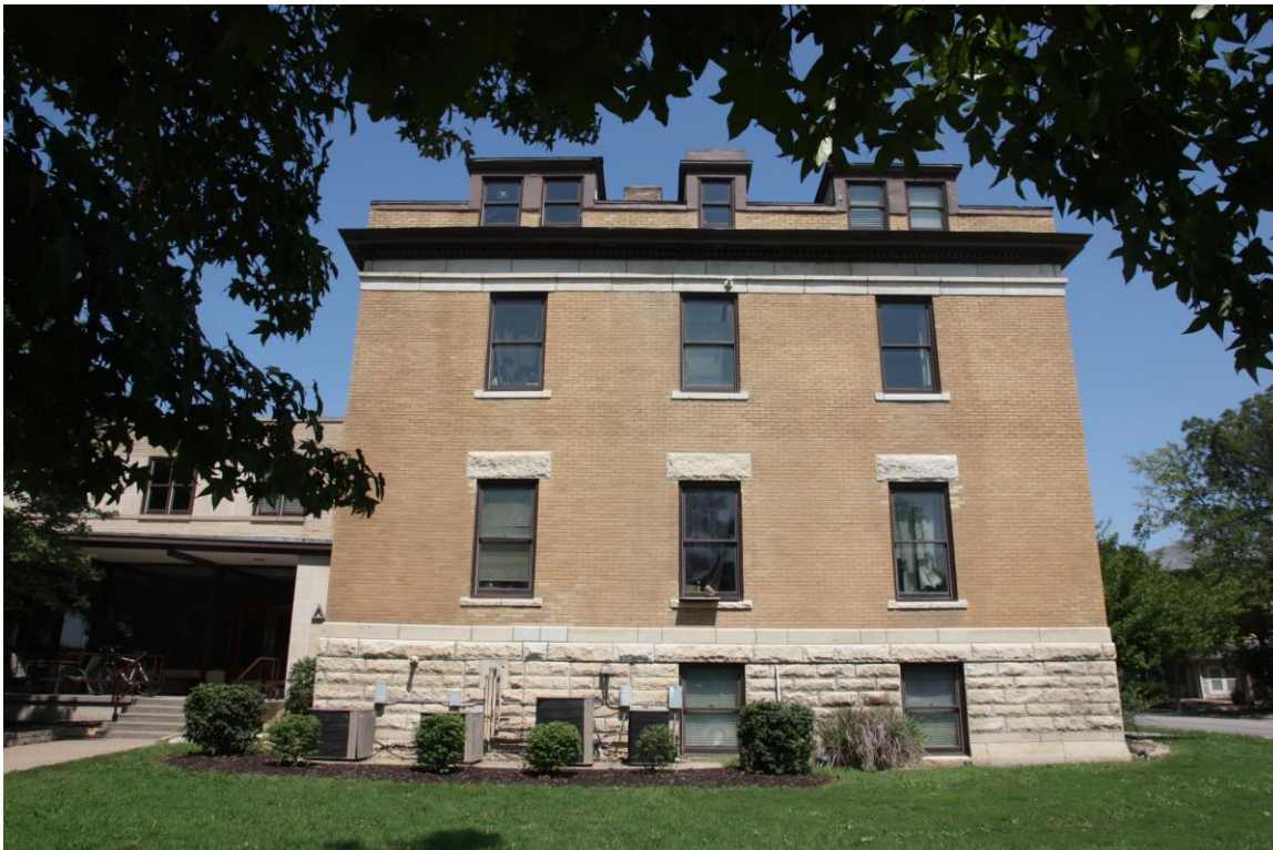
South elevation of original building.
