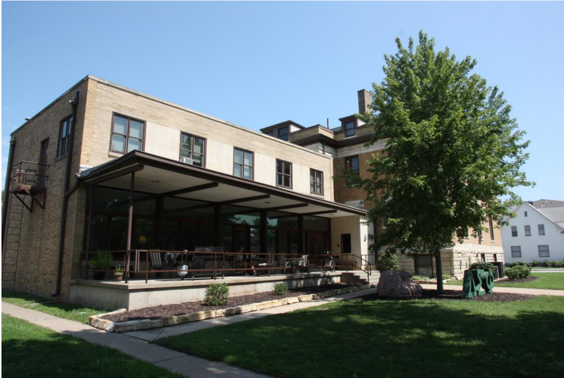
West & south elevation from southwest.
