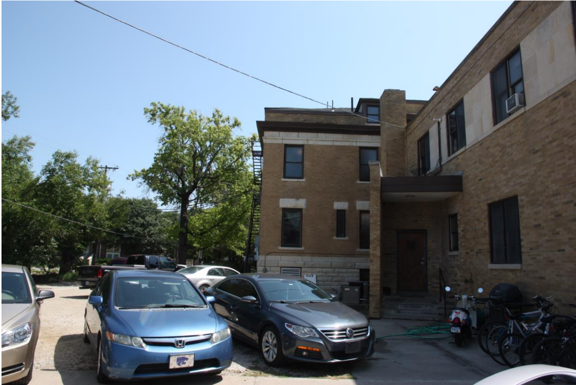
West elevation, north (original) portion, with 1958 addition to the right.
