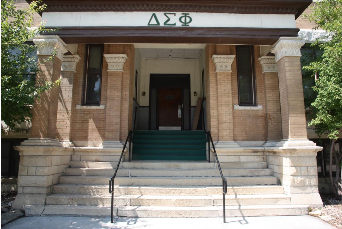
East elevation of entry to original building.
