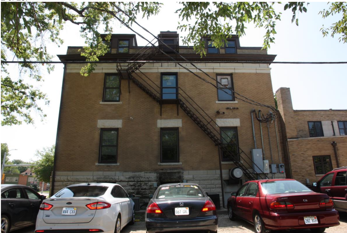
North elevation, east (original) portion.
