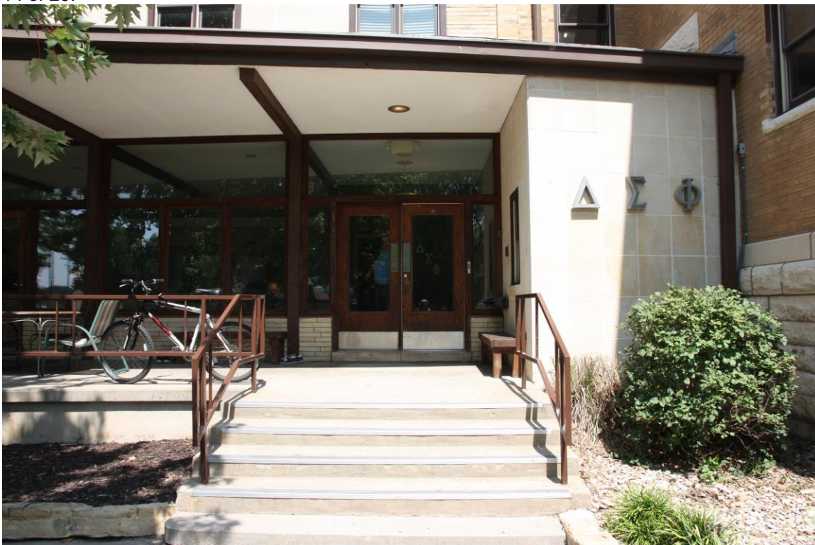
South elevation of entry to 1958 addition.
