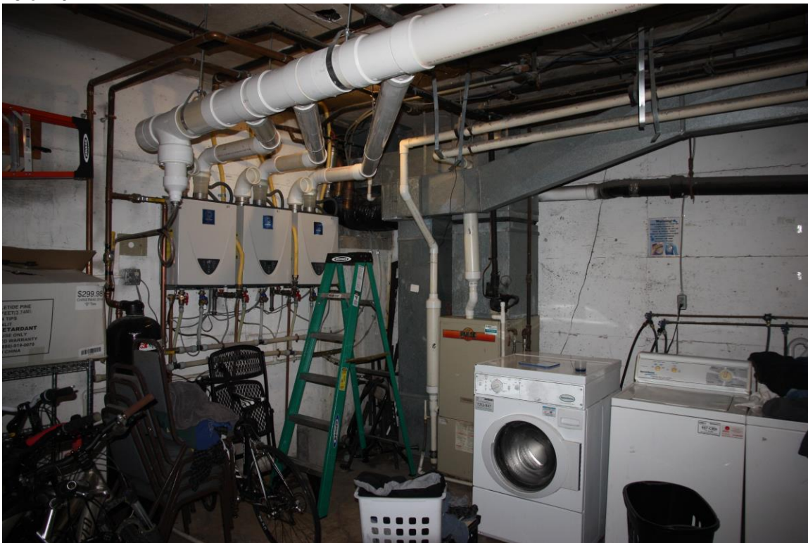
Basement Mechanical Room, looking northwest. Original building.
