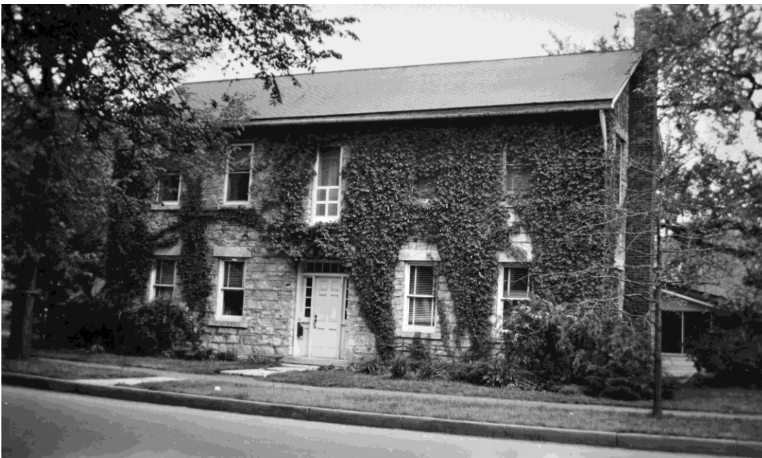
Figure 15 - Undated View of Wolf House at 630 Fremont after 1906 remodel with new windows,
