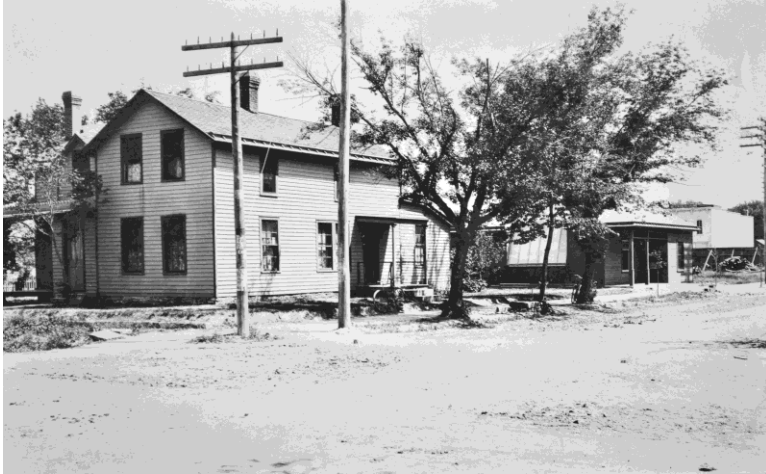
Figure 11 - Looking SE on 5 th Street before construction of Courthouse. Moses House can be seen behind the prominent house on right; Wolf Studio on left, ca.1904.
