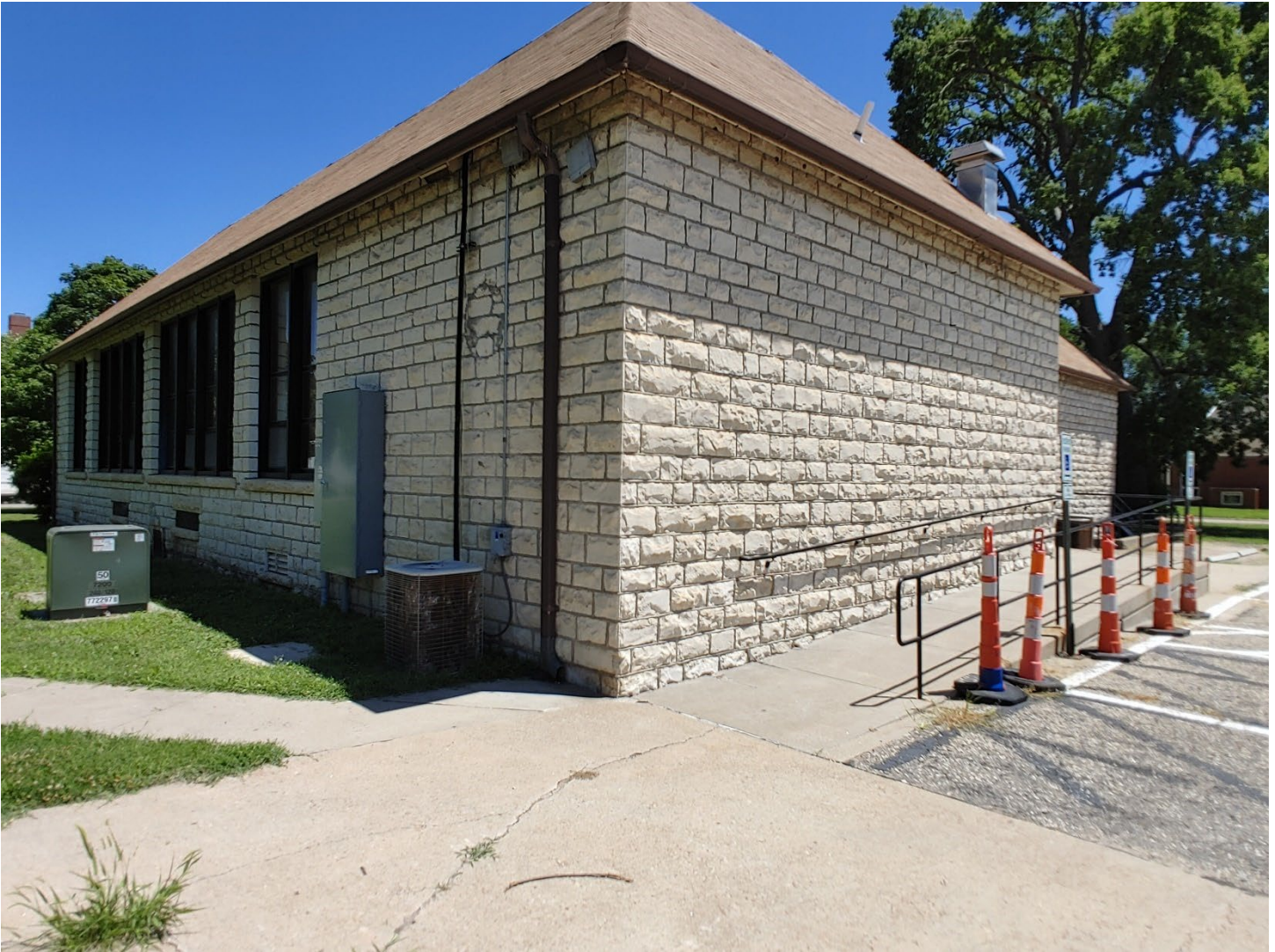
Photo 13: Douglass School, SW corner, camera facing NE
