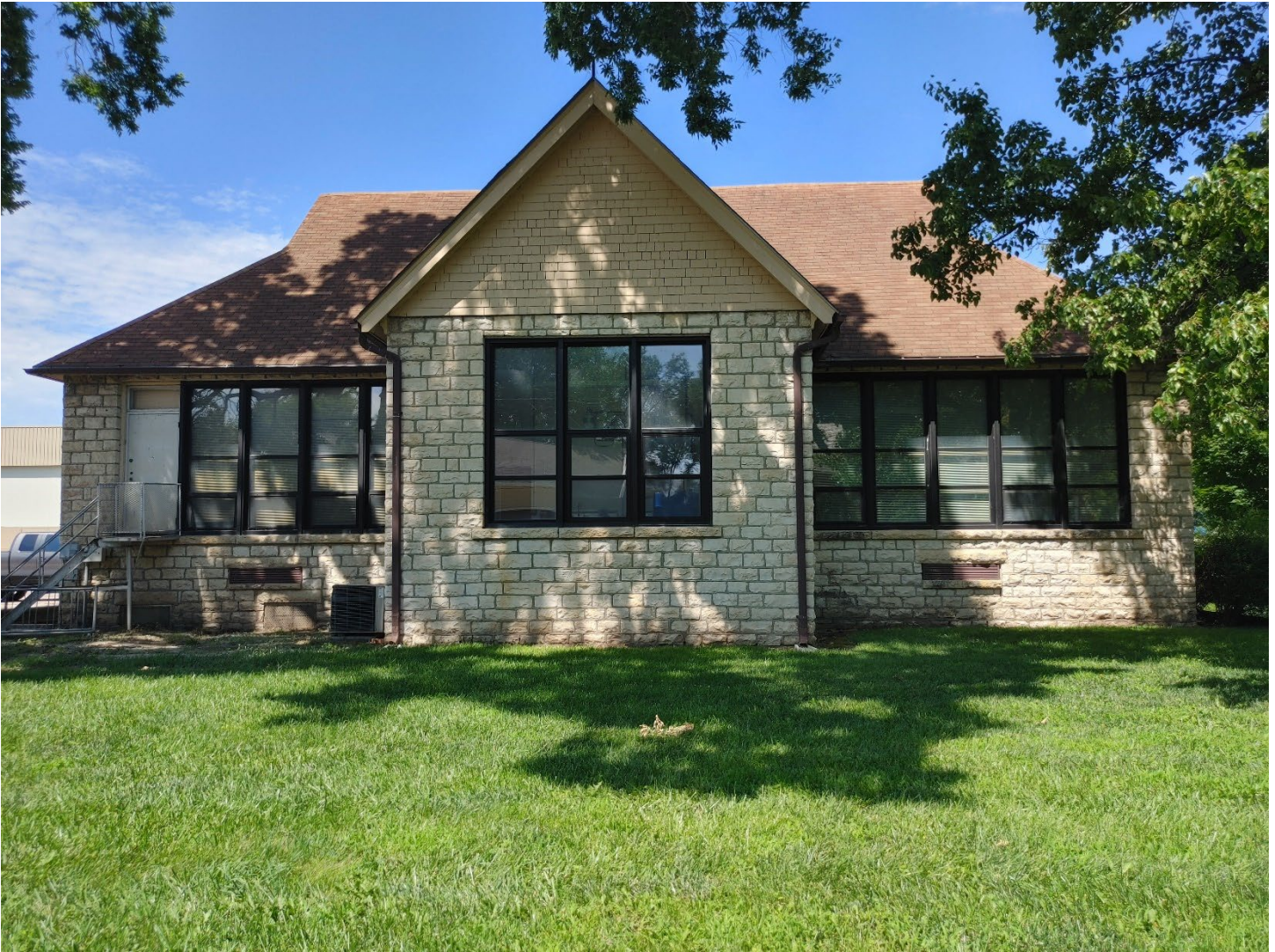
Photo 32: Douglass School, E façade, facing W
