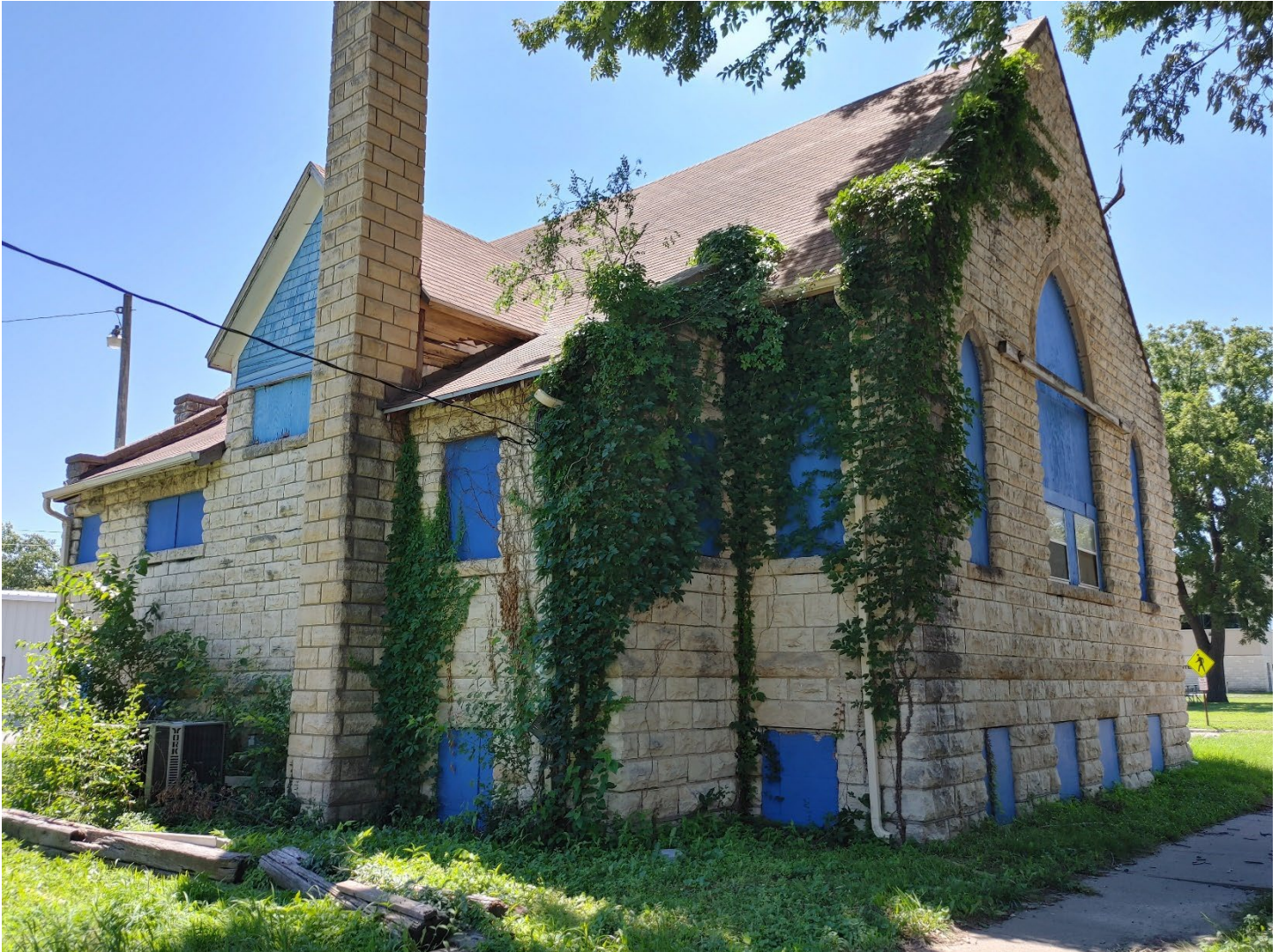
Photo 2: Shepard Chapel, NW corner, camera facing SE
