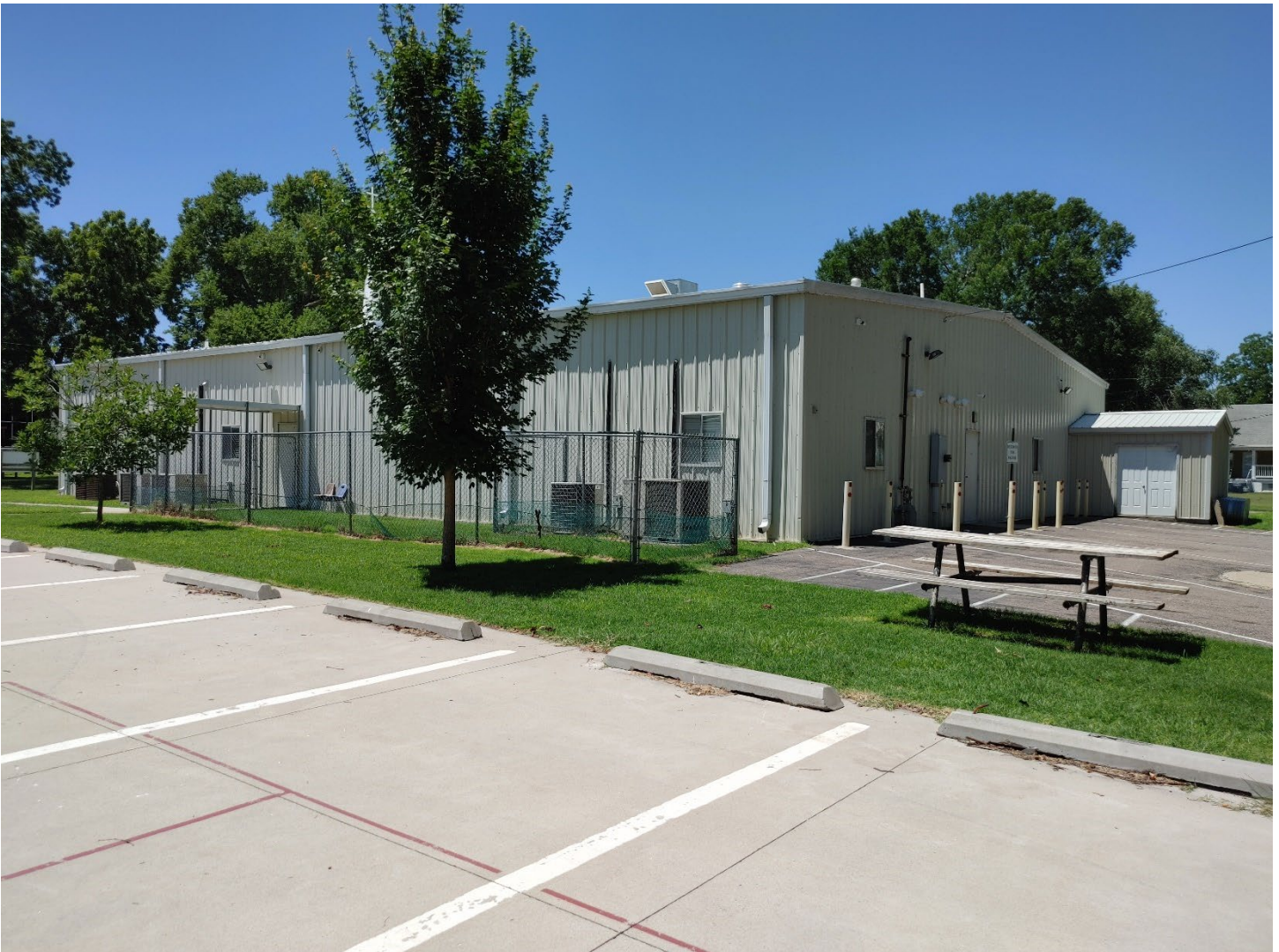
Photo 6: Mt Zion, NE corner, camera facing SW
