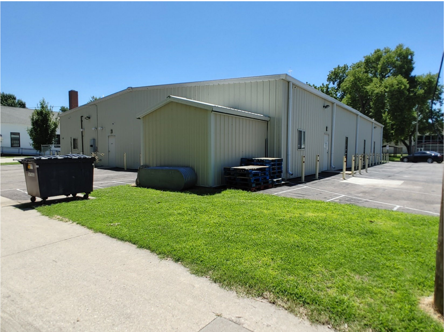
Photo 5: Mt Zion, NW corner, camera facing SE
