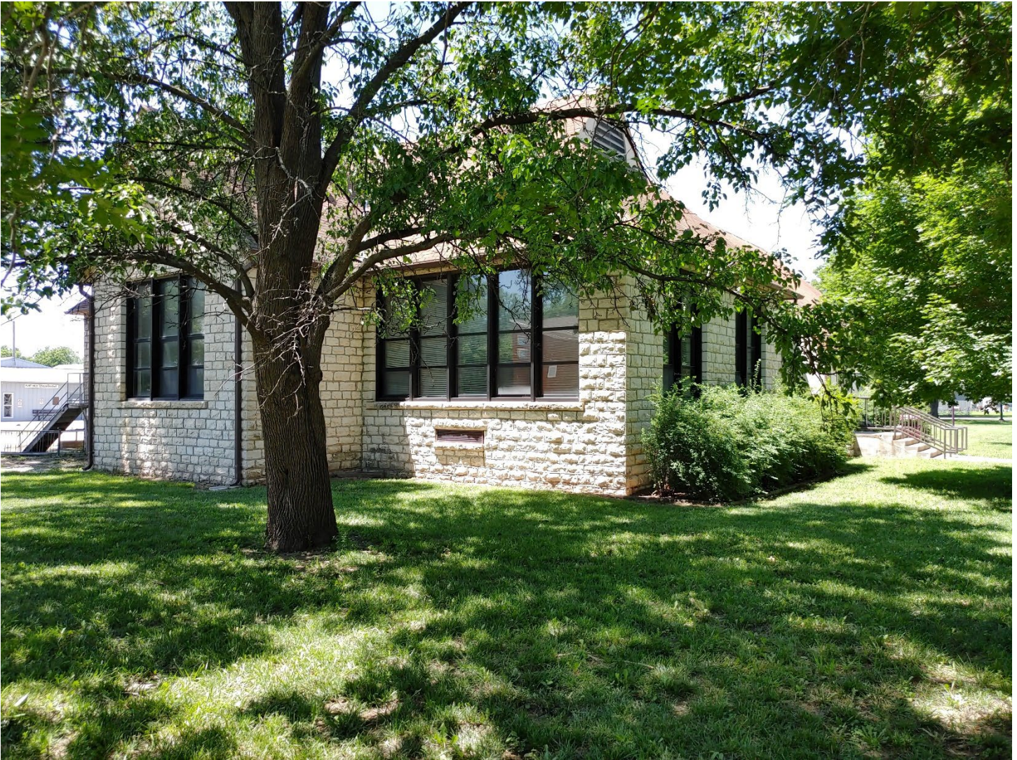
Photo 11: Douglass School, NE corner, camera facing SW
