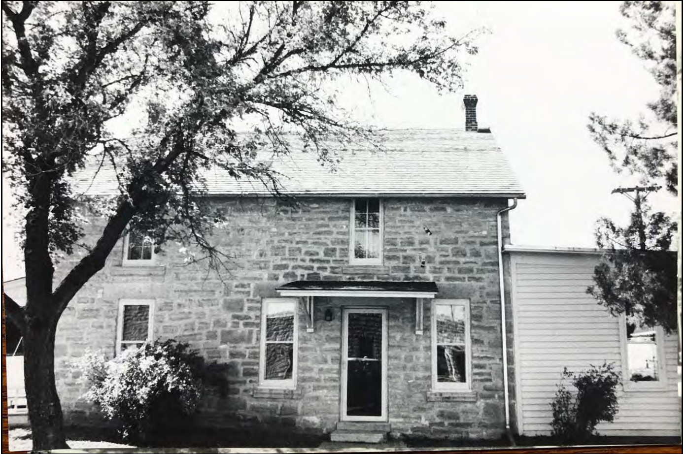
View of east elevation of Gernon House, 1981. Source: Russell County Historical Society .
