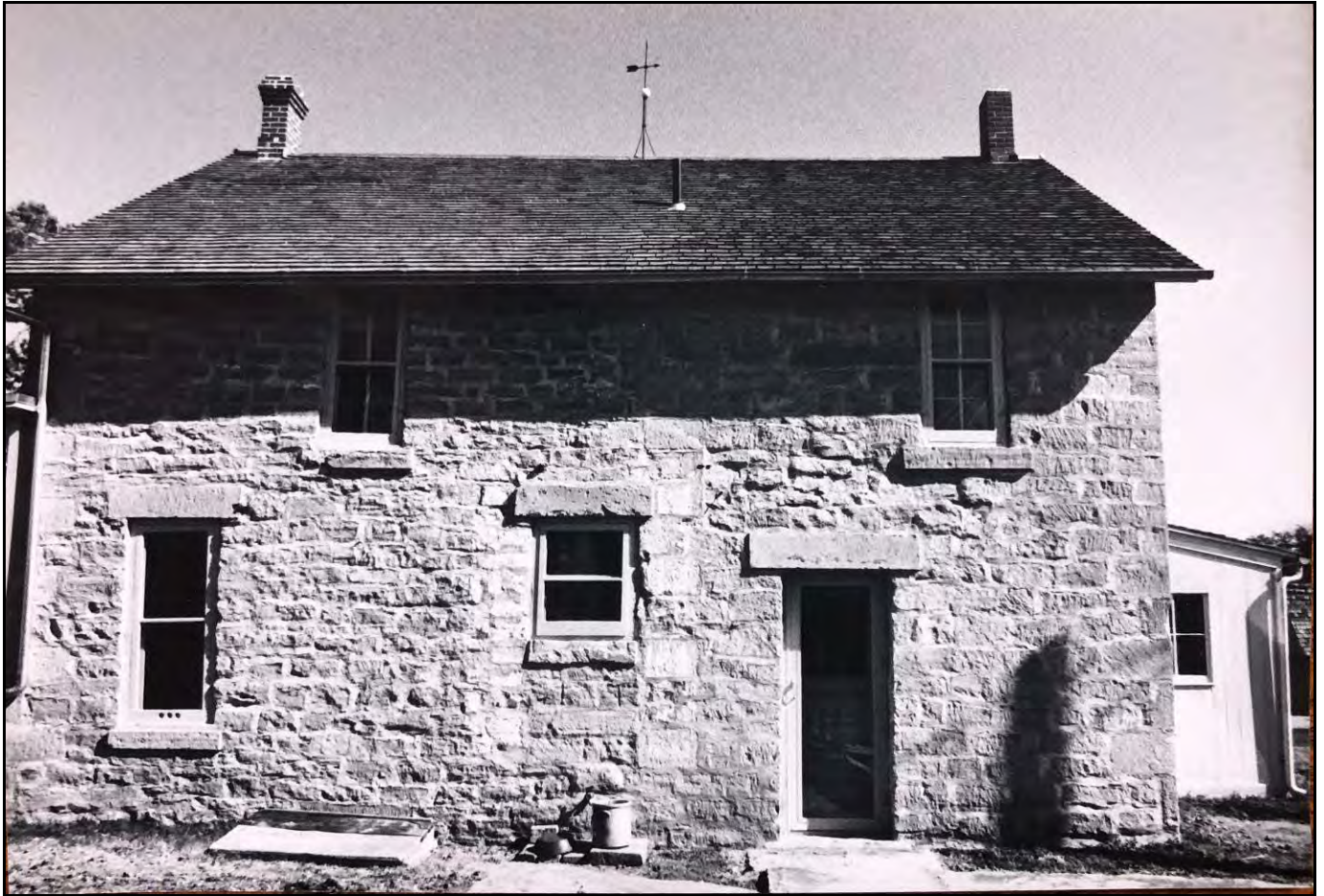
View of west elevation of Gernon House, 1981, after renovation. Photo shows the west elevation after the entrance at the center was removed and replaced with a window. The original side entrance was restored. Source: Russell County Historical Society .
