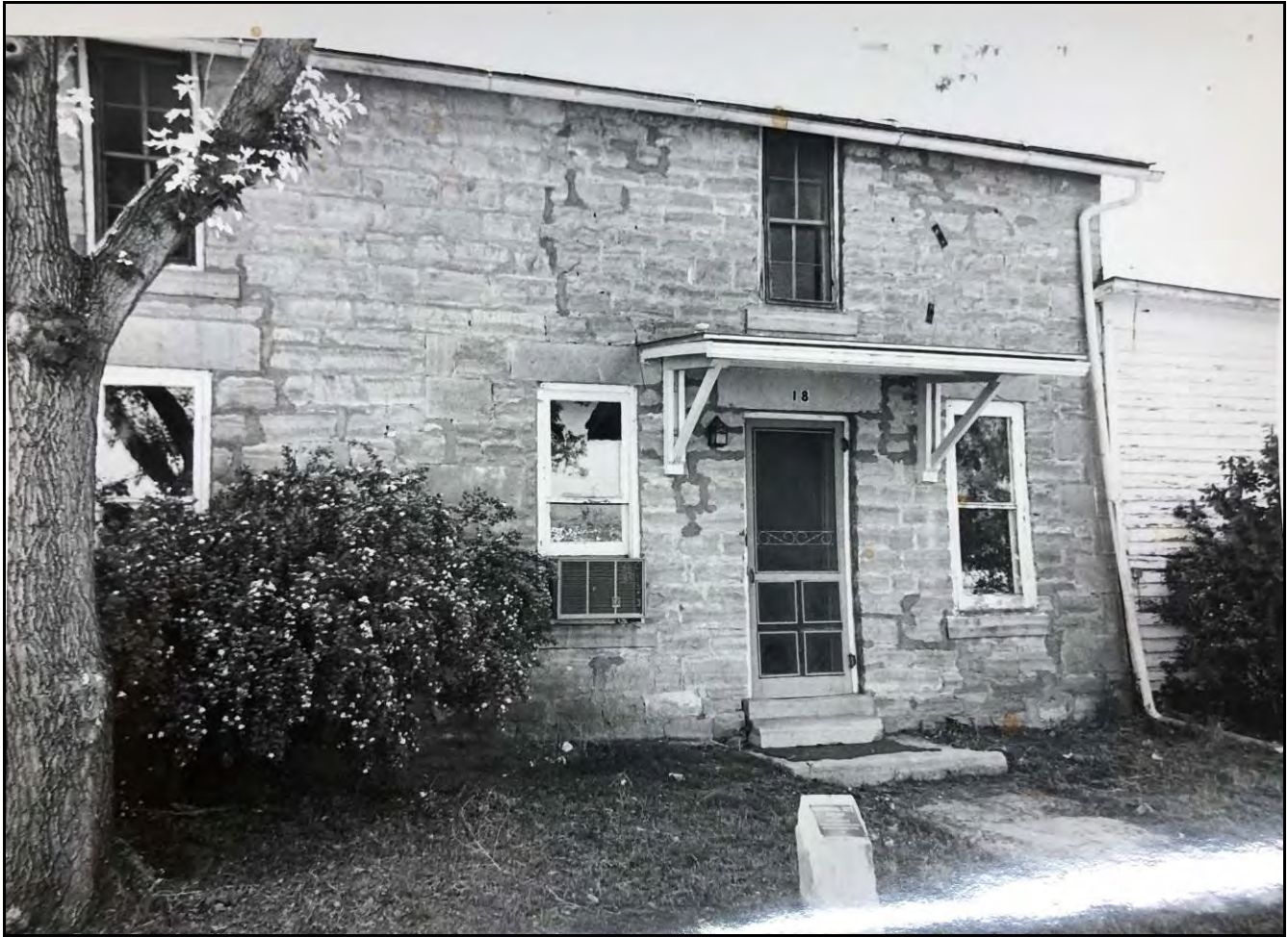
View of east elevation of the Gernon House, 1981. Source: Russell County Historical Society .
