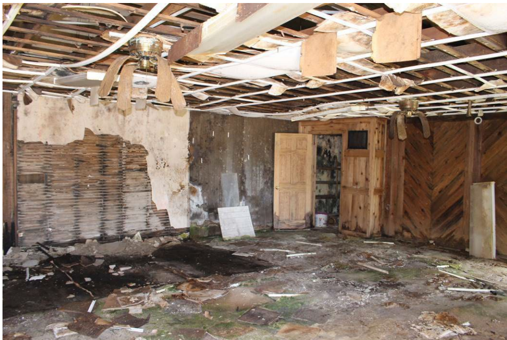
Photo 9 Interior, first floor of the south half of the building
