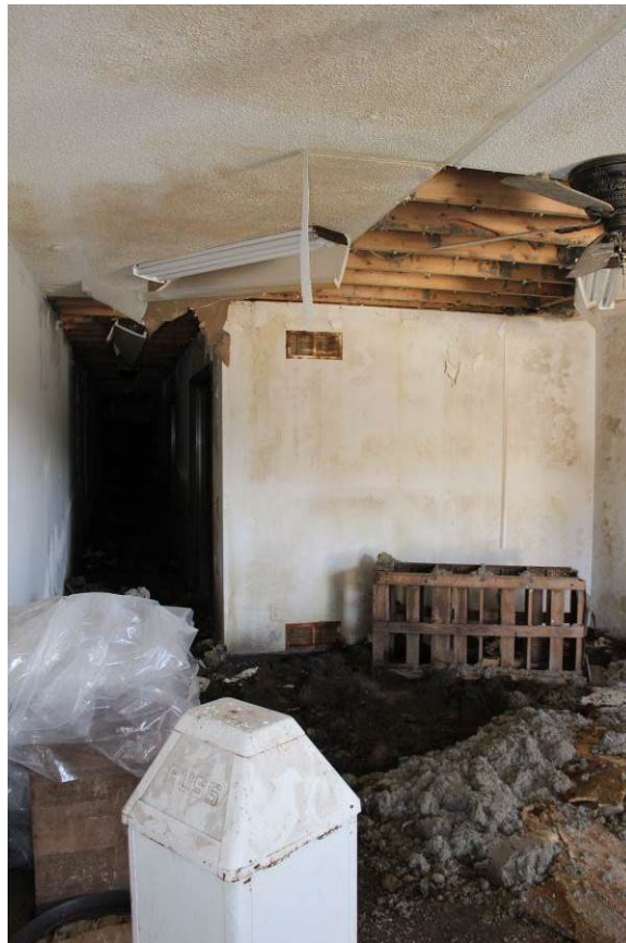
Photo 11 Interior, first floor of the north half of the building
