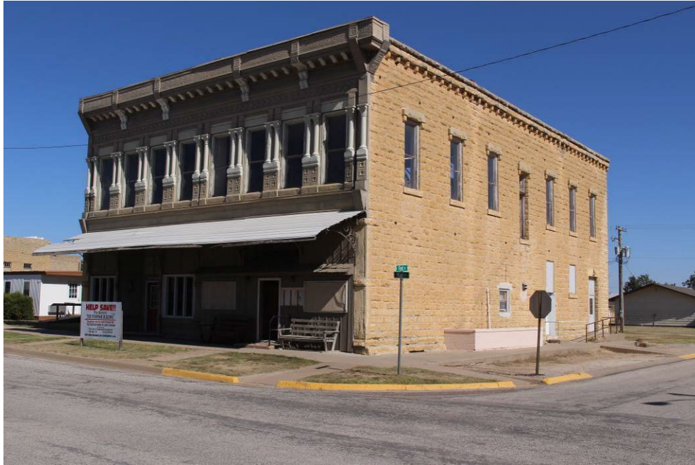
Photo 2 West and south elevations
