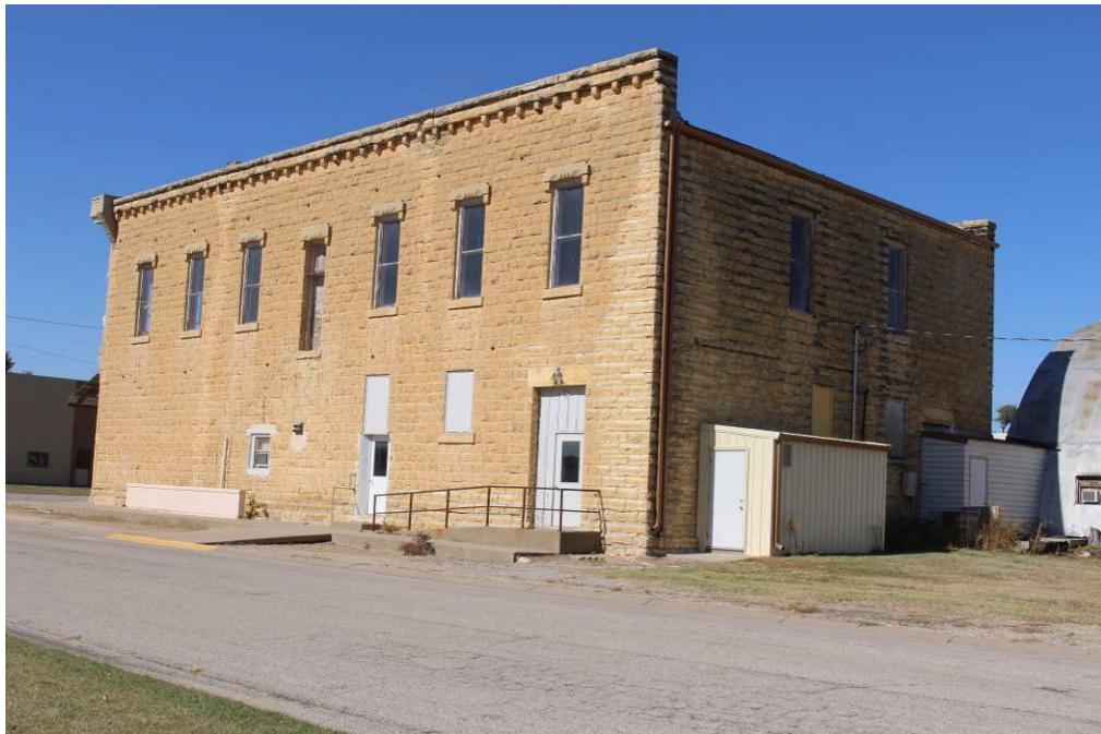
Photo 5 South and east elevations
