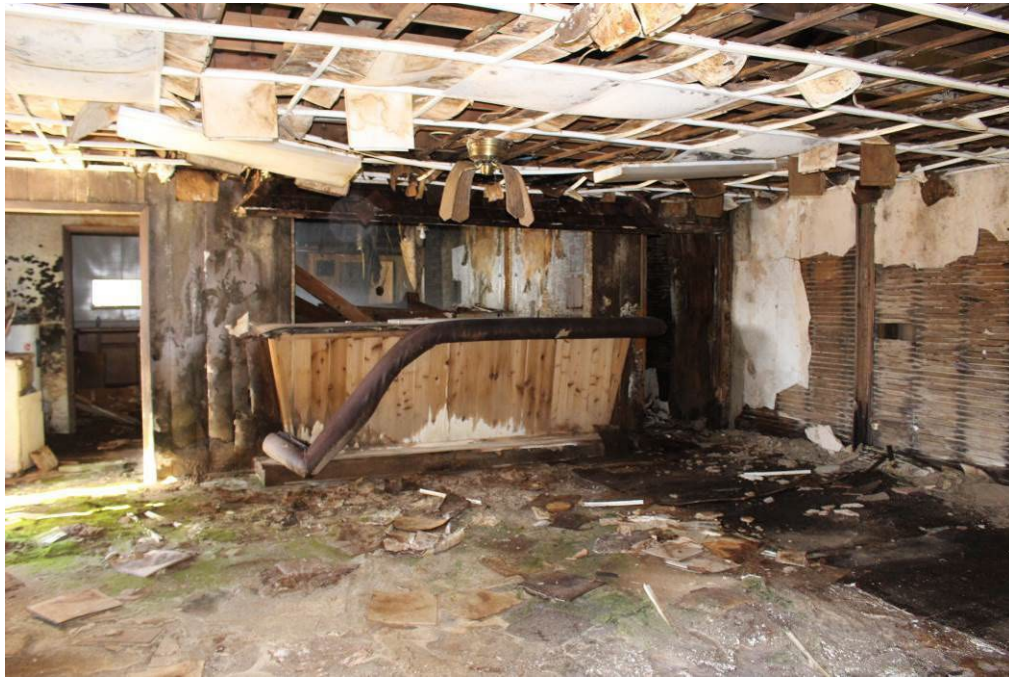
Photo 10 Interior first floor of the south half of the building
