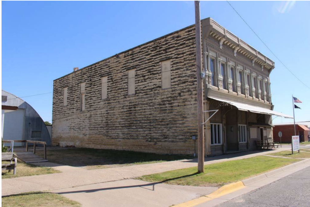
Photo 7 North and west elevations
