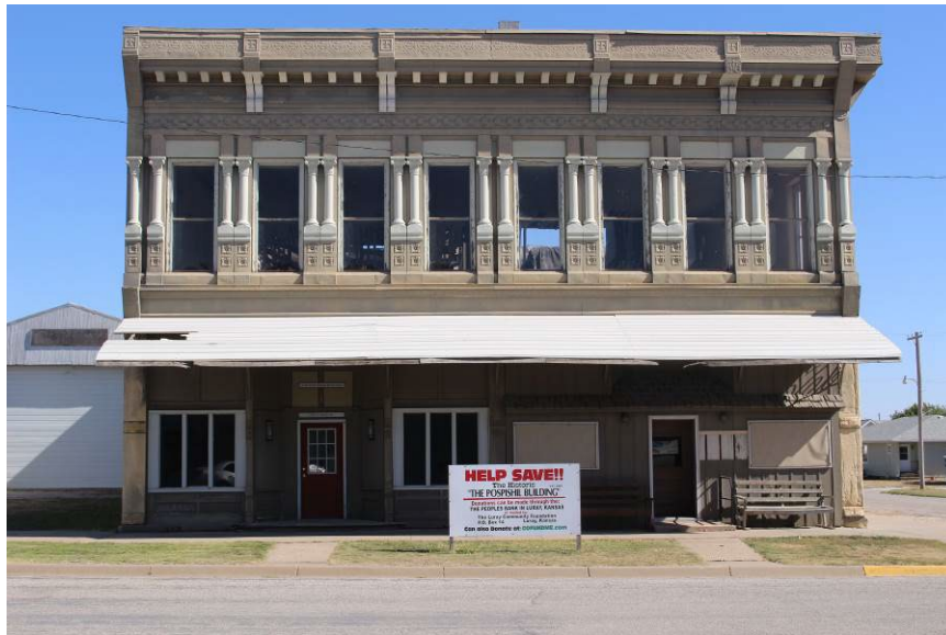
Figure 2 West elevation and the Meskers metal façade
