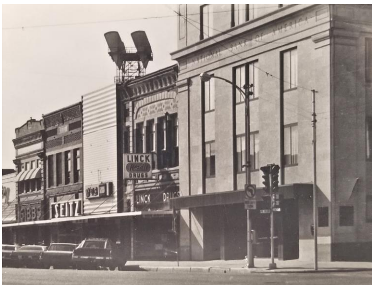
Figure 8 - ca. 1975 View of southeast corner of S. Santa Fe and W. Iron with Teague Nelson Building south/left of corner bank building with metal siding over upper facade of 106. Source: Campbell Room Collection, Salina Public Library.
