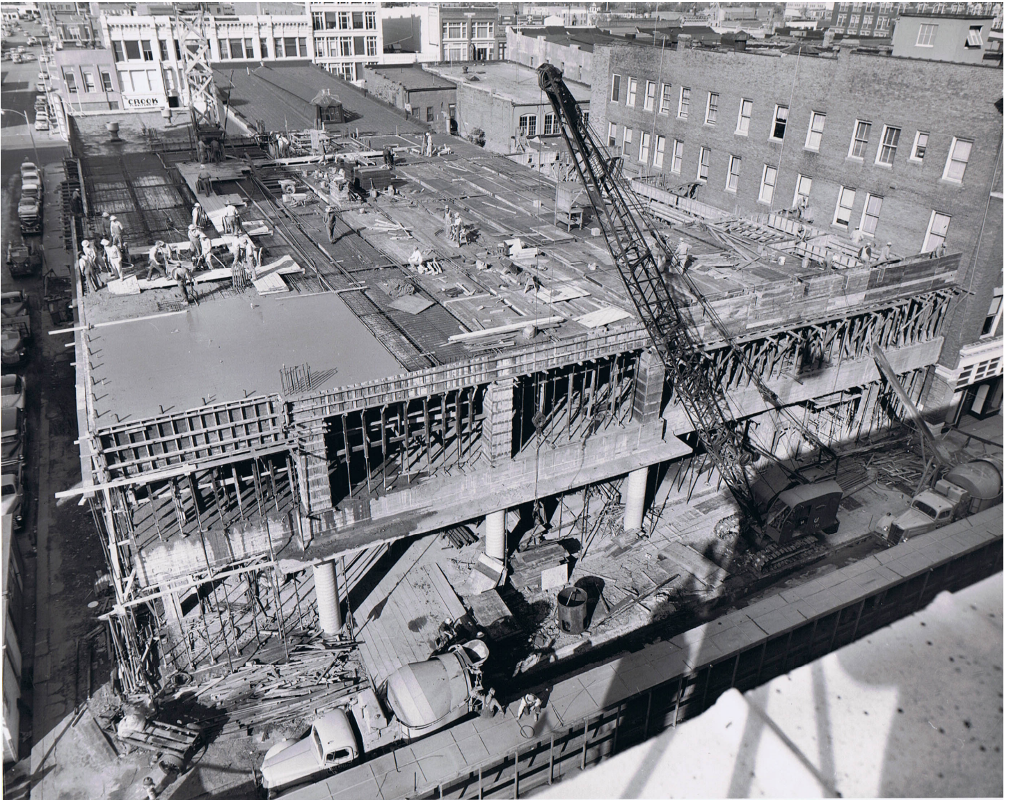
Kansas Gas & Electric Company, 1953 Source: Files, GLMV Architects, Wichita
