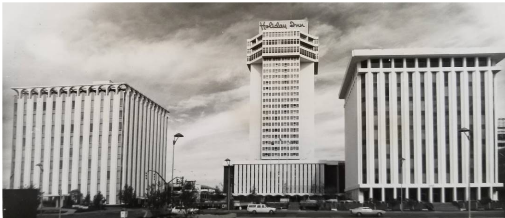
Figure 1 - ca.1971 View of Garvey Center – the R.H. Garvey Building on left, Holiday Inn in center, and O.W. Garvey Building on right. (Platt & Associates, Architects Photo Book, archives of Platt, Adams,
