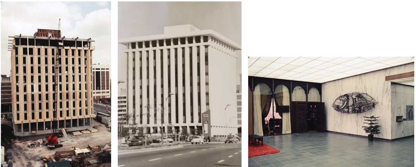
Figure 7 – Left: ca.1969 view of O.W. Garvey Building during construction; Center: ca.1971 view of O.W. Garvey Building from the southeast on Water Street; Right: ca.1971 view of the lobby with metal wall sculpture (Platt & Associates, Architects photo book and slides, archives of Platt, Adams, Bradley and Associates, Architects, Wichita).
