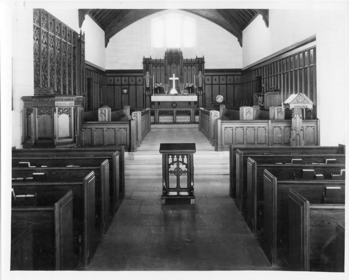
Figure 10: The chancel in the late 1930s. The woodwork has been installed but the rood beam and the stained glass window over the altar have yet to be added.
