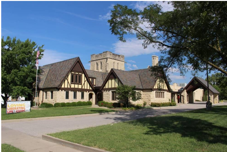
Figure 4: The new music room addition dates from the 2000s but mirrors the architecture of the office wing. The porte-cochere in the back marks the entrance to the lobby.
