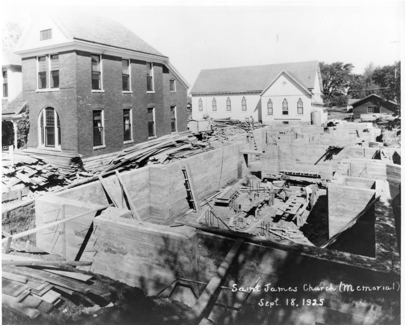
Figure 16: Construction taking place. This view is looking north from Douglas Avenue.
