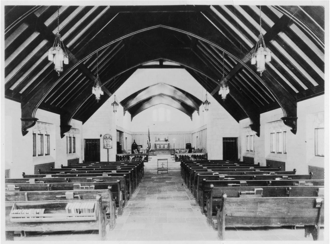
Figure 6: The nave soon after construction was finished. The pews and furnishings from the former St. Stephens are still being used. The chancel walls have fabric instead of the later woodwork. The stained glass windows will be installed decades later.
