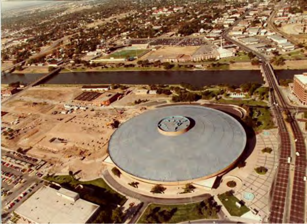
Figure 31 – Aerial Photo of Century II with Foundation of Bob Brown Expo Center, 1985 – Photographer Unknown, WICHITA PHOTO ARCHIVE, wicitaphotos.org, Archives of the Wichita Chamber of Commerce, Wichita State University Library, Special Collections, Date Digital 2003
