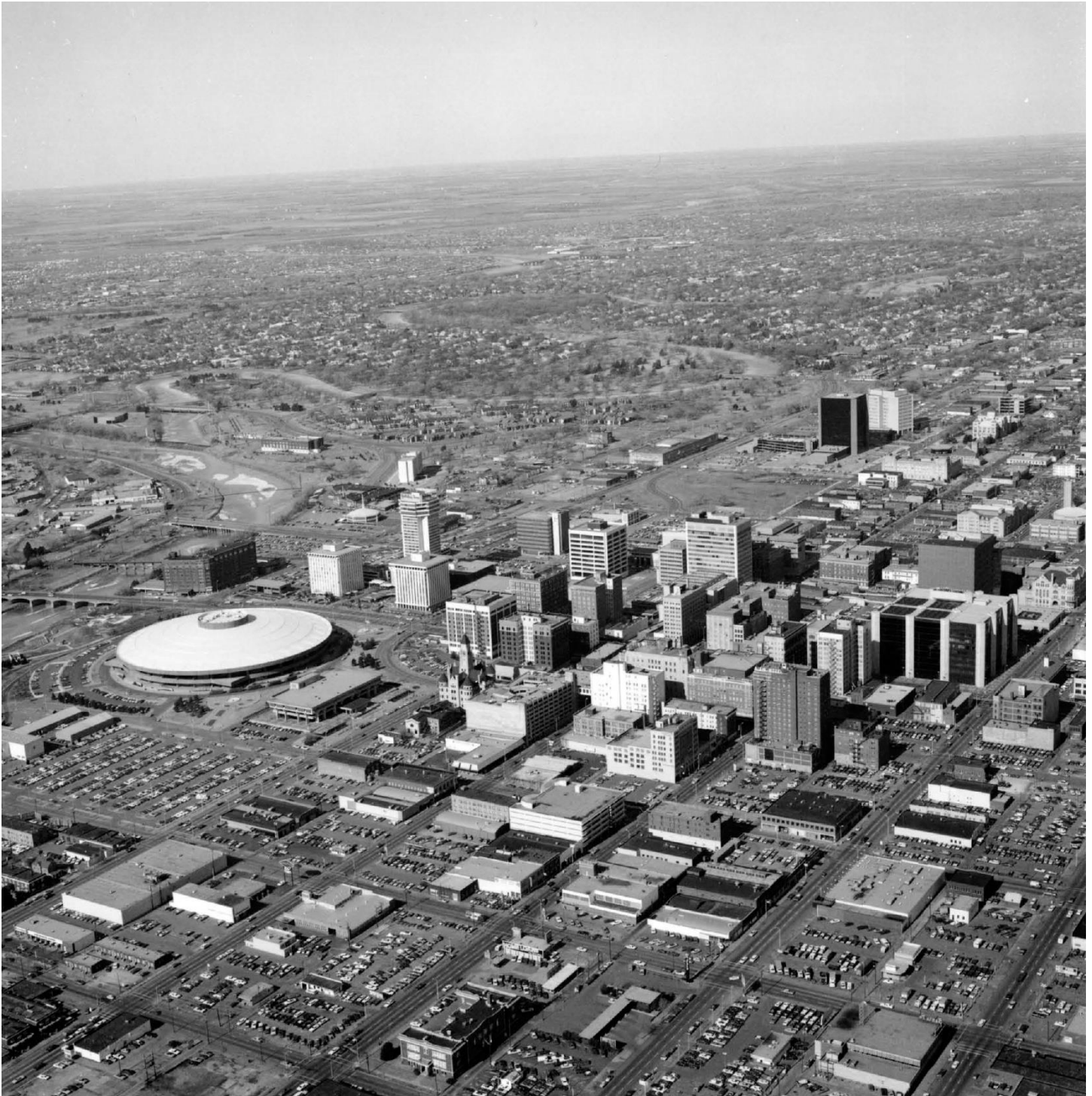
Figure 30 – Aerial Photo Century II, Looking Northwest, Circa 1976 – Photographer, Tom Doan, WICHITA PHOTO ARCHIVE, wichitaphotos.org, Archives of the Wichita Chamber of Commerce, Wichita State University Library, Special Collections, Date Digital 2003
