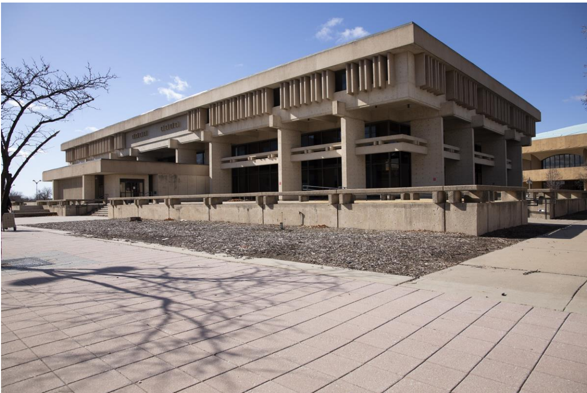
Photo #2 – Exterior View from Northeast
