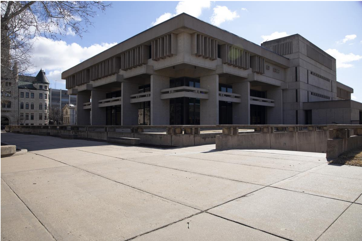
Photo #4 – Exterior View from Northwest
