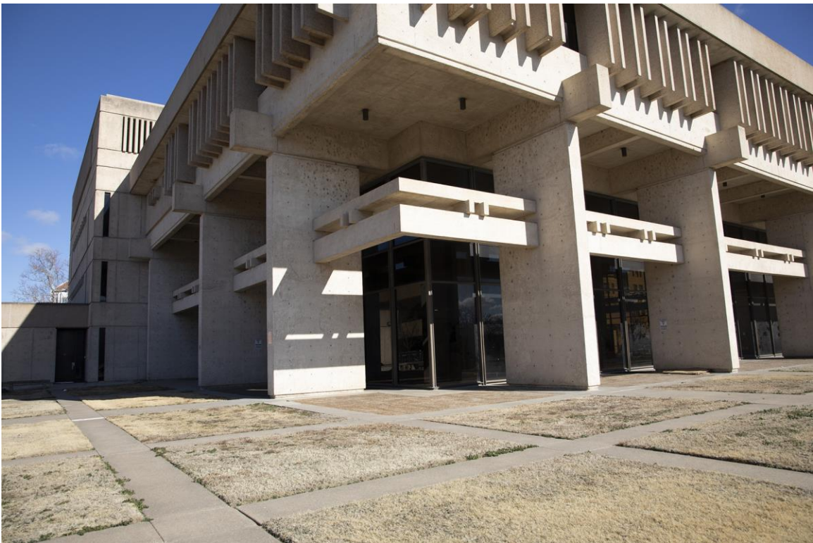
Photo #6 – Exterior View from Southwest
