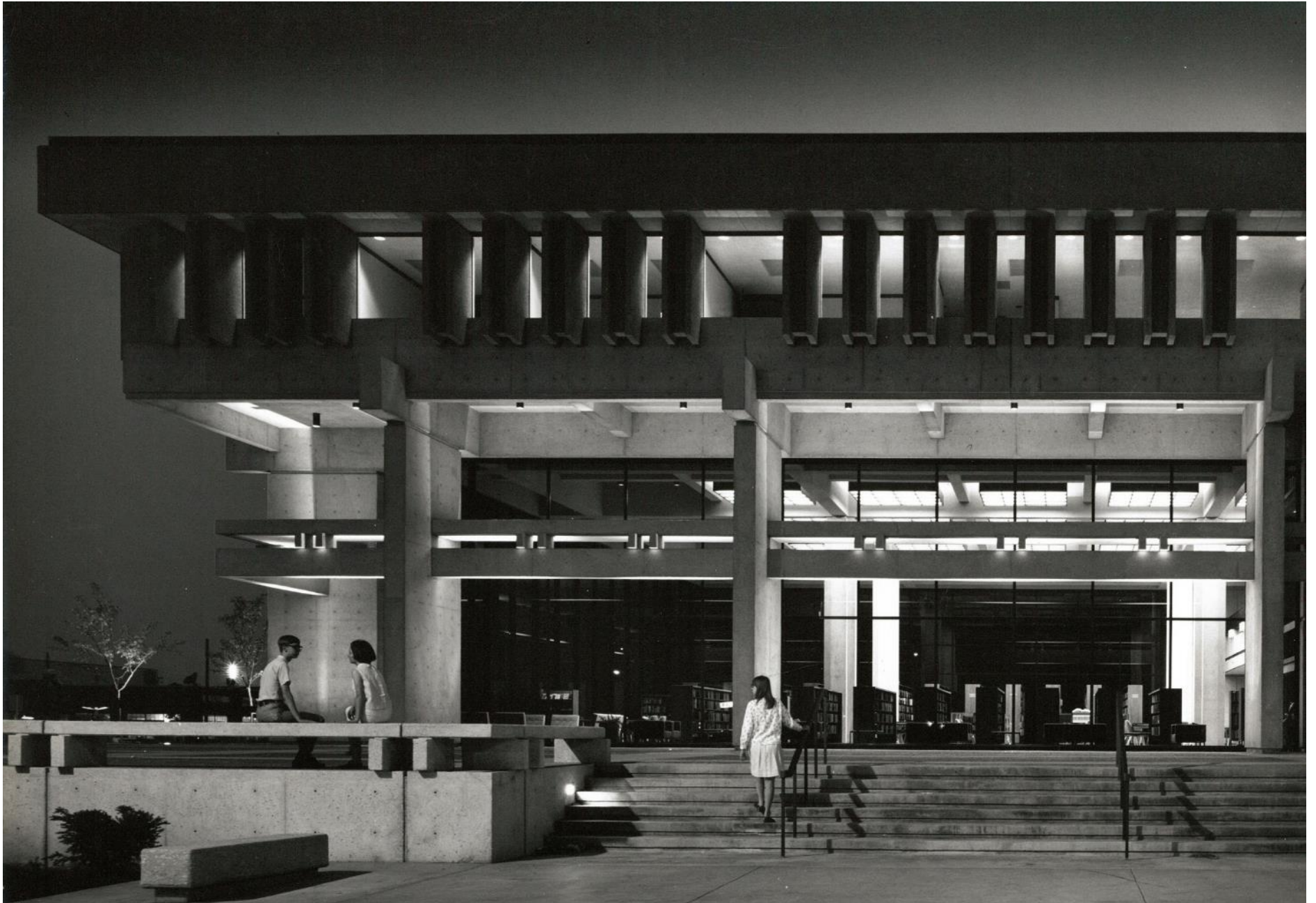
Figure 24 – Photo of Partial Front Façade from East at Dusk – Wichita Public Library of Wichita, Kansas – Photo by Julius Shulman – Taken May 28-30, 1967 – Architects, Schaefer Schirmer and Eflin, AIA; Scan of photo courtesy of SJCF Architecture Archives Accessed 2/14/2020 & © J. Paul Getty Trust. Getty Research Institute, Los Angeles (2004.R.10) Job #4248 – Julius Shulman, 1910-2009, was an active architectural photographer from 1936-1986.
