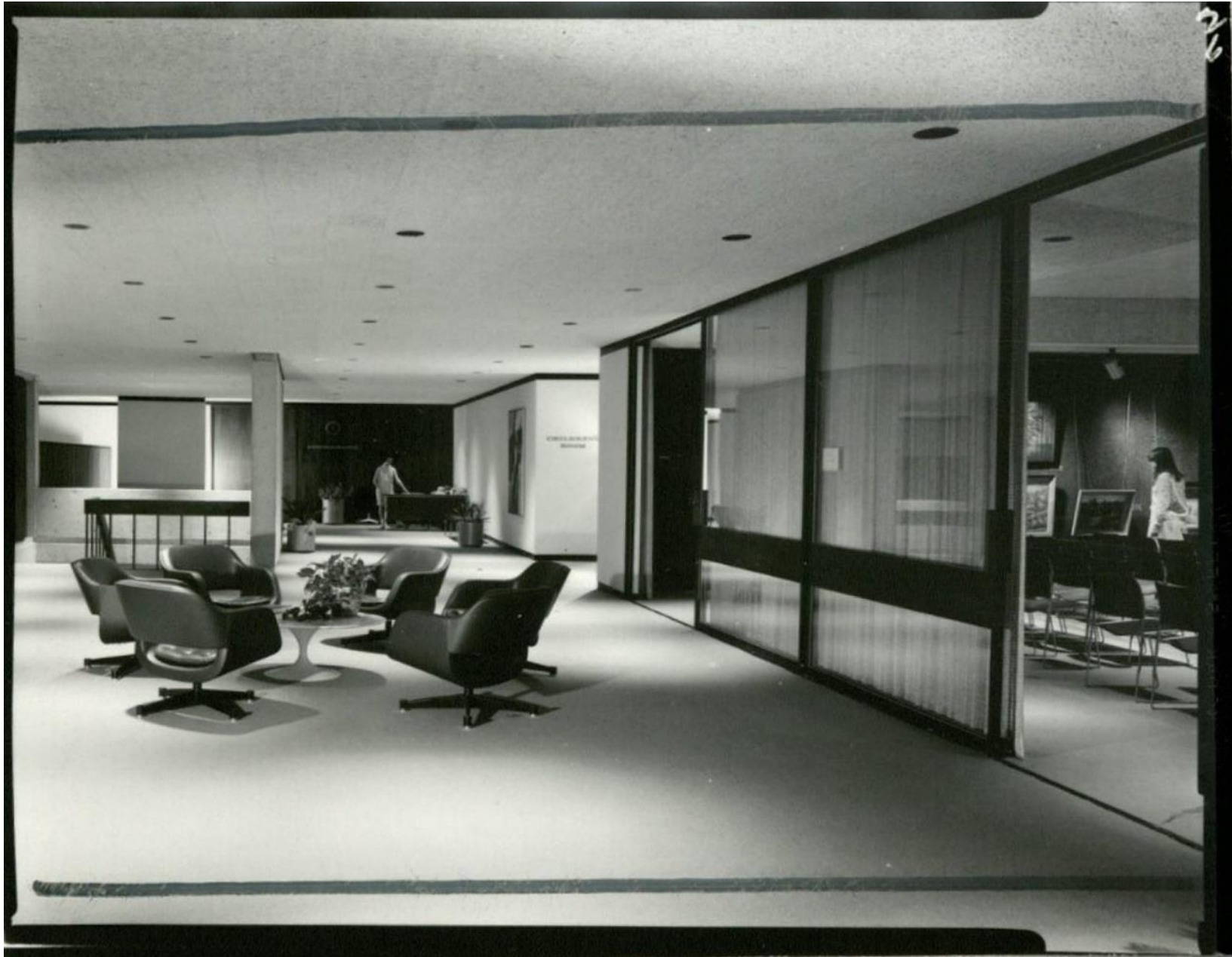
Figure 33 – Contact Print of Upper Level Lobby (Notice the 2 horizontal crop lines by Julius Shulman) – Wichita Public Library of Wichita, Kansas – Photo by Julius Shulman – Taken May 28-30, 1967 – Architects, Schaefer Schirmer and Eflin, AIA; Scan of photo courtesy of Julius Shulman Archive © J. Paul Getty Trust. Getty Research Institute, Los Angeles (2004.R.10) Job #4248 – Julius Shulman, 1910-2009, was an active architectural photographer from 1936-1986.
