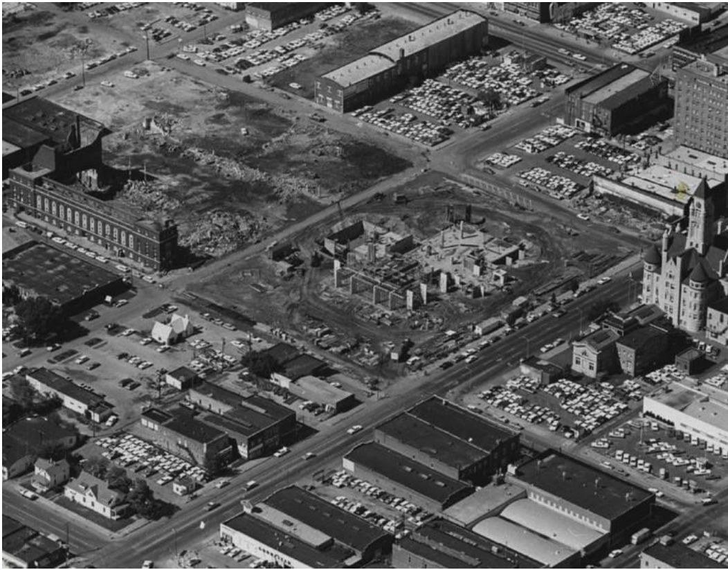
Figure 39 – Aerial Wichita Public Library Construction Photo (Center), Demolition of Forum (Upper Left) – Wichita, Kansas – Architects, Schaefer Schirmer and Eflin, AIA 1965; Photographer Unknown, Image Courtesy of Wichita Eagle
