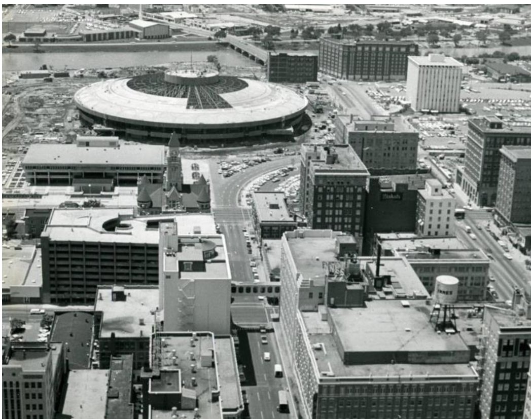
Figure 42 – Aerial Century II Construction Photo with Wichita Public Library, Wichita, Kansas, No Date – Architects, Schaefer Schirmer and Eflin, AIA; Photographer Unknown, Image Courtesy of Wichita Eagle
