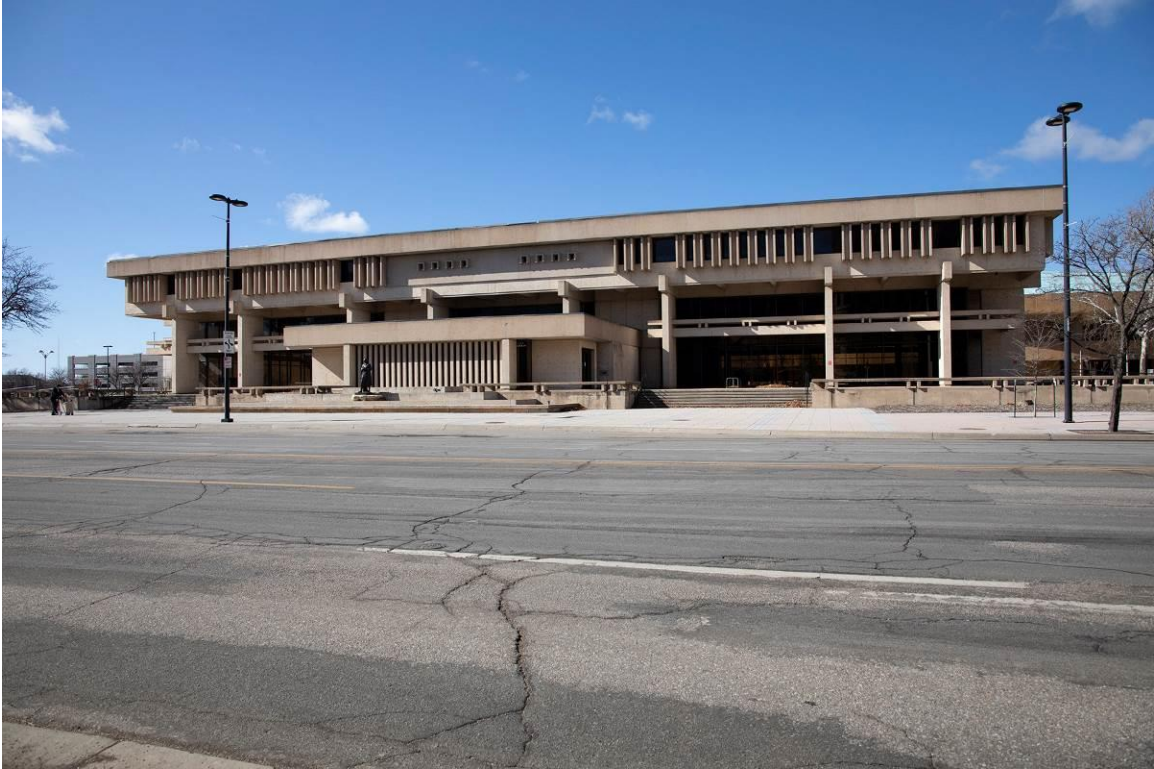
Photo #1 – Exterior View of Front Elevation from East on Main Street
