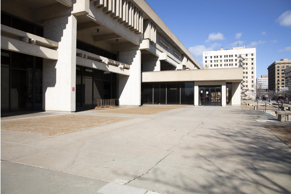
Photo #7 – Exterior View of Entry Pavilion from South
