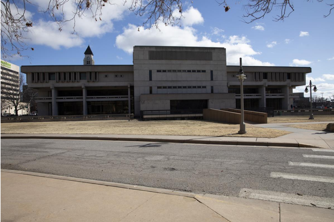
Photo #5 – Exterior View of Back Elevation from West on South Cancun Street
