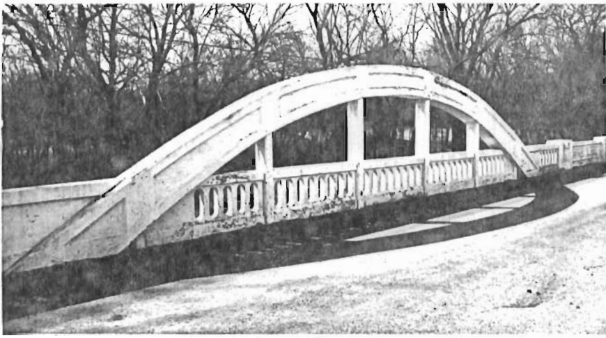
Blacksmith Creek Bridge South arch looking southwest.
