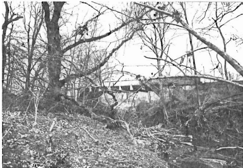
Blacksmith Creek Bridge South side looking northwest.
