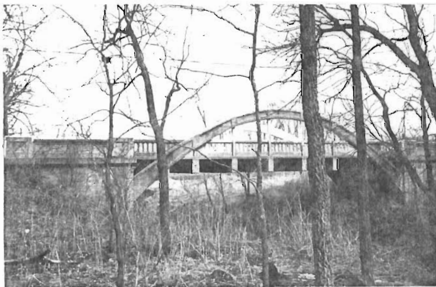
Blacksmith Creek Bridge South side looking northeast.
