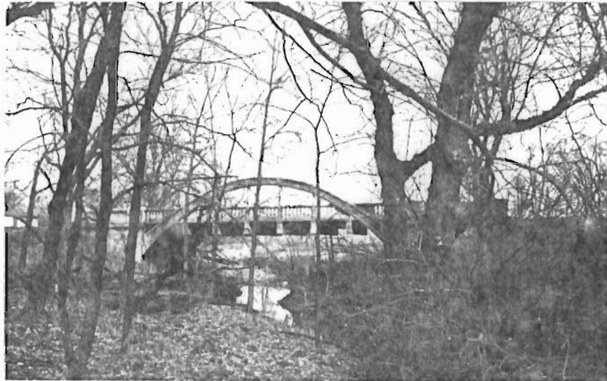
Blacksmith Creek Bridge South side looking north.
