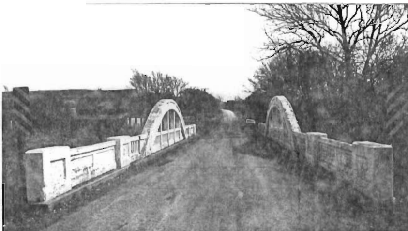
Blacksmith Creek Bridge West approach looking east.
