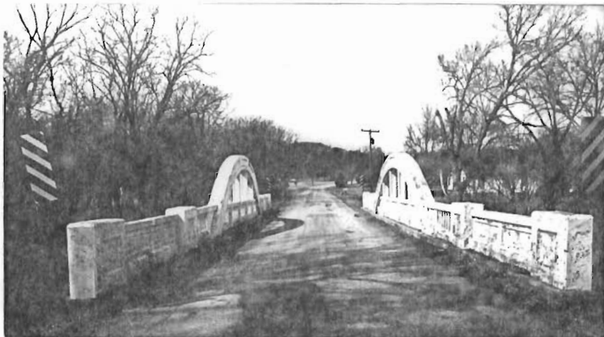
Blacksmith Creek Bridge East approach looking west.
