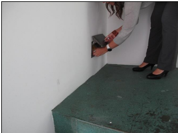
Figure 5: Mail slot at stair landing (KSHS, May 2017).
