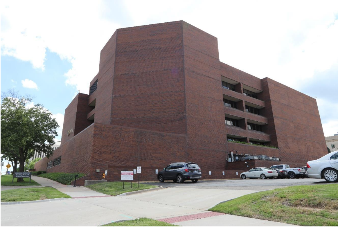
Figure 5. Oblique view of north elevation. [STRATA, 2022]
