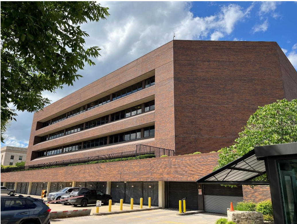
Figure 4. Oblique view of south elevation. [Quinn Evans, 2022]
