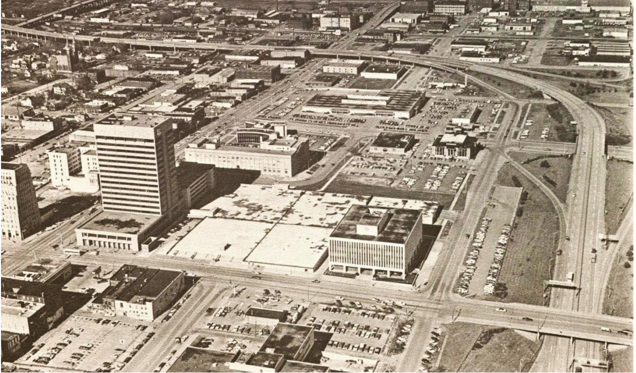
Figure 30. Ca. 1973 view of the partially constructed Townsite Plaza. At center-right is the site of the future Frank Carlson Federal Building and US Courthouse at that time in use as a parking lot. [Urban Renewal Agency of the City of Topeka. Annual Report (Topeka, Kansas, 1973)]
