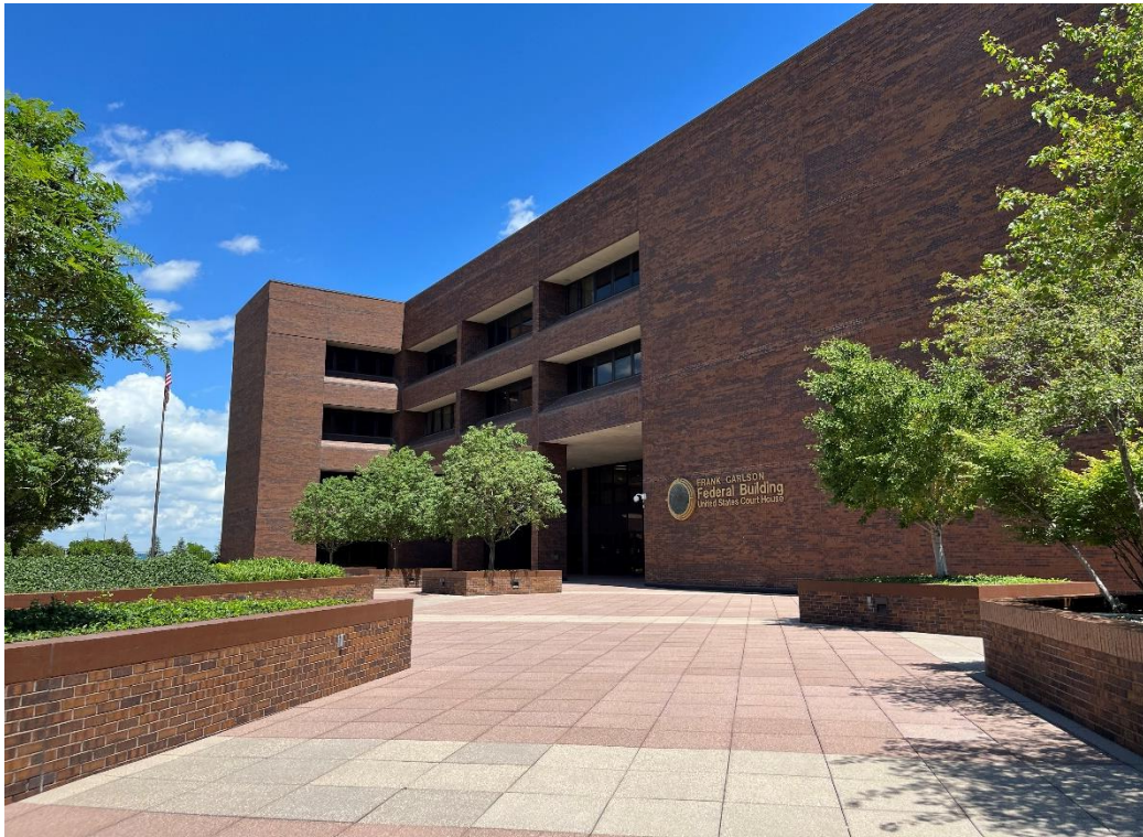
Figure 1. Oblique view of front façade and front section of plaza, looking northeast. [Quinn Evans, 2022]
