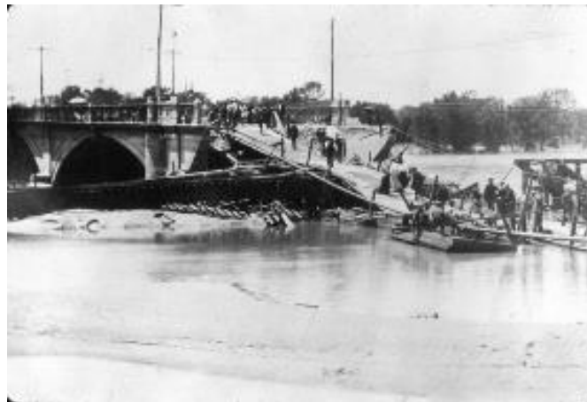
1965 Melan Bridge Collapse (July 2, 1965)
