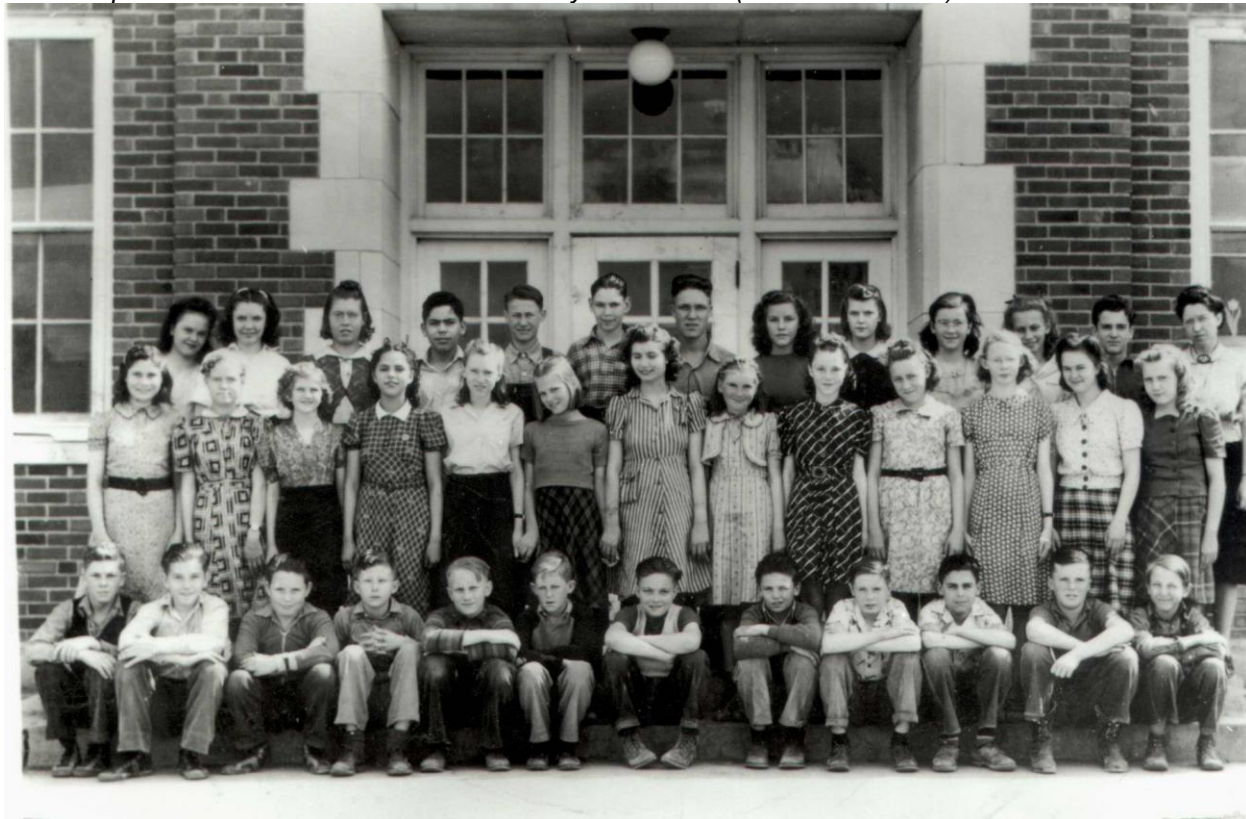
Group of students at front entrance of Grant School, 1942 (illustrating original entrance and windows)
