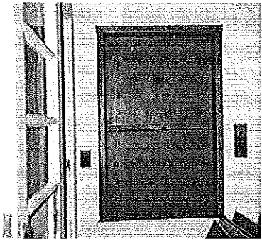
Dumbwaiter, basement, west
