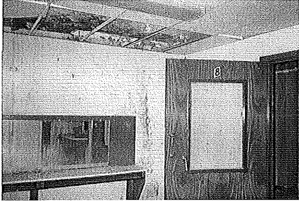
Choir level, Room 8, next to stairway
