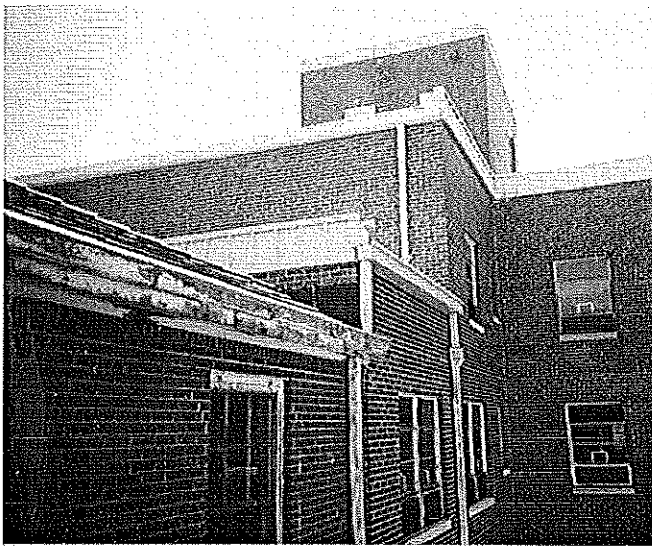
1941 and 1948 Roof Connections, Southeast view
