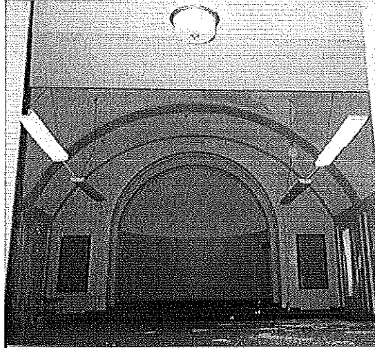
Chapel floor level doorway
