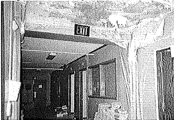
Main Building, Addition Central Hallway
