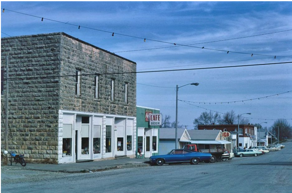
Figure 6 – 1976 View of Pearl Opera House building – note cornice had been removed prior to 1976 (John Margolies, Library of Congress)
