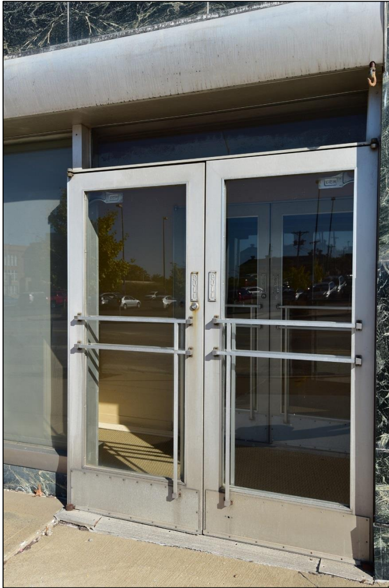
Figure 14. Historic aluminum doors on west façade [Brad Finch, photographer. October 2018].
