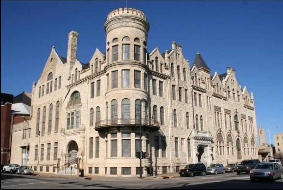
Figure 13. Top: Wichita's 1887-1888 YMCA/Scottish Rite Temple, 332 E. 1 st Street. View looking northwest at south and east facades. 2007. Source: Kansas Historic Resources Inventory, https://khri.kansasgis.org/index.cfm?in=173-5880-00005 (accessed 7 January 2019). Bottom: Marion's 1887 YMCA (not extant). 1907. Source: Kansas Memory, https://www.kansasmemory.org/item/312465 (accessed 7 January 2019).
