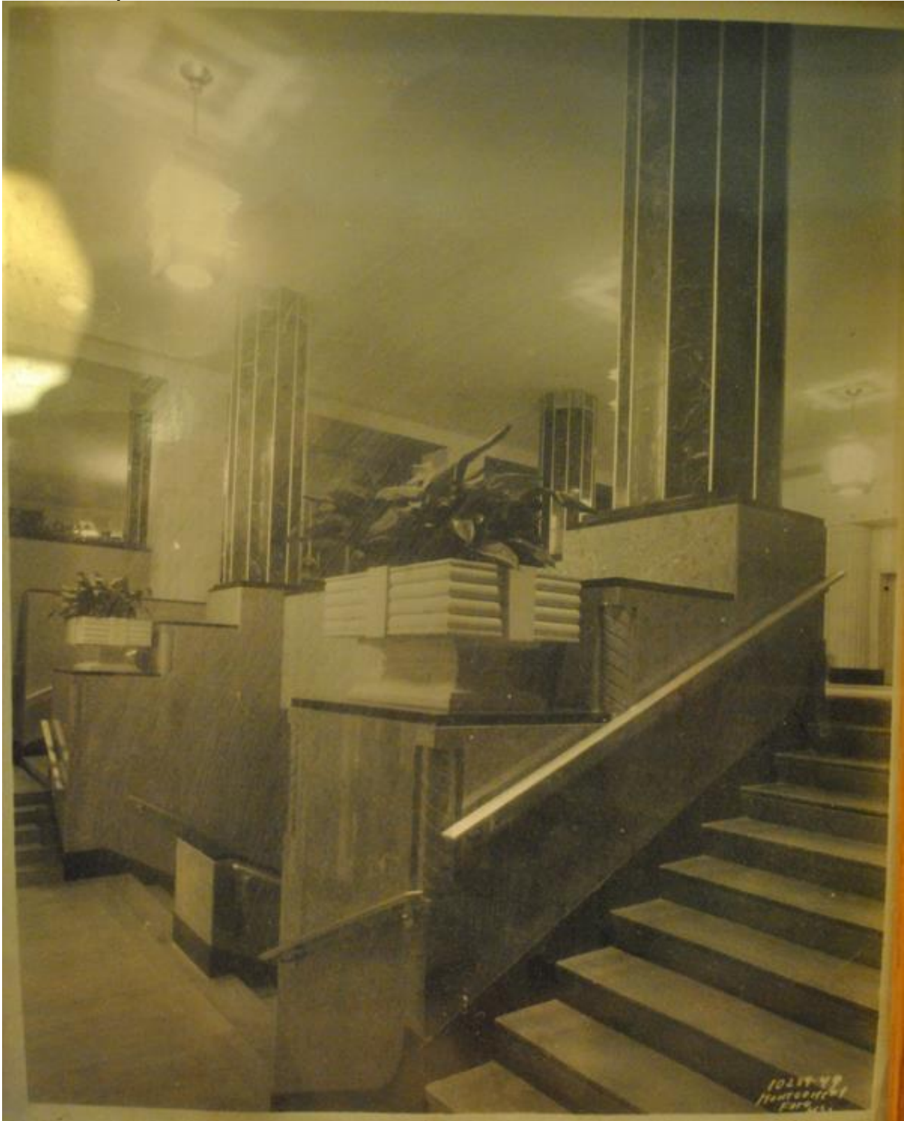
Figure 7. Lobby at State Avenue entrance, c. 1951. Photo courtesy of Cross-Line Towers, Inc.
